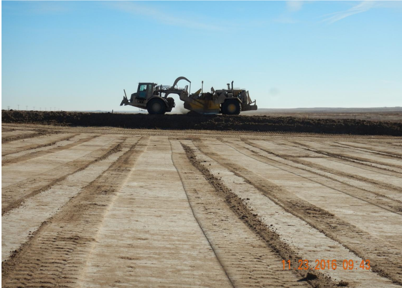
Photo 3. Photo taken from approximate center of location, facing East, towards the topsoil stockpile. Topsoil salvage IN-PROCESS.
