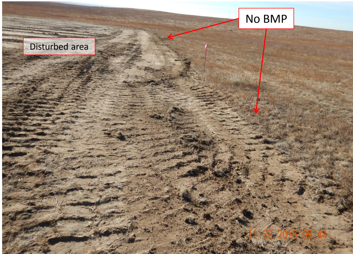
Photo 4. Photo taken from the western location, facing South. No BMPs. Stormwater and erosion control BMPs need to be installed prior to the start of construction.
