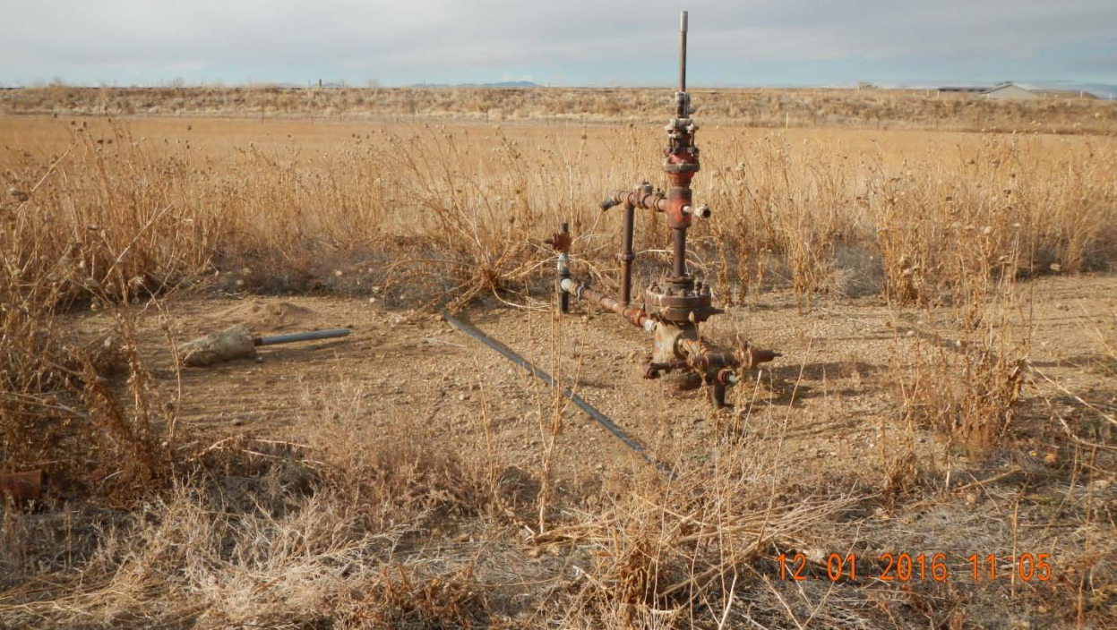
API # 123-10103, unused equipment at well.
