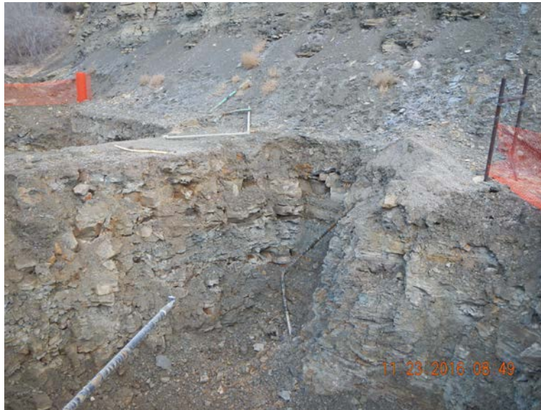
Excavation into weathered bedrock looking north
