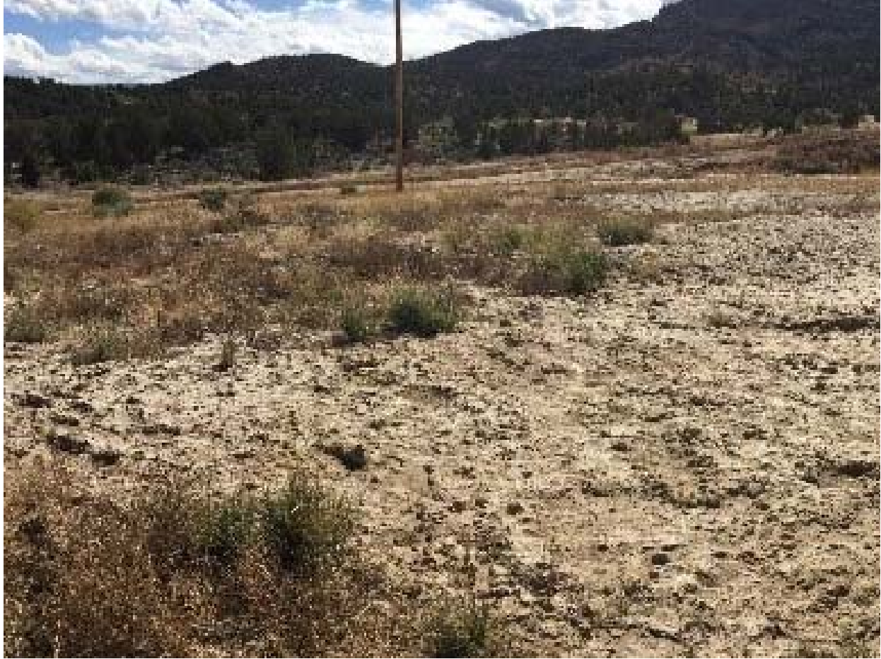
GREENLEAF DISPOSAL 1 PAD, NESW, SECTION 36, T 9 S, R 97 W, MESA COUNTY OVERALL WELL PAD VIEW LOOKING NORTHERLY
