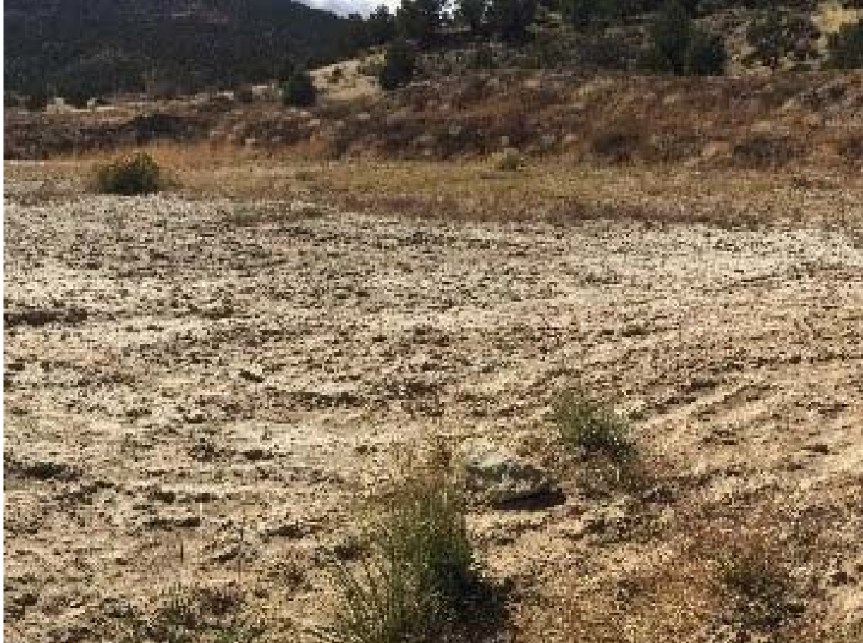
GREENLEAF DISPOSAL 1 PAD, NESW, SECTION 36, T 9 S, R 97 W, MESA COUNTY WELL PAD ACCESS ROAD VIEW LOOKING NORTHEASTERLY
