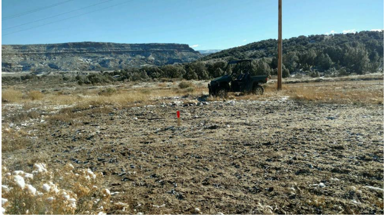
GREENLEAF DISPOSAL 1 PAD, NESW, SECTION 36, T 9 S, R 97 W, MESA COUNTY WELL PAD LOOKING EAST
