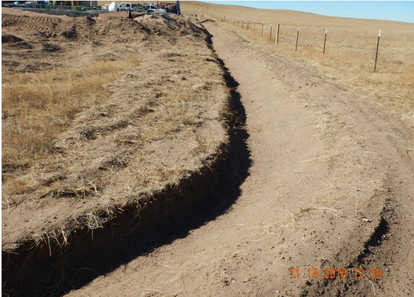
Photo 5. Photo taken from the northeast location , facing West. Ditch and berm BMP installed around the location perimeter. Ditch should be constructed with a 2:1 slope on both sides.
