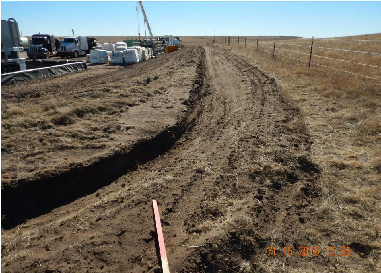
Photo 6. Photo taken from the northwest location , facing South. Ditch and berm BMP installed around the location perimeter. Ditch should be constructed with a 2:1 slope on both sides.
