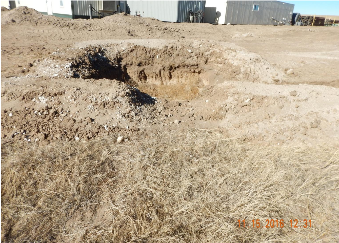
Photo 2. Photo taken from the southeastern location, facing West, towards the sediment trap. Sediment trap side slopes should not be steeper than 2:1 and the outlet should be stabilized (e.g., geotextile with rip rap on top).
