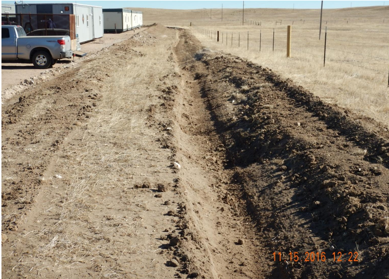
Photo 1. Photo taken from the southern location , facing East. Ditch and berm BMP installed around the location perimeter.
