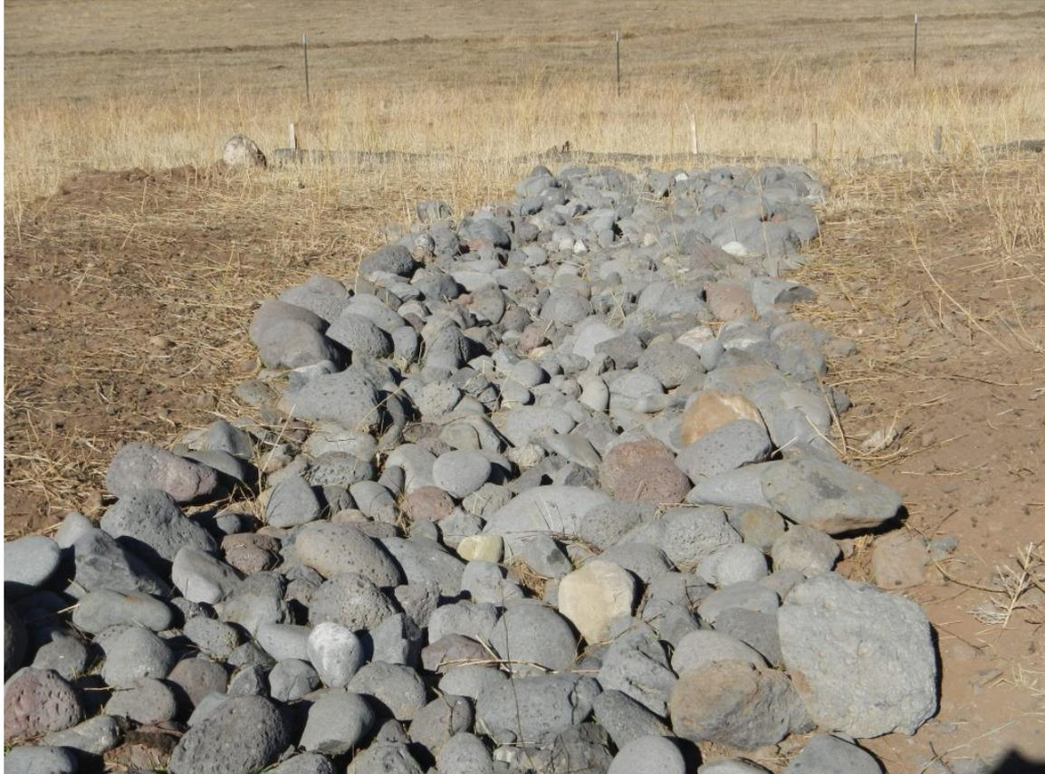
Photo#3: Rock Drain and Wattles at east end of Location
