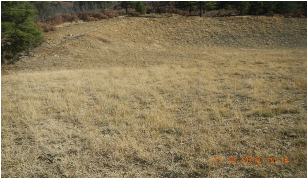
photo 8: Facing east toward the cut slope side of the location.
