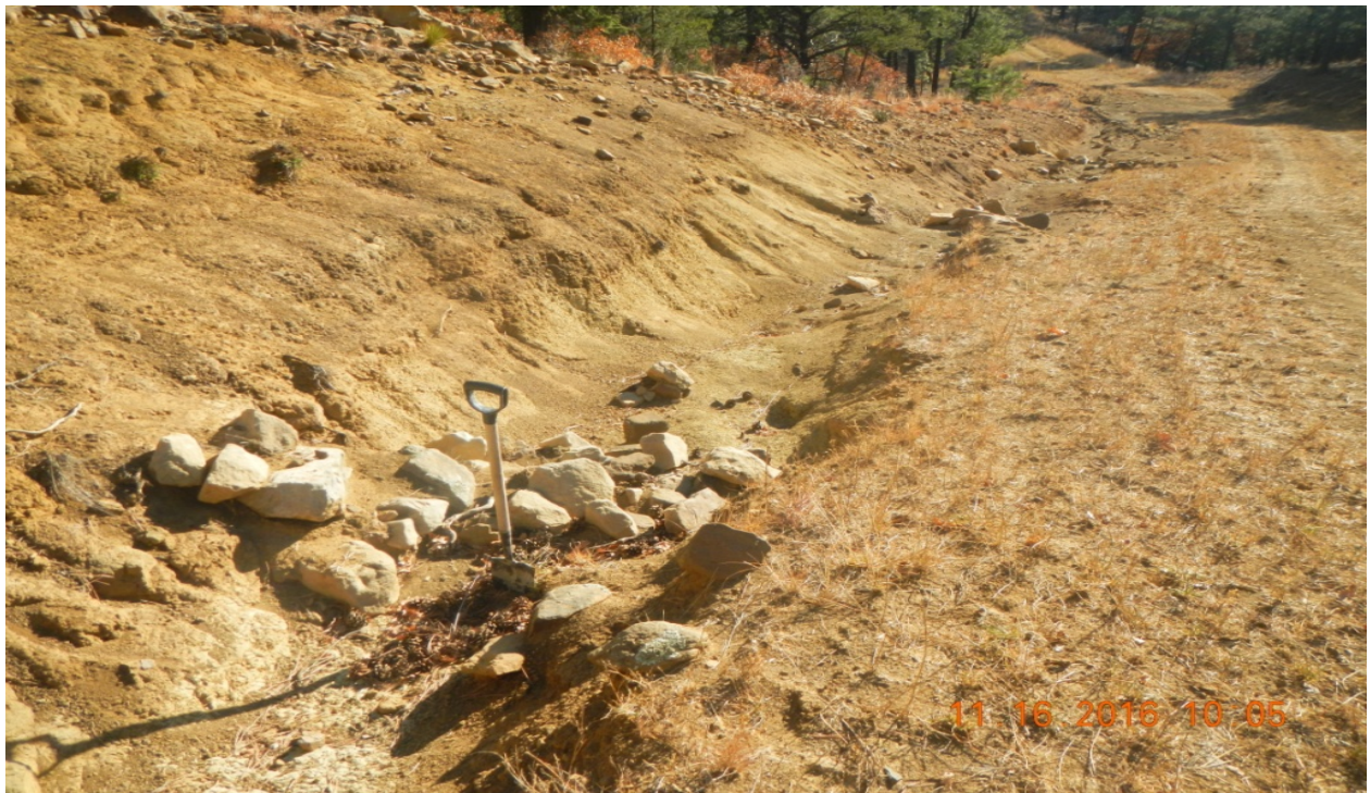
photo 6: The rock check dams are not maintained and erosion is occurring along the road side.
