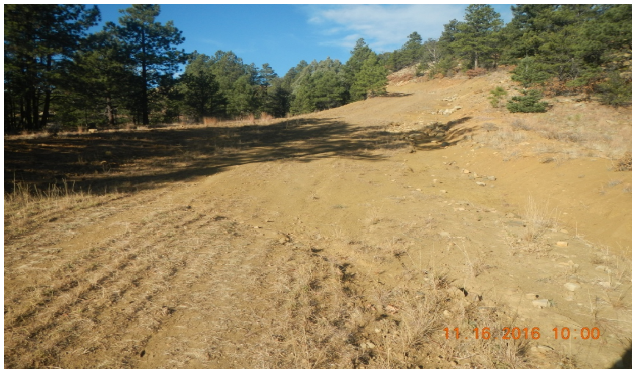
photo 3: Facing west along the access road.
