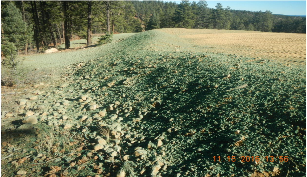
photo 3: North side of the location which was being hydro-mulched.
