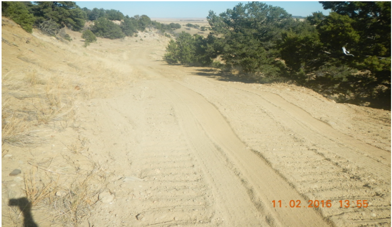
photo 3: Facing northeast along the access road.
