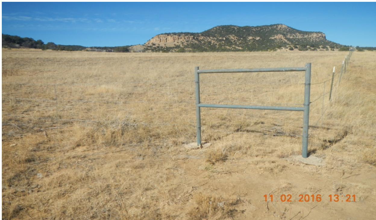
photo 5: Southeast side of the location facing northwest.
