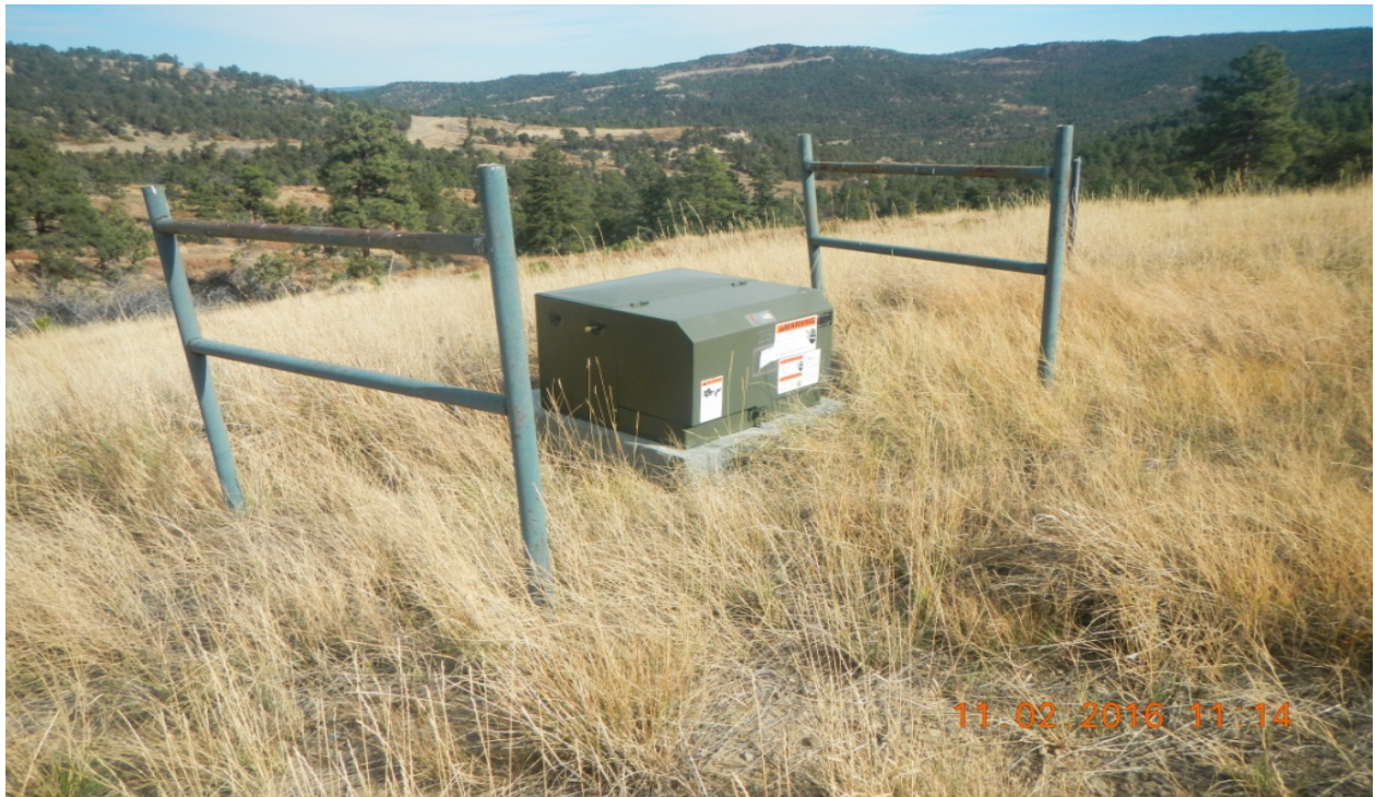
photo 5: An electric utility remains at the location.
