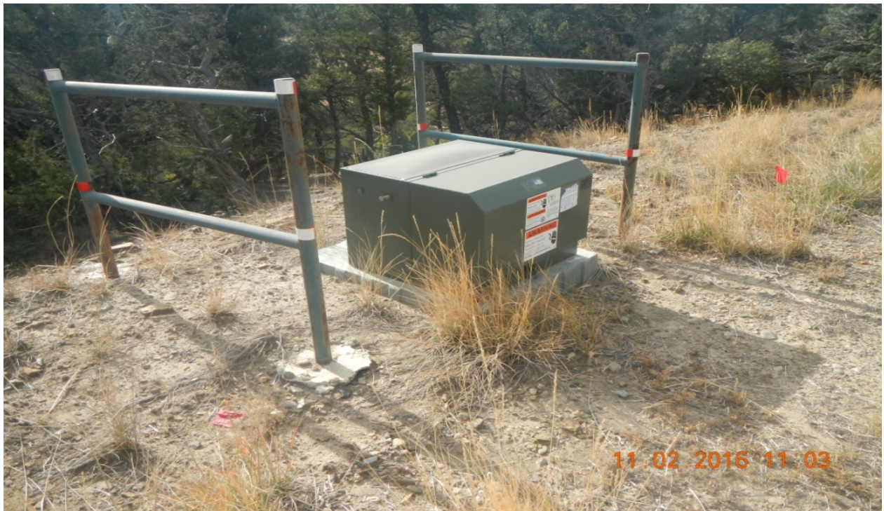
photo 4: An electric utility remains along the access road.
