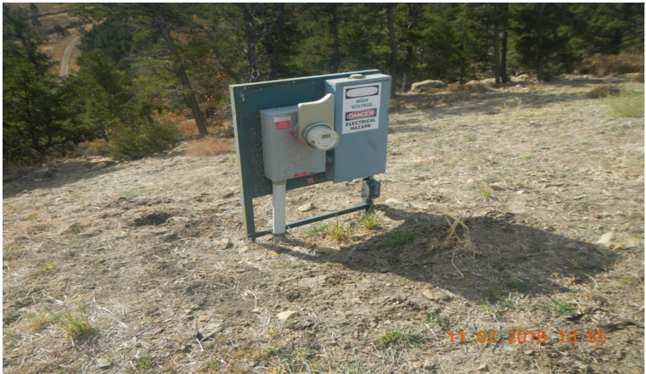
photo 8: An electric utility remains at the location.
