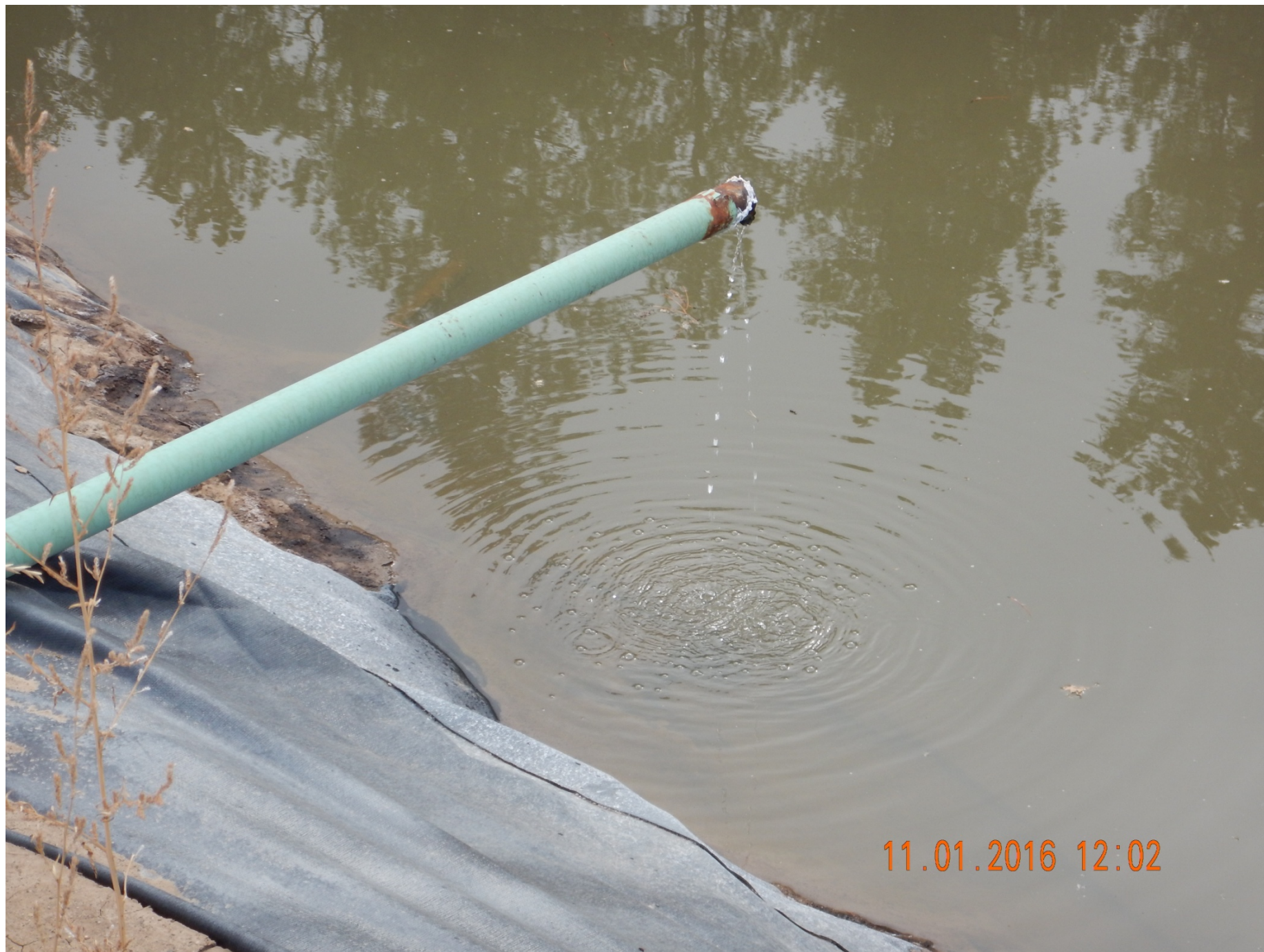
Samples obtained directly from produced water line feeding lined pit.
