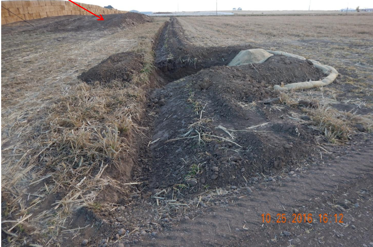
Photo 1. Photo taken from northwestern corner of perimeter, facing South, south of the access road. Stabilized sediment trap installed. Topsoil pile stored along western location. Ditch and berm constructed around outer perimeter of the location.
