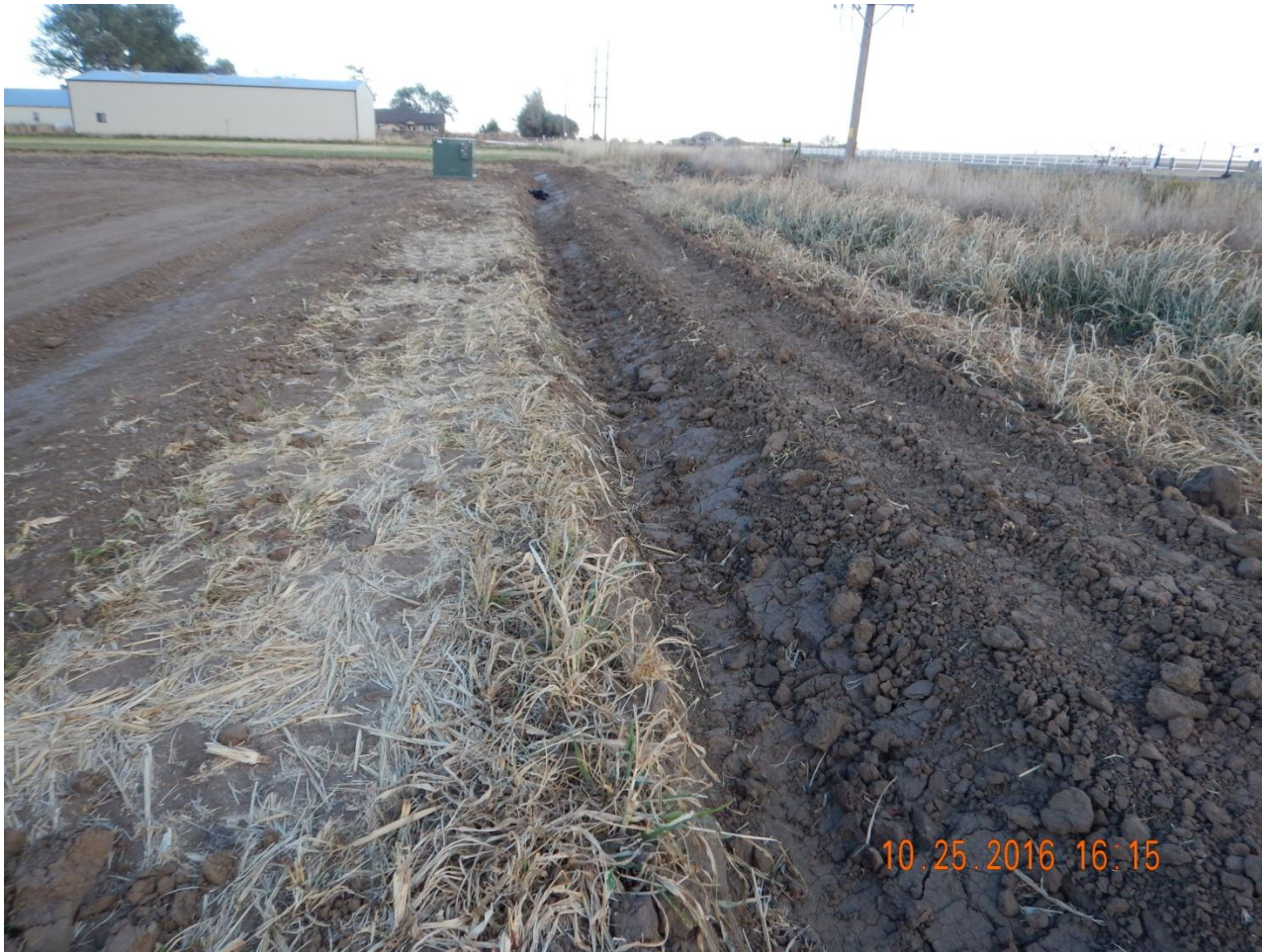
Photo 4. Photo taken from southern perimeter of the location, facing East. Ditch and berm constructed around outer perimeter of the location.
