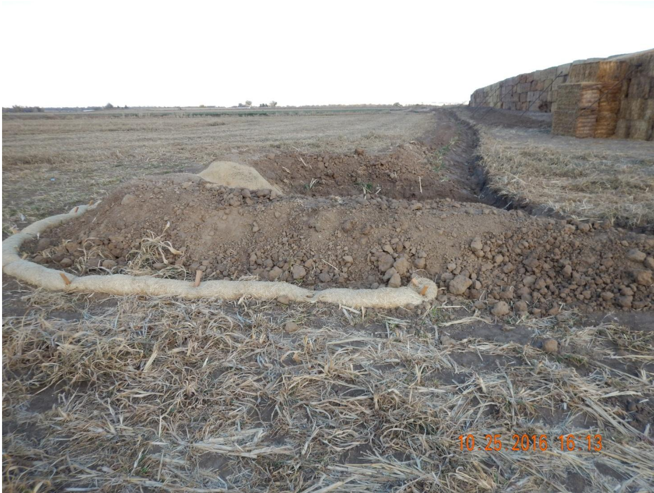
Photo 2. Photo taken from northwest corner of perimeter, facing East, north of the access road. Stabilized sediment trap installed. Ditch and berm constructed around outer perimeter of the location.
