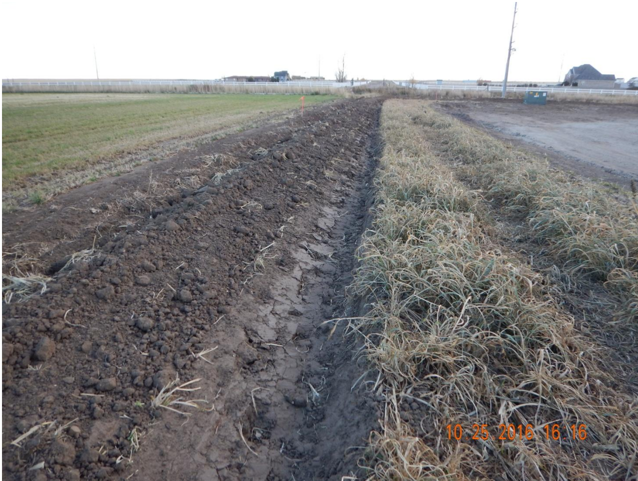
Photo 5. Photo taken from eastern perimeter of the location, facing South. Ditch and berm constructed around outer perimeter of the location.
