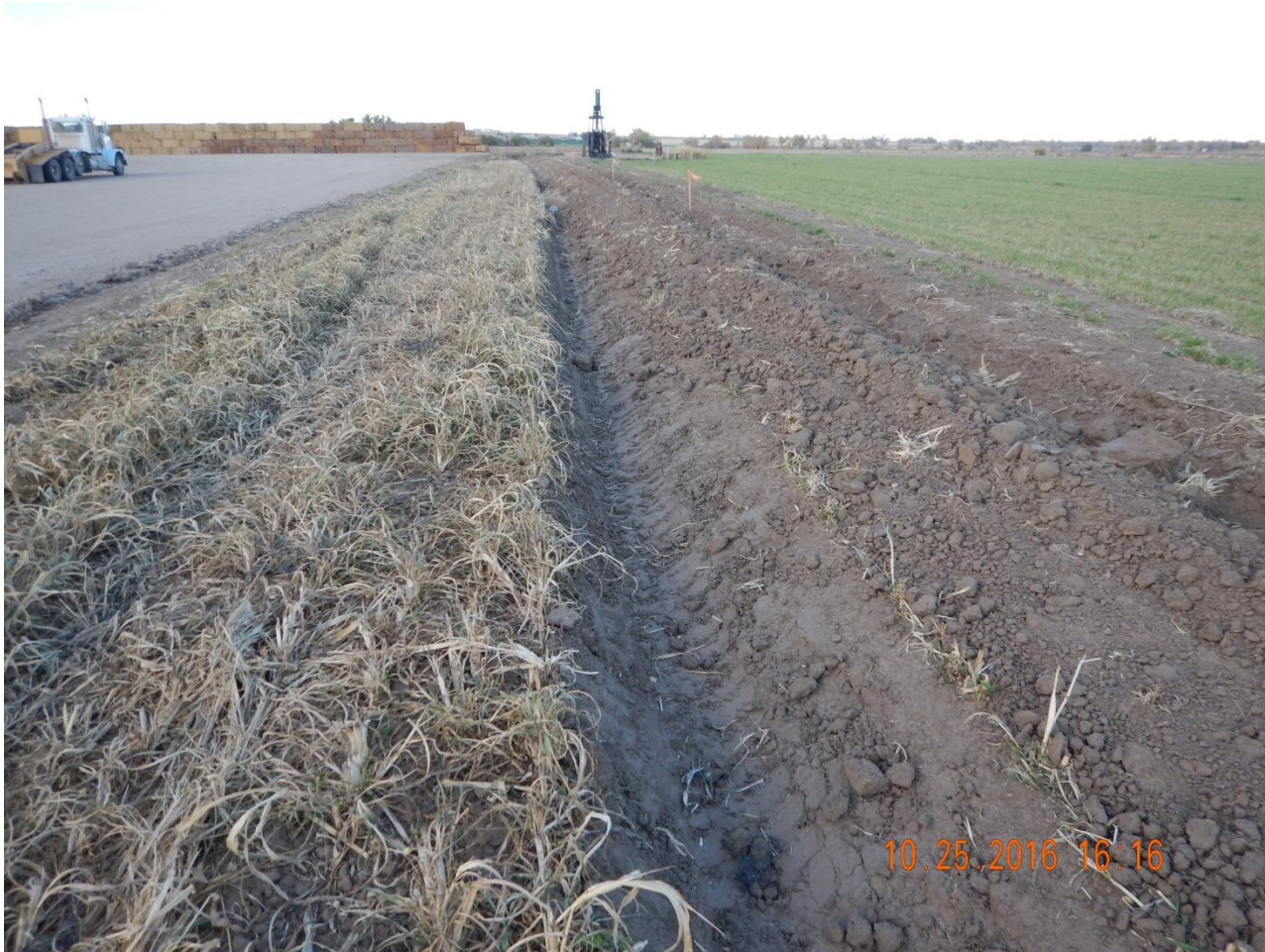
Photo 6. Photo taken from eastern perimeter of the location, facing North. Ditch and berm constructed around outer perimeter of the location.
