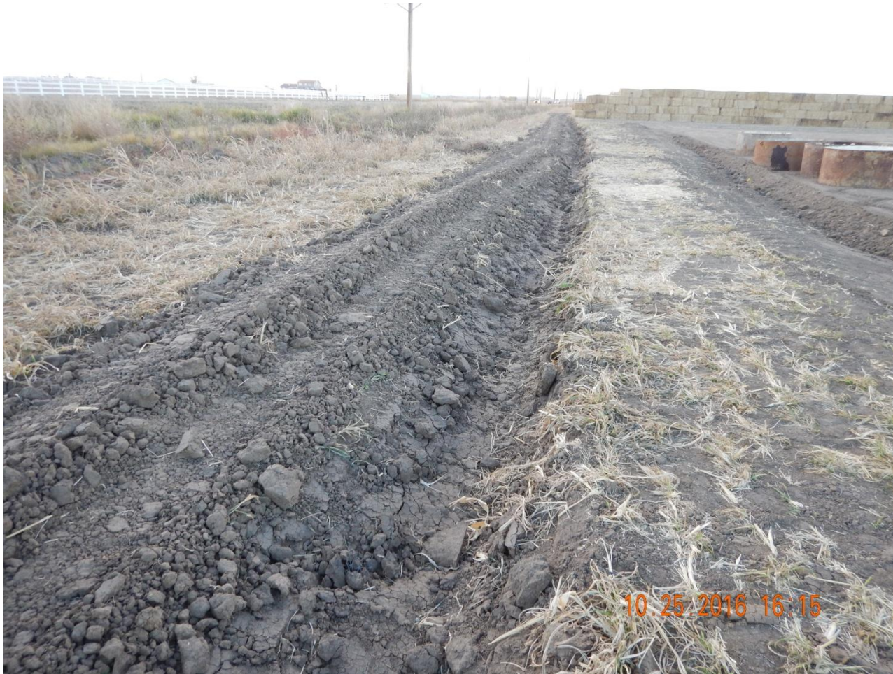
Photo 3. Photo taken from southern perimeter of the location, facing West. Ditch and berm constructed around outer perimeter of the location.
