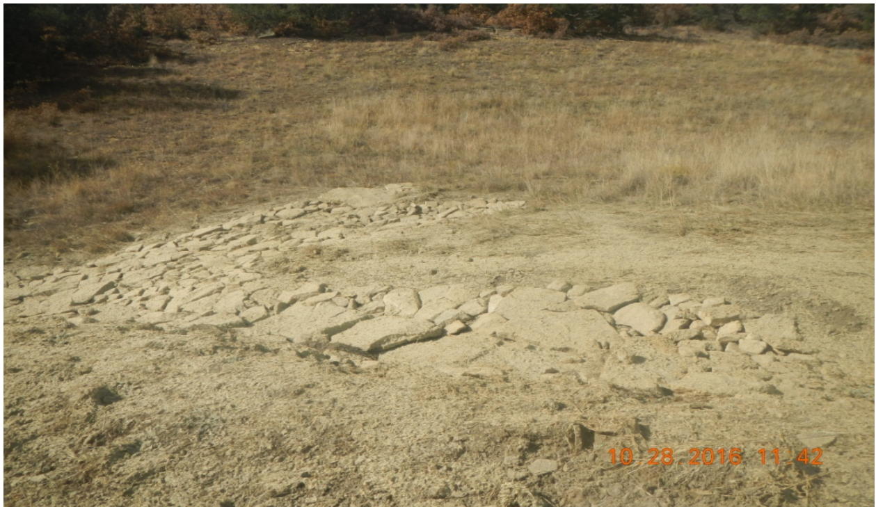
photo 8: South side of the location facing west. Rip/rap rock has been placed in this area for stormwater control.
