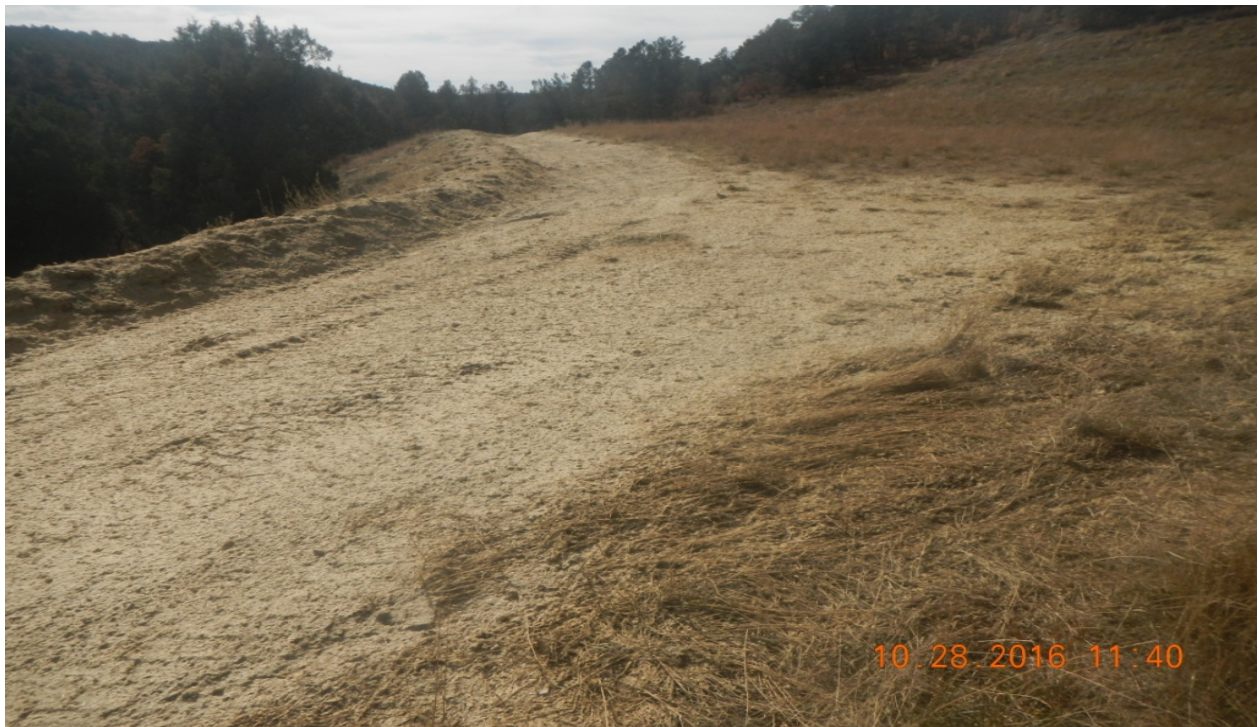
photo 6: Facing south toward the location. The east side has been seeded and hydromulched.
