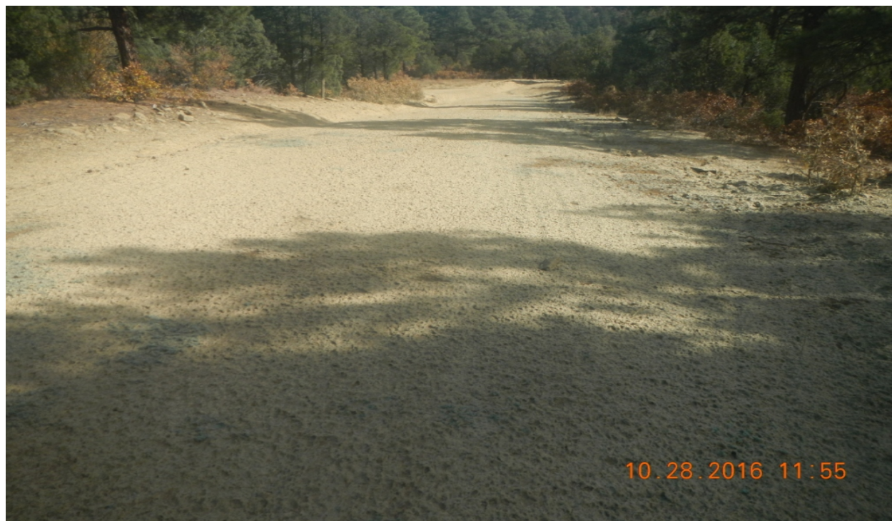
photo 1: Facing east along the access road near the Wriggly Red 44-21 location. This portion of pre-existing road had recently been seeded and hydromulched.
