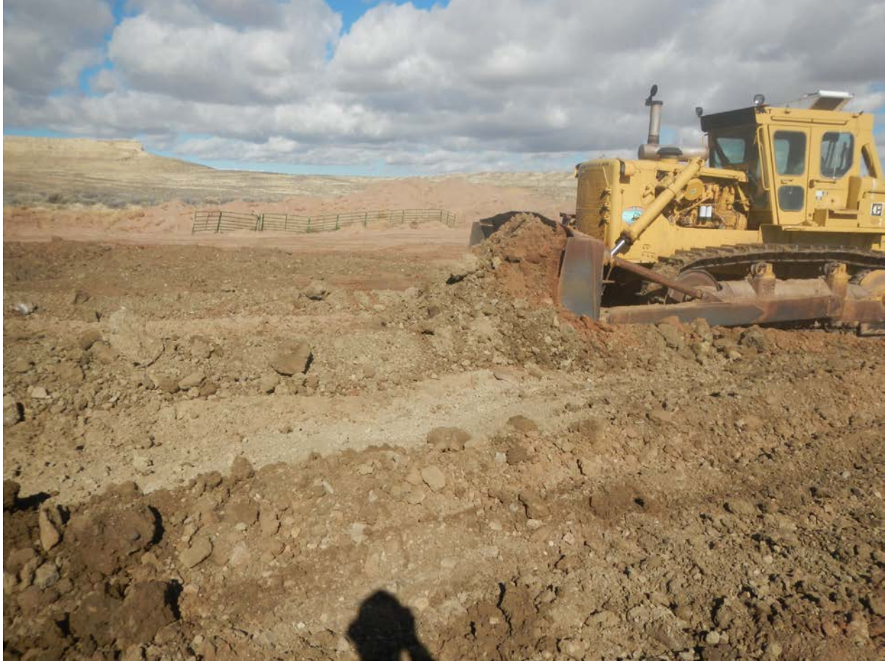
Material spread on location to assess if it has been contaminated with any foreign material.
