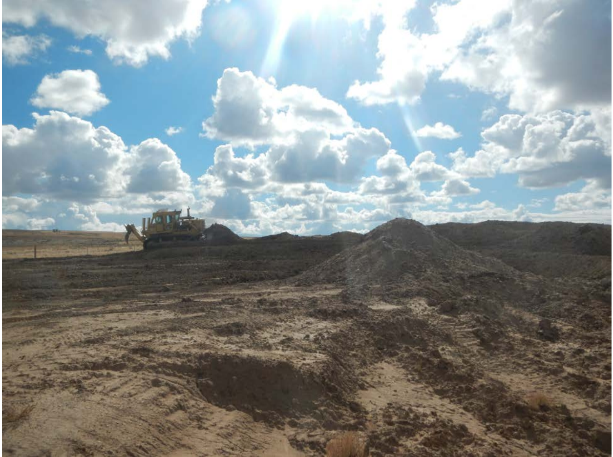
Soil pile in the foreground, is contaminated material that needs to be hauled off to offsite disposal
