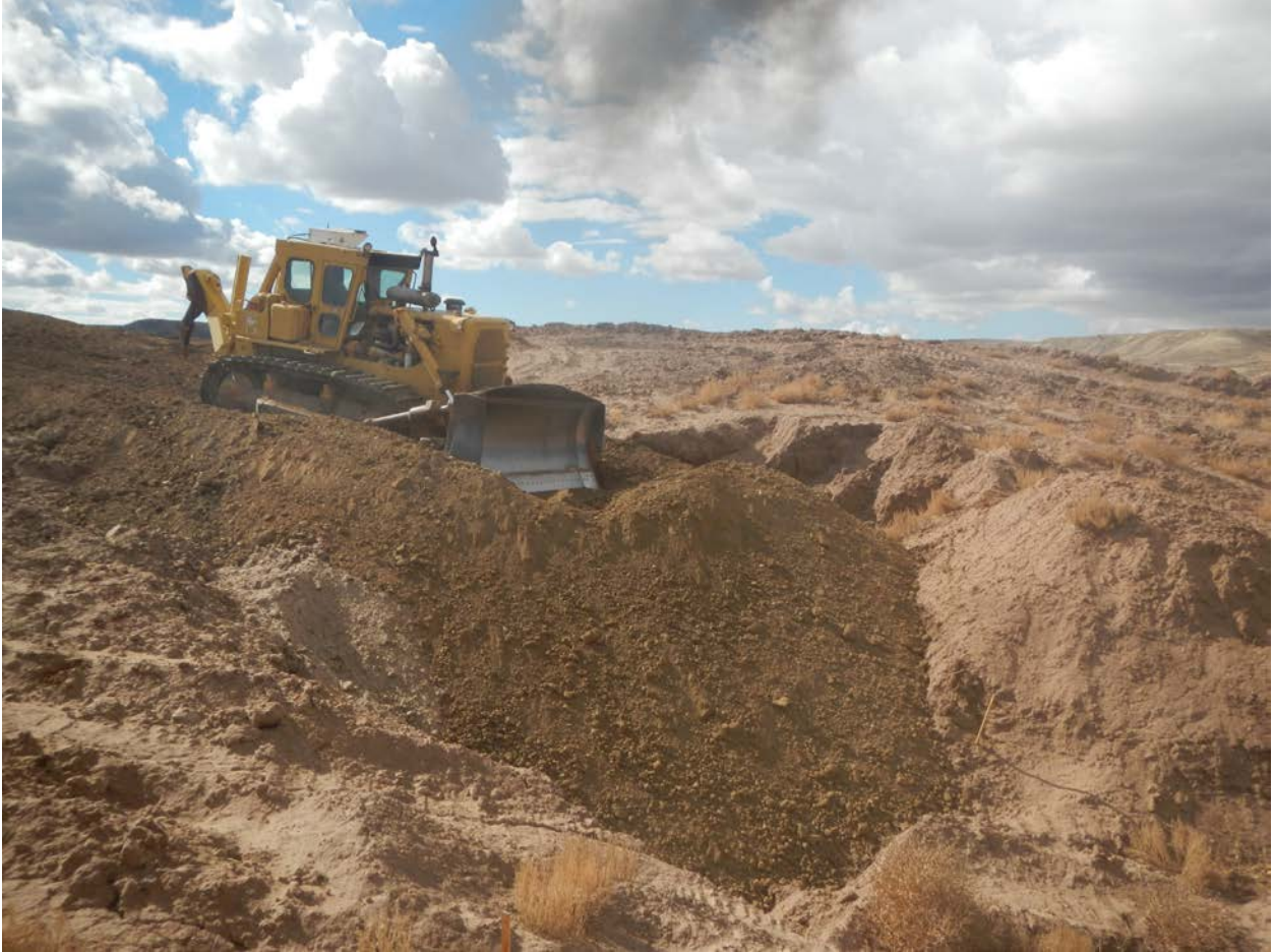
Pushing fill material into pit.
