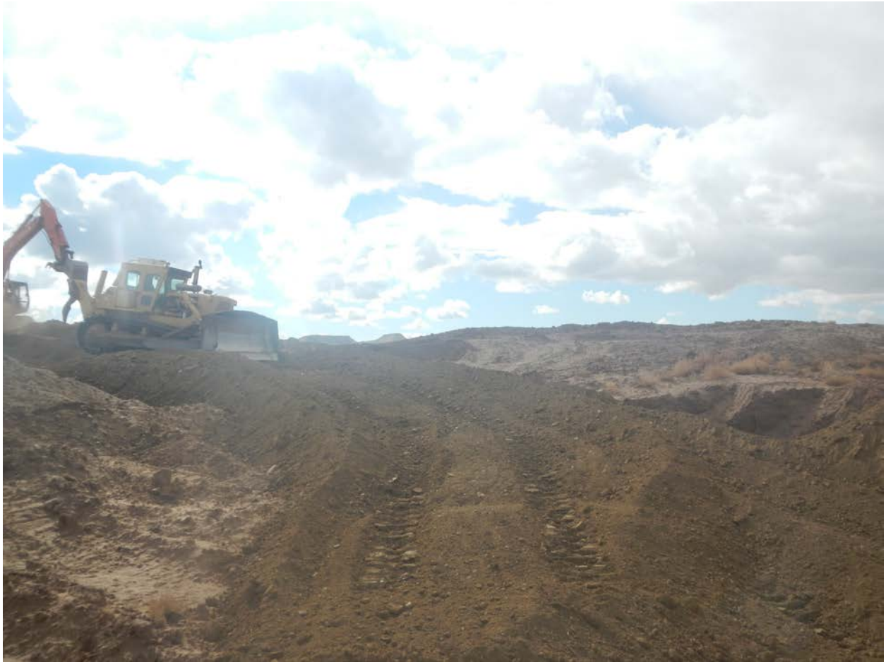
Crews working the fill material into pit excavation.
