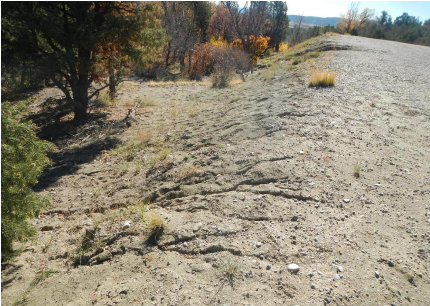
Photo 4. View of the eastern portion of the project area from the northeastern corner facing southward. Rill and gully erosion is still occurring and stormwater controls are not sufficient.
