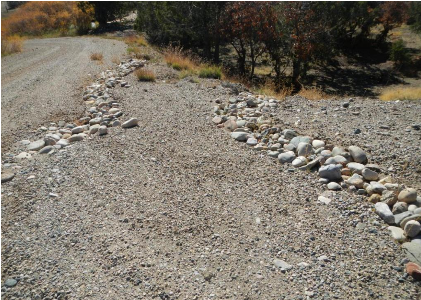
Photo 1. View of cobble run-downs and gravel at the entrance to the well pad. These appear to be functioning at this time.
