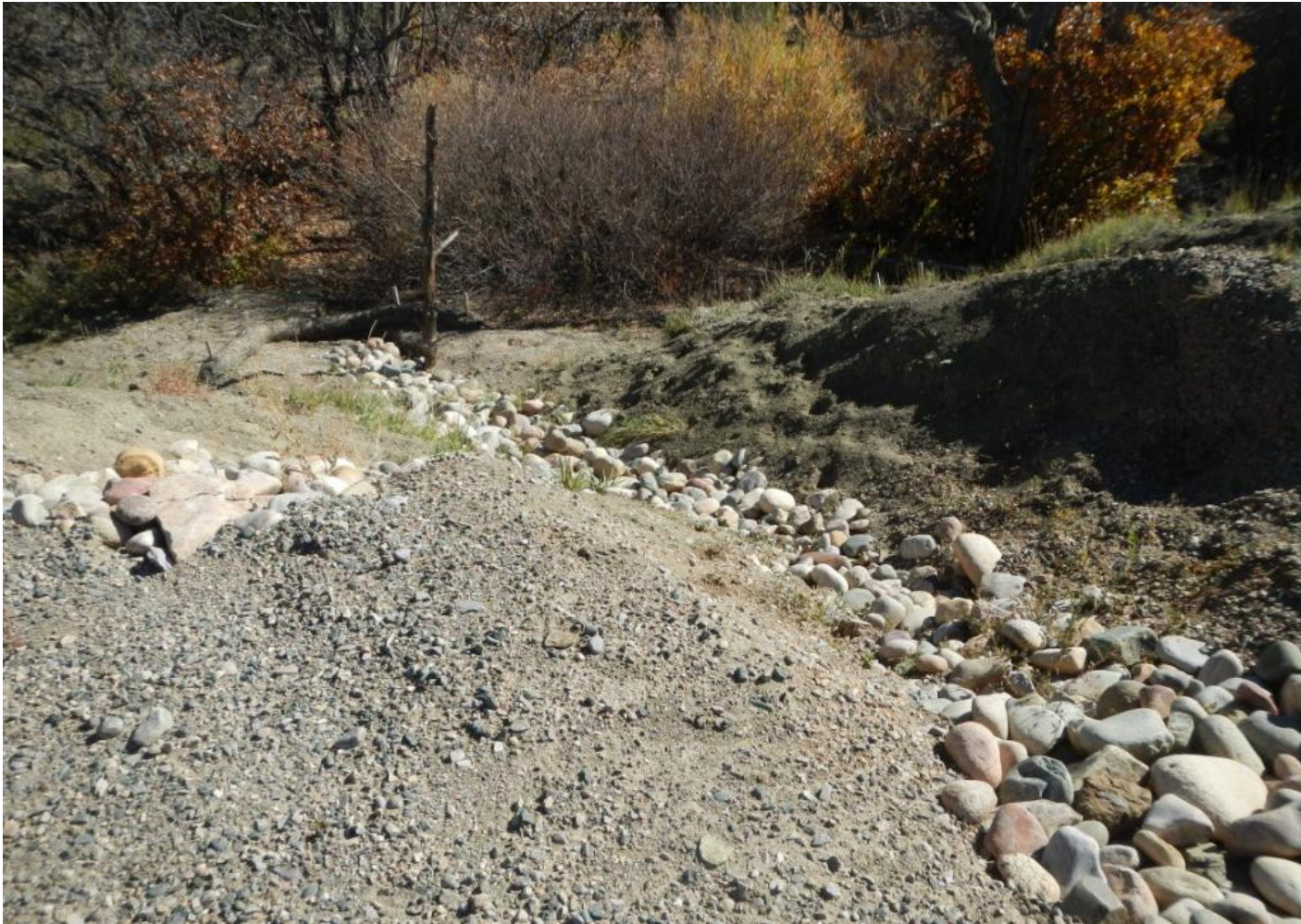
Photo 5. View of cobble run down in the eastern portion of the project area. Wattles at bottom of the slope need maintenance.
