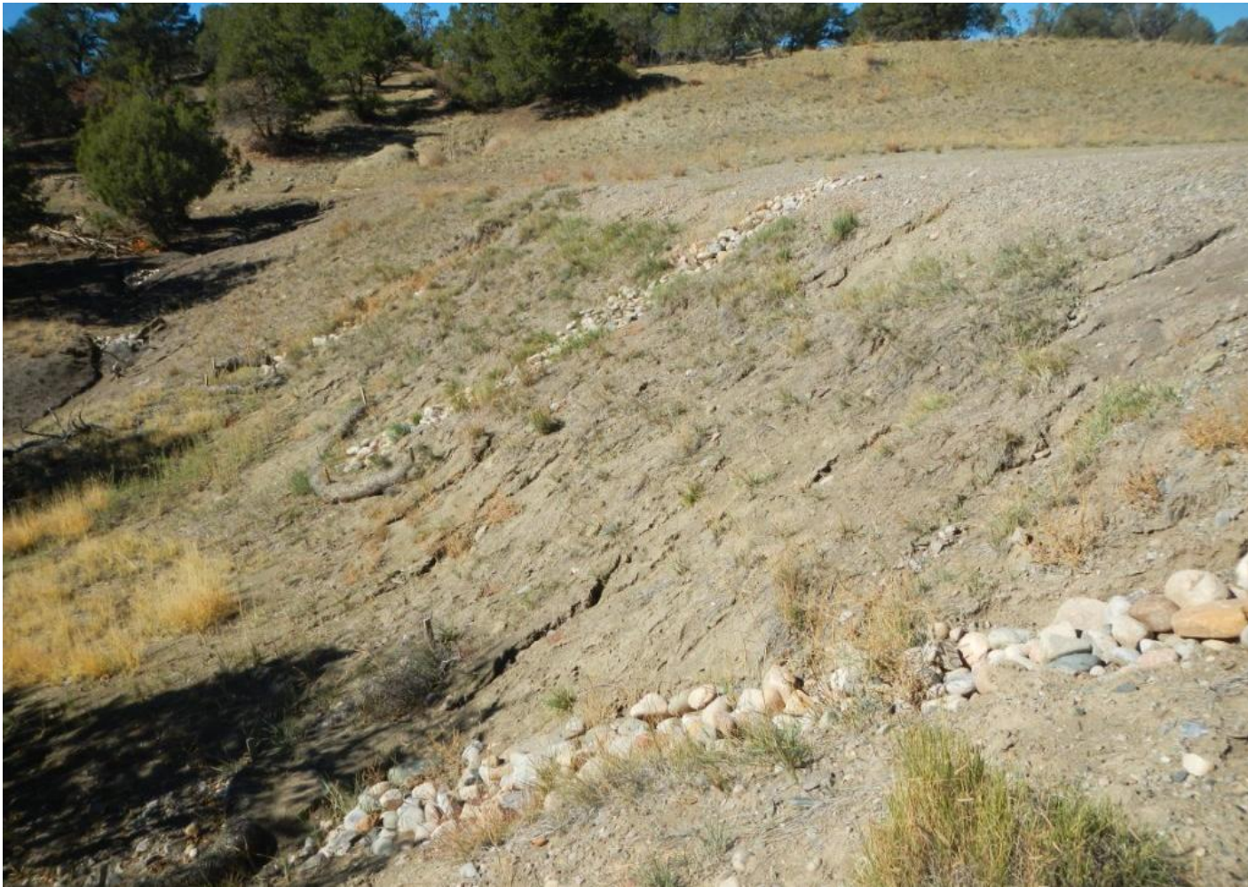
Photo 2. View of the southern portion of the project area from the well pad entrance facing westward. In some areas stormwater controls are functioning in other areas stormwater controls need maintenance (photo 6), and in other areas there are no controls and additional controls are needed. Rills and gullying are still present in the southern fill slope.
