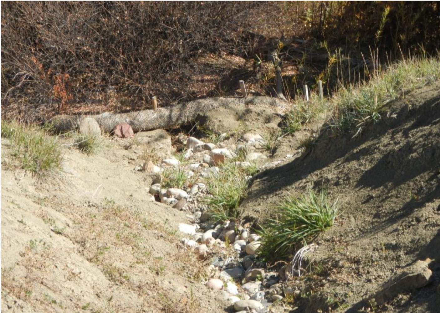
Photo 6. Closeup of straw wattles at bottom of eastern fill slope where sediment is accumulated and stormwater flows beneath the wattle. An irrigation ditch is just beyond the wattle.
