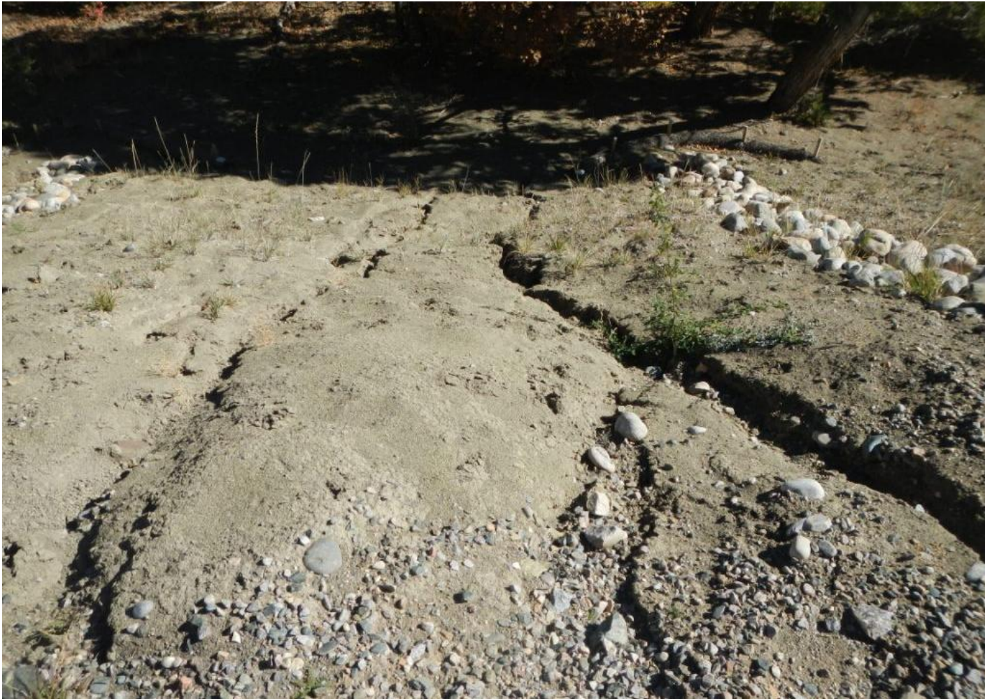
Photo 7. Another view of rills in the eastern portion of the project area that do not have sufficient stormwater controls.
