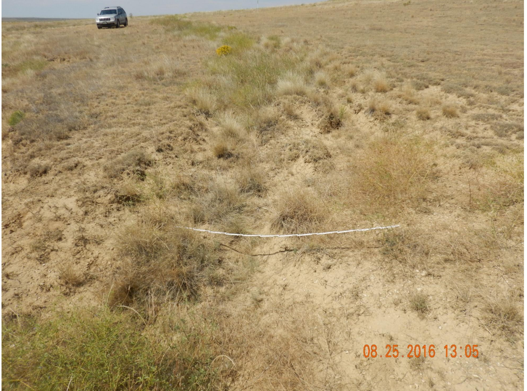
Figure 12: Photo taken from the northeast corner of the location, facing northwest. Photo shows areas of the access road experiencing erosion. 6' measuring stick for reference.
