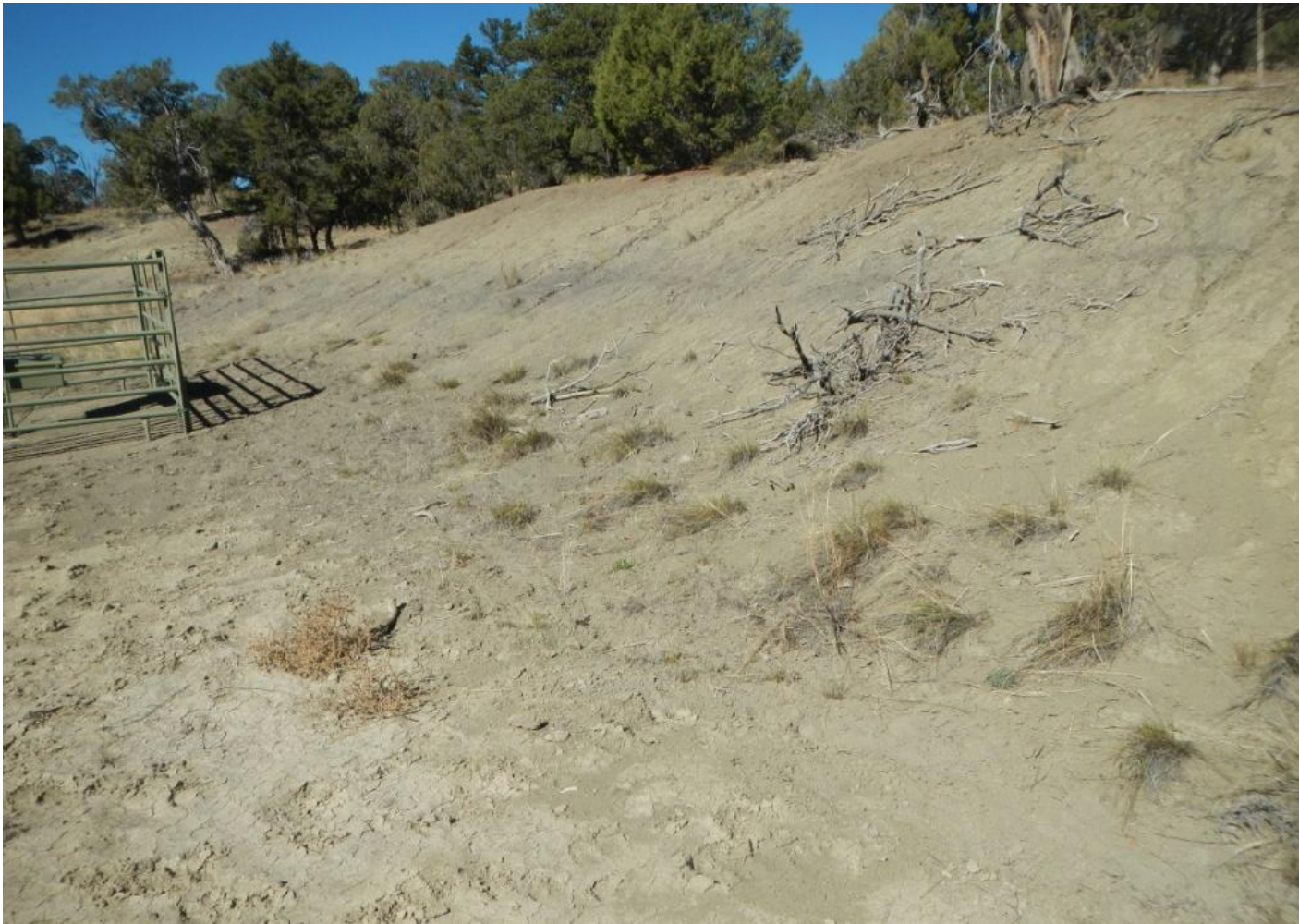
Photo 3. View of northern cut-slope with sparse revegetation.
