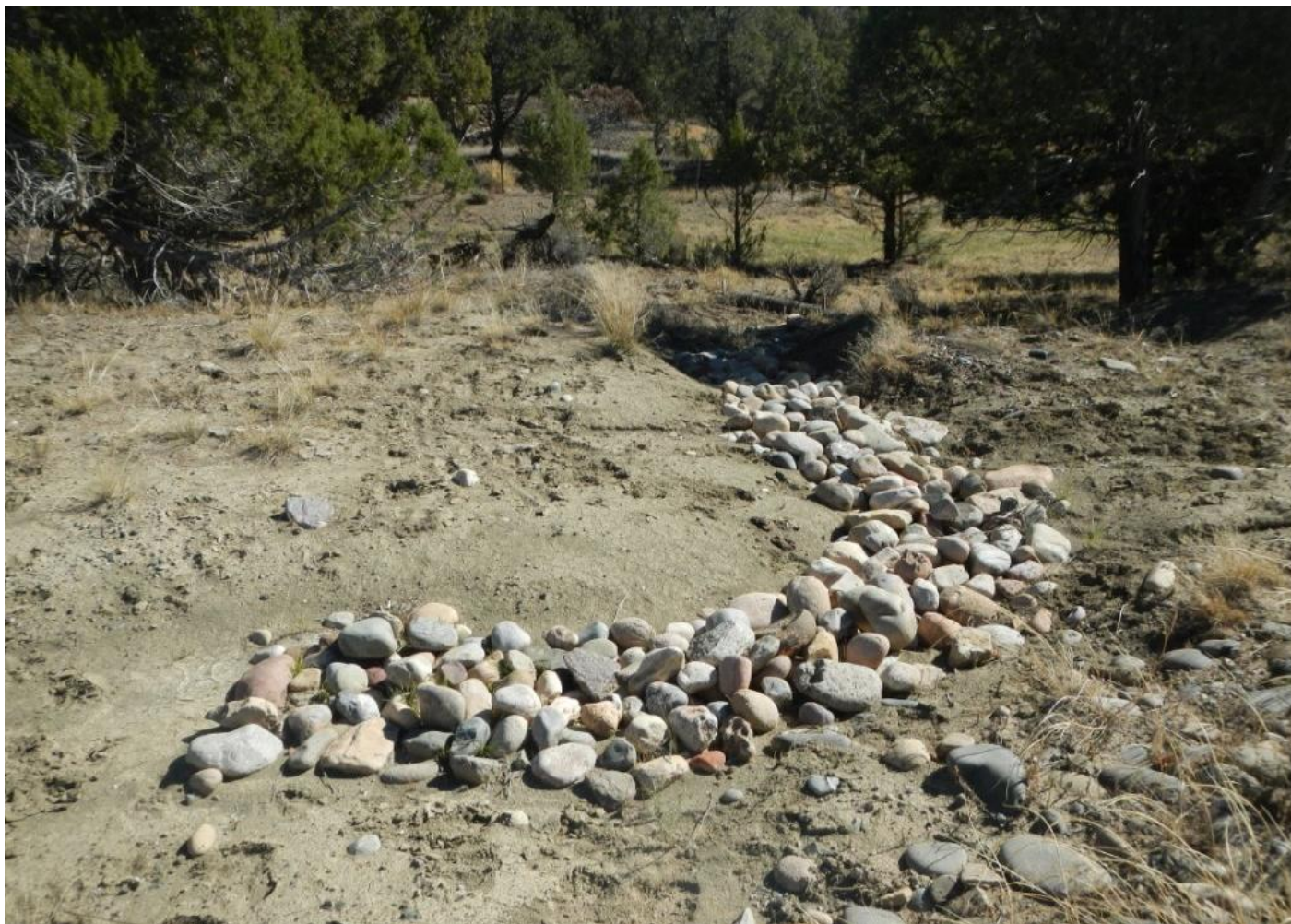
Photo 4. View of cobble run-down placed to stabilize erosional channel in the northeastern portion of the project area.
