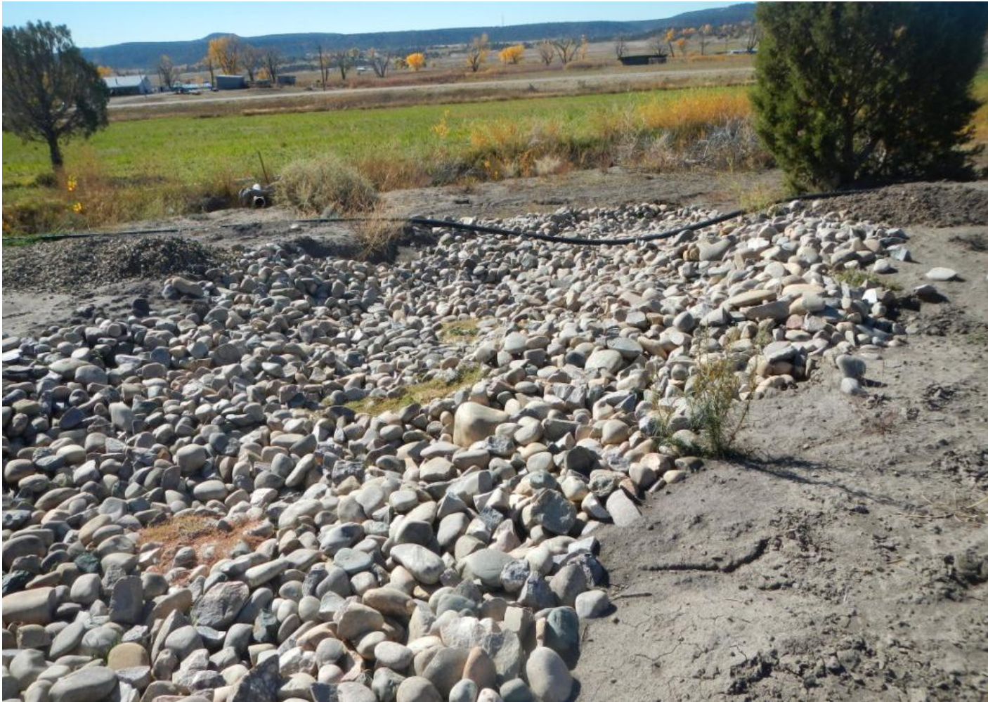
Photo 4. View cobble run-down in the southwestern corner of the project area, appears to be functioning.
