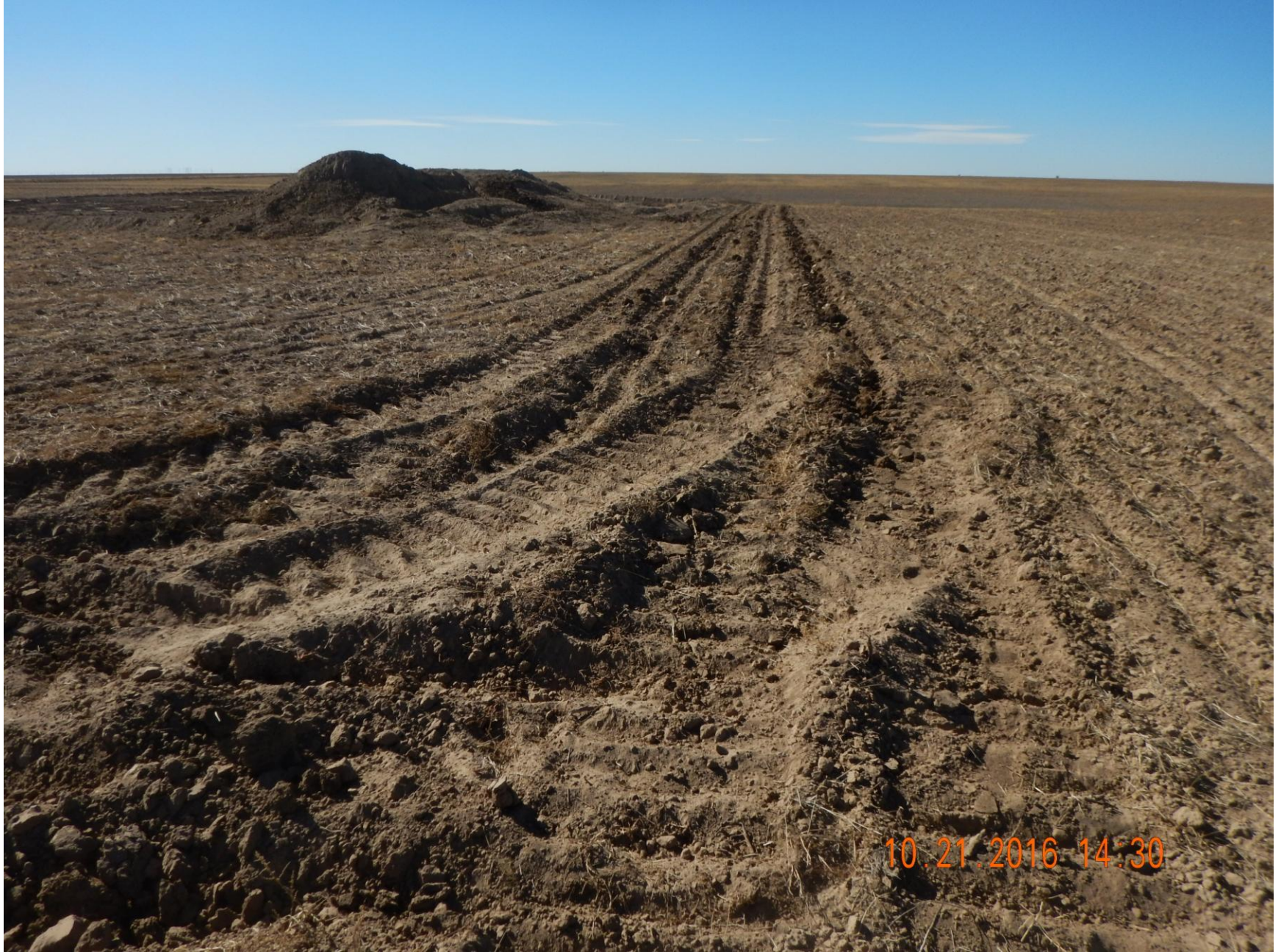
Figure 11: Photo taken from the northeast corner of the location, facing west. Photo shows surface roughening implemented around perimeter of location. Topsoil stockpile to the top right of the photo.
