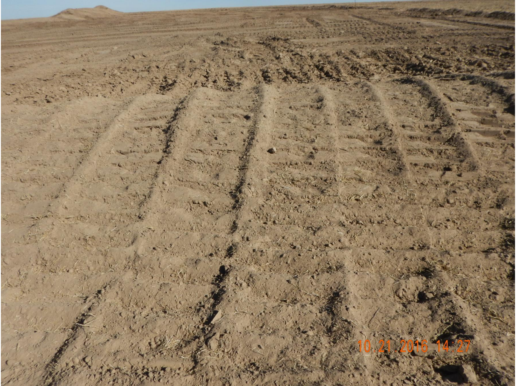
Figure 8: Photo taken from the west end of the location, facing north. Photo shows berms along the western and northern perimeter of the location have been adequately tracked.
