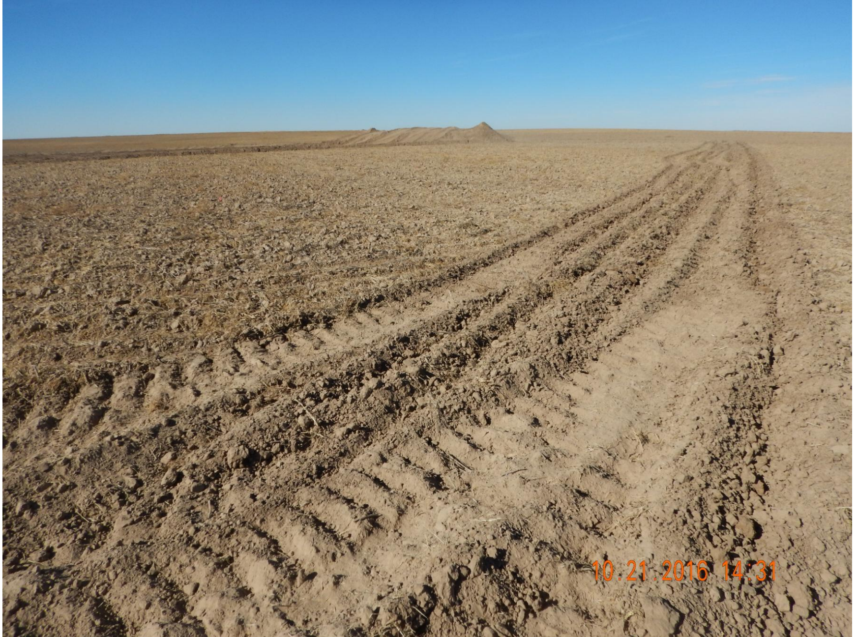
Figure 14: Photo taken from the southeast corner of the location, facing north. Photo shows surface roughening implemented around perimeter of location
