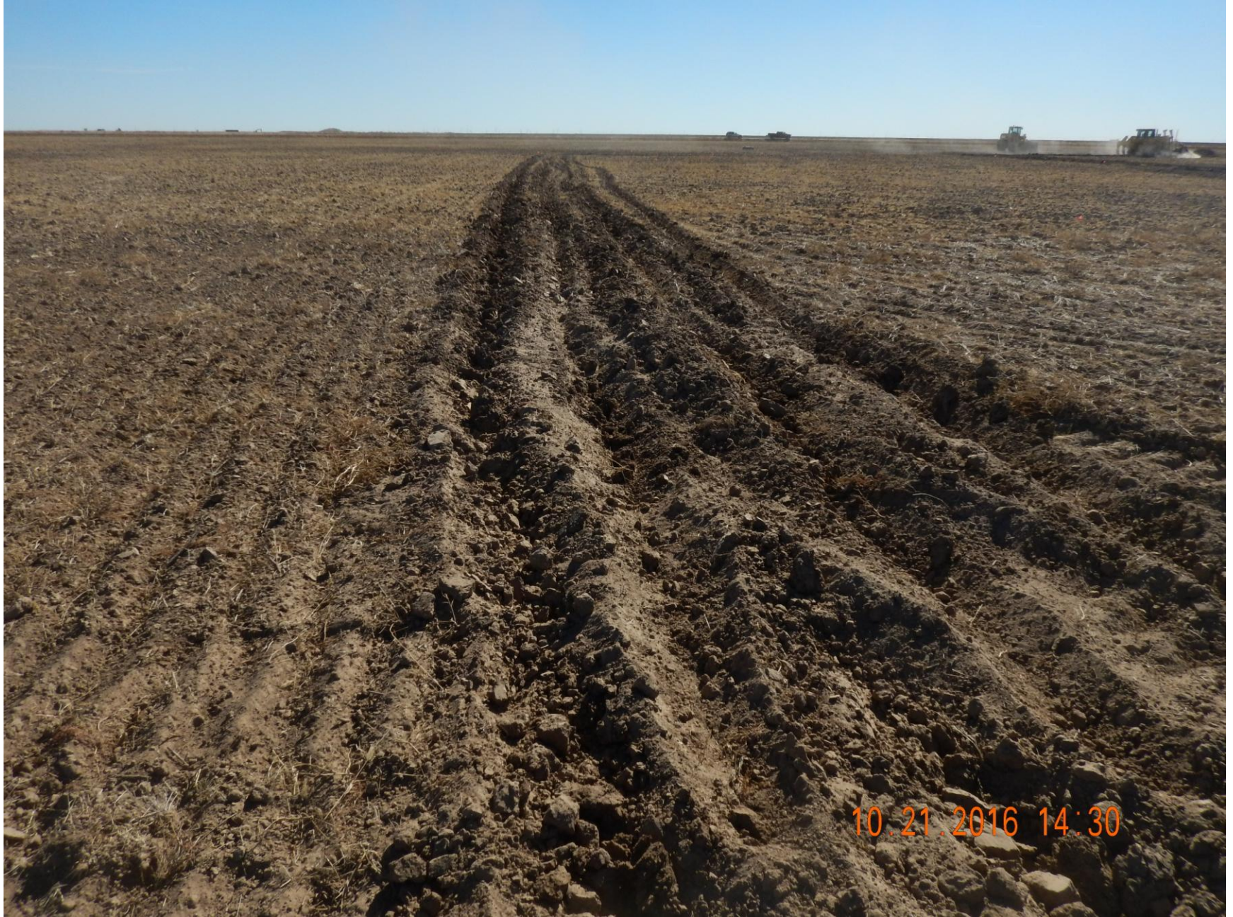
Figure 12: Photo taken from the northeast corner of the location, facing south. Photo shows surface roughening implemented around perimeter of location.
