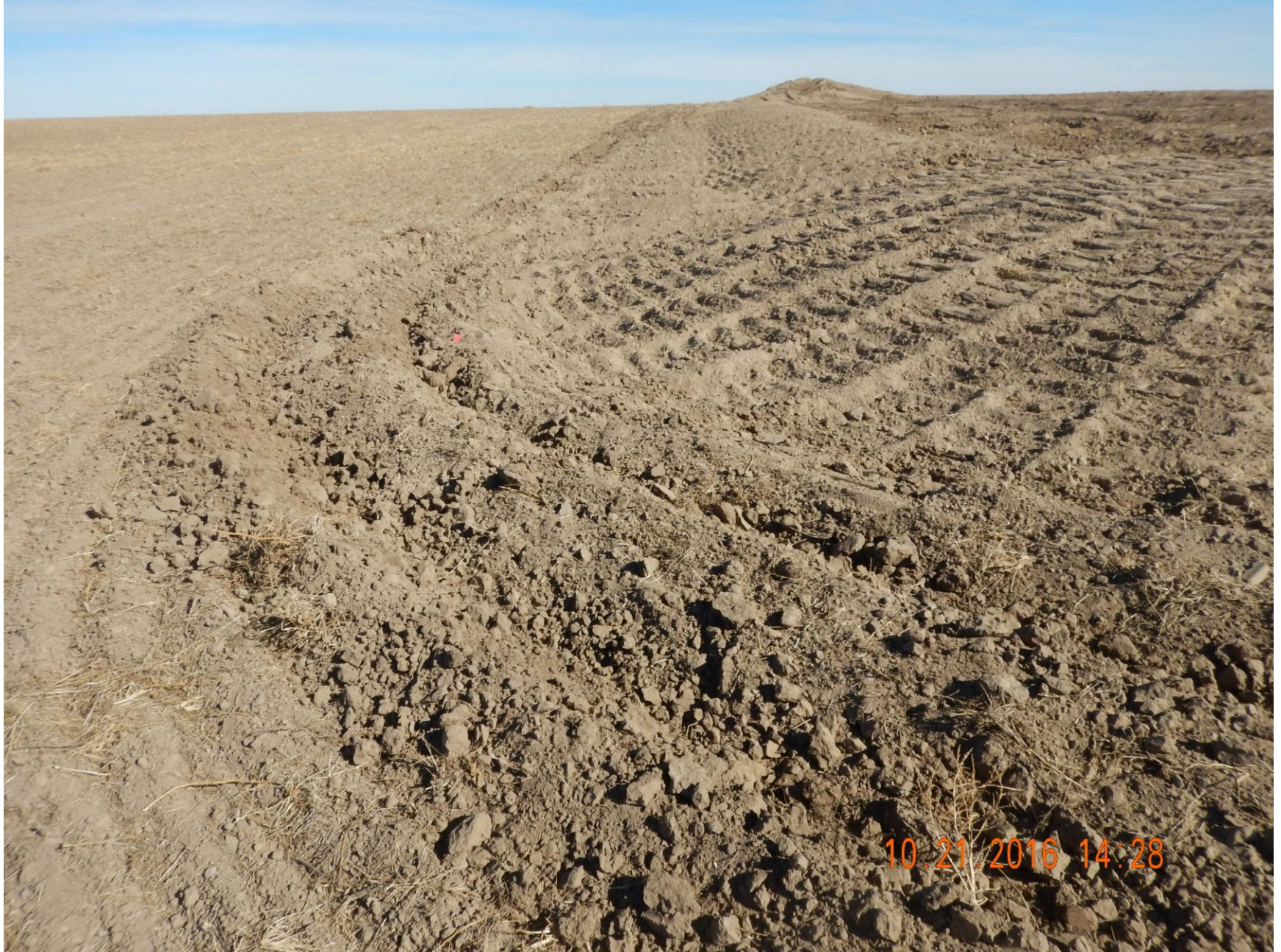
Figure 10: Photo taken from the northwest corner of the location, facing east. Photo shows surface roughening used in conjunction with berms as a stormwater and sediment control BMP.
