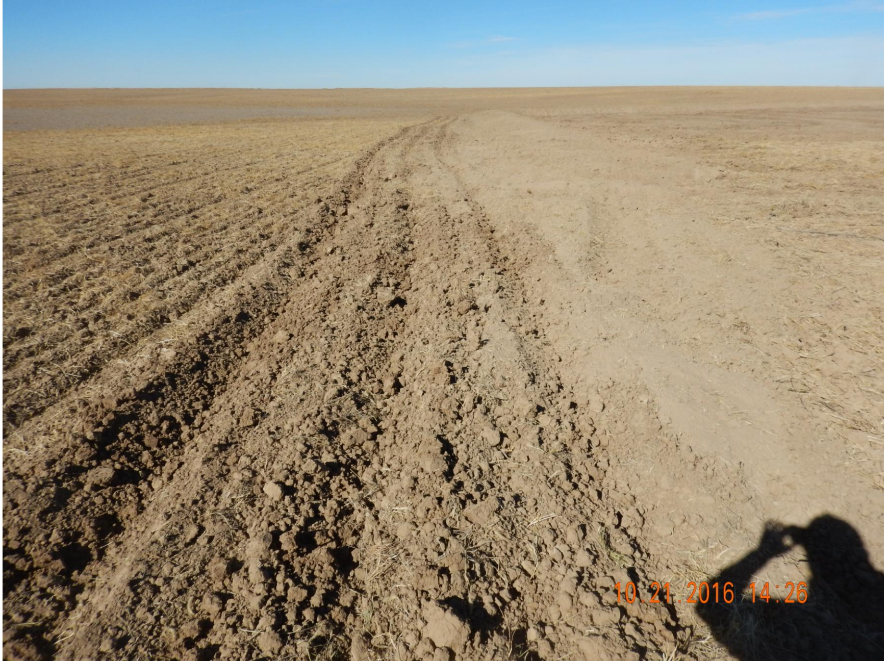
Figure 7: Photo taken from the west end of the location, facing north. Photo shows surface roughening has been constructed in conjunction with berms as a stormwater and sediment control BMP
