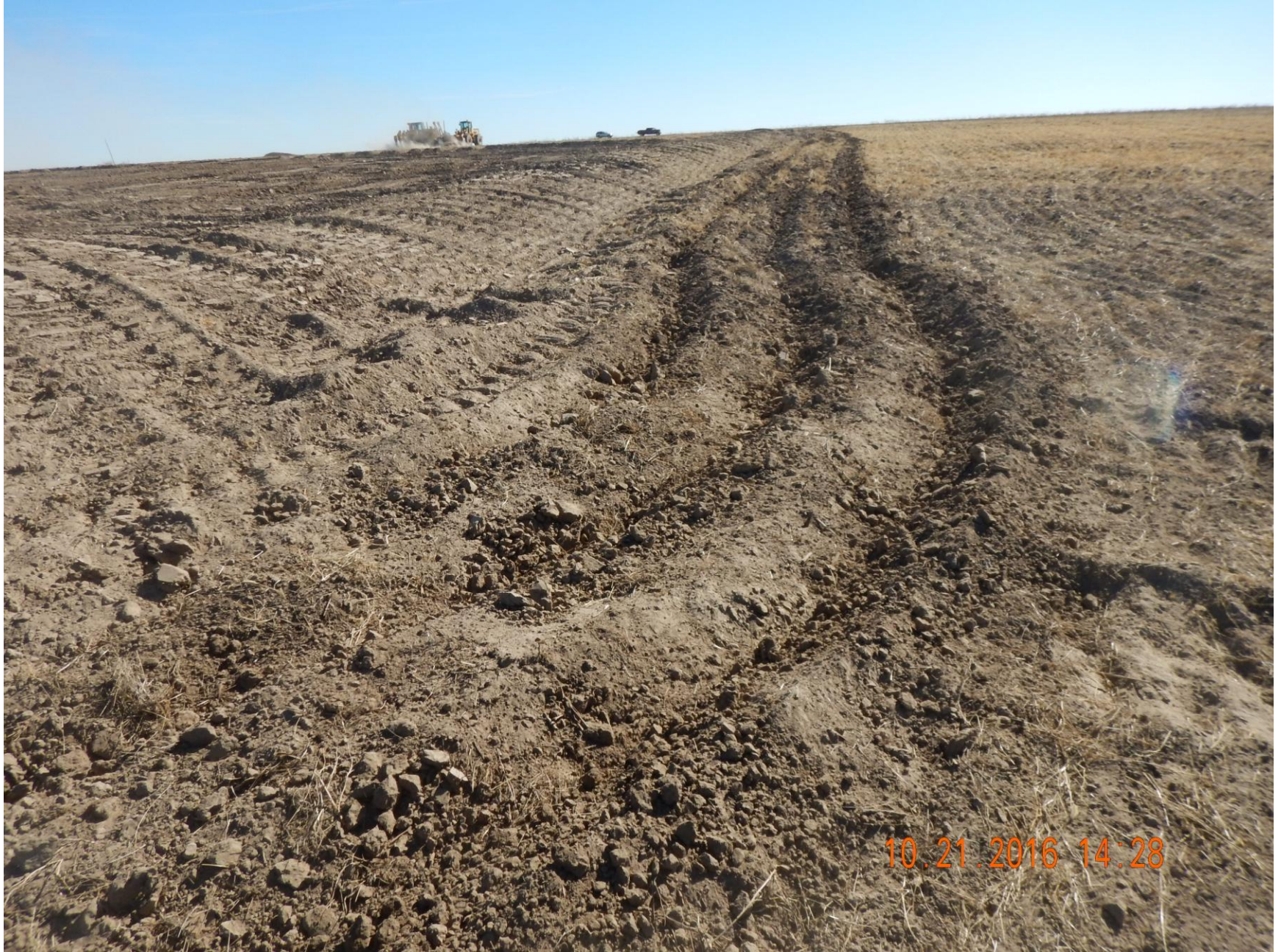
Figure 9: Photo taken from the northwest corner of the location, facing south. Photo shows surface roughening used in conjunction with berms as a stormwater and sediment control BMP.
