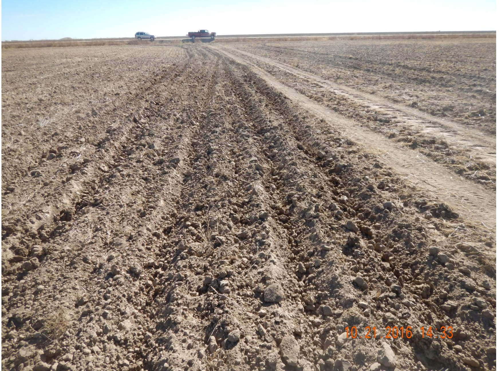
Figure 15: Photo taken from the south end of the location, facing south. Photo shows surface roughening implemented around perimeter of location
