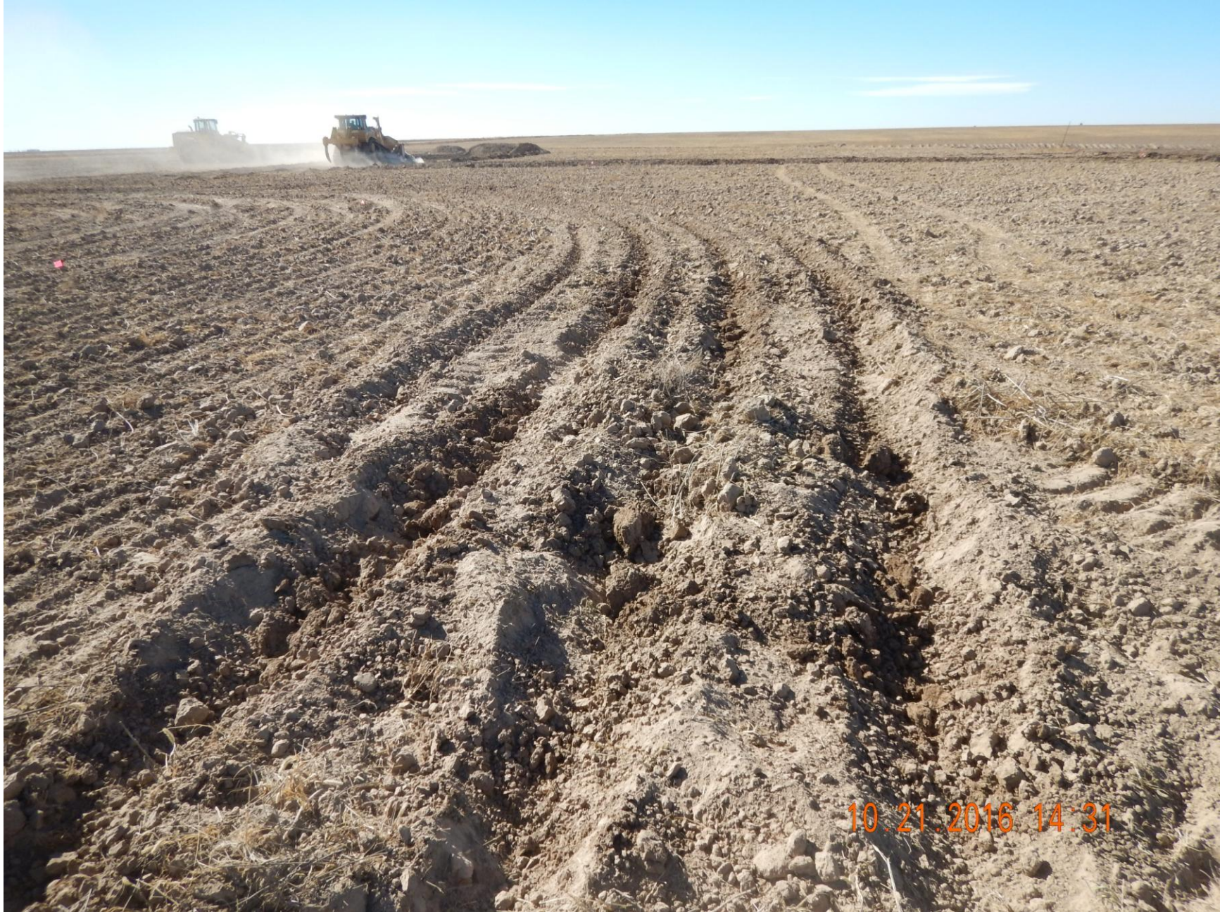
Figure 13: Photo taken from the southeast corner of the location, facing west. Photo shows surface roughening implemented around perimeter of location.
