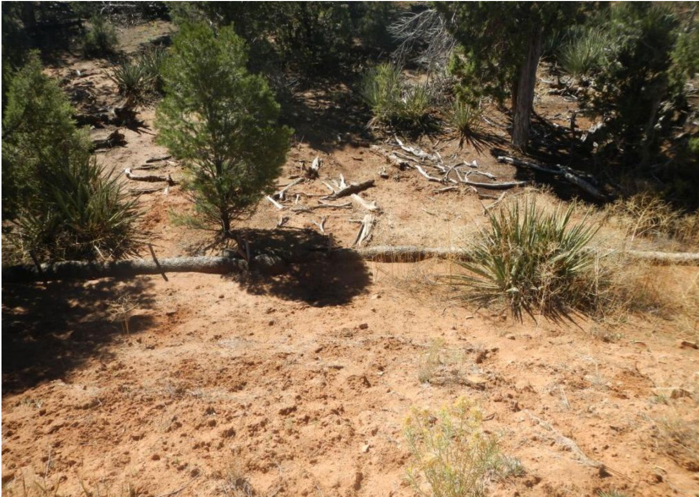
Photo 5. View of straw wattles on the northern edge of the project area.
