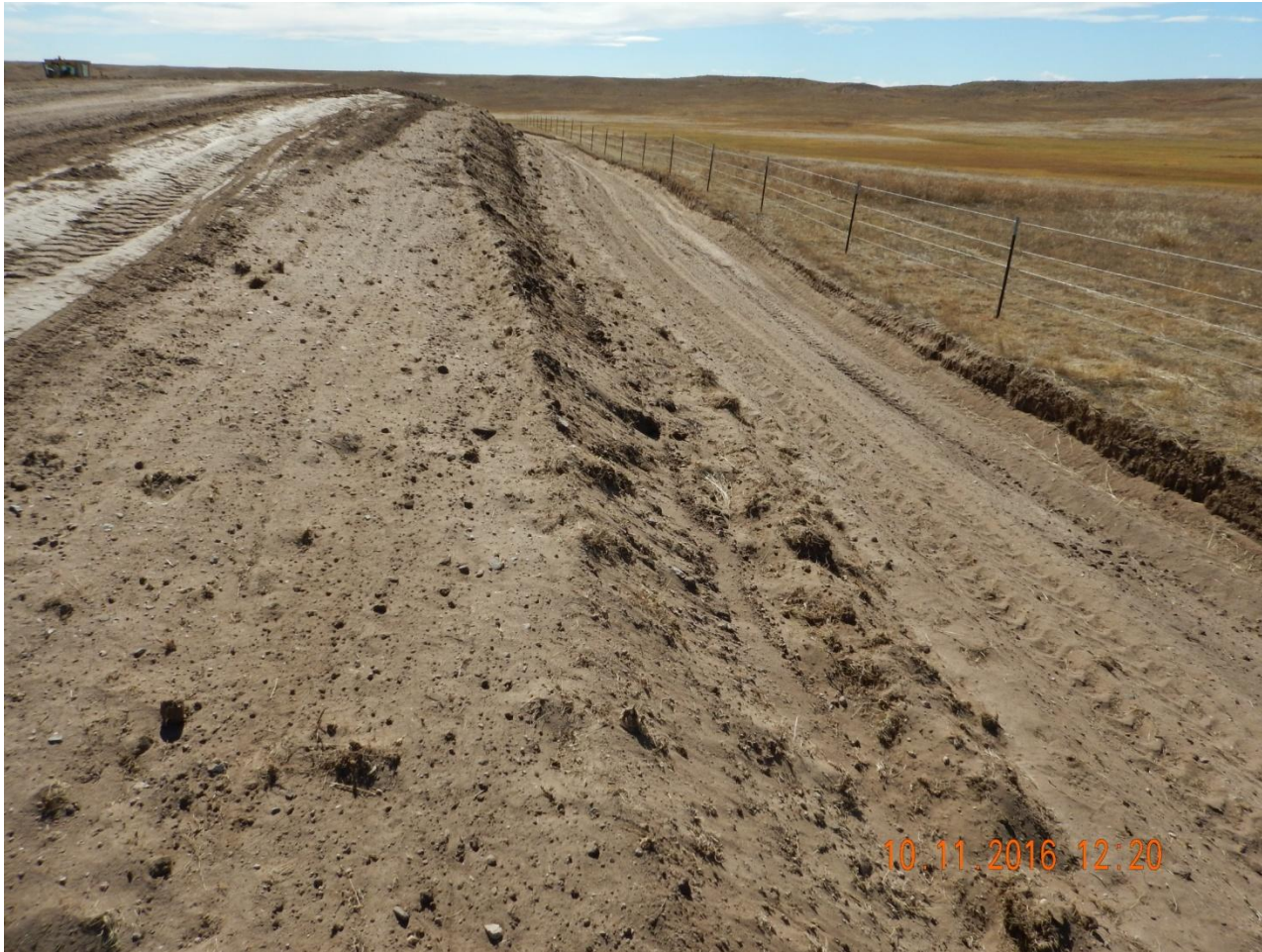
Photo 3. Photo taken from western topsoil pile, facing South. Ditch and berm constructed around outer perimeter of topsoil pile to control run-off.
