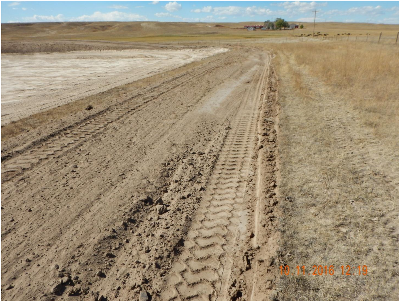
Photo 1. Photo taken from northern location, facing West. Ditch and berm constructed along northern location to control run-on onto location.
