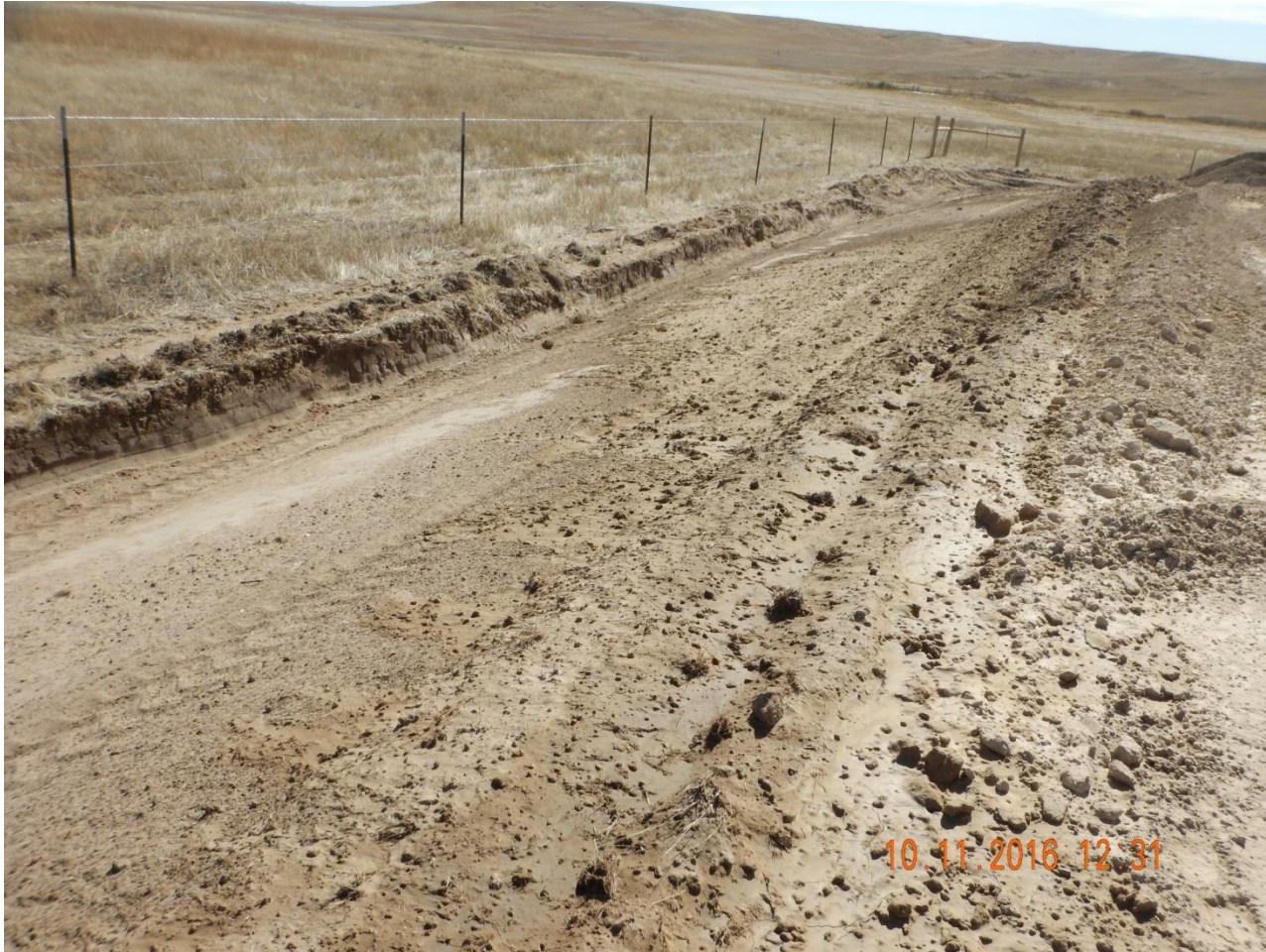
Photo 5. Photo taken from eastern location, facing South. Ditch and berm constructed along eastern location to control run-off.
