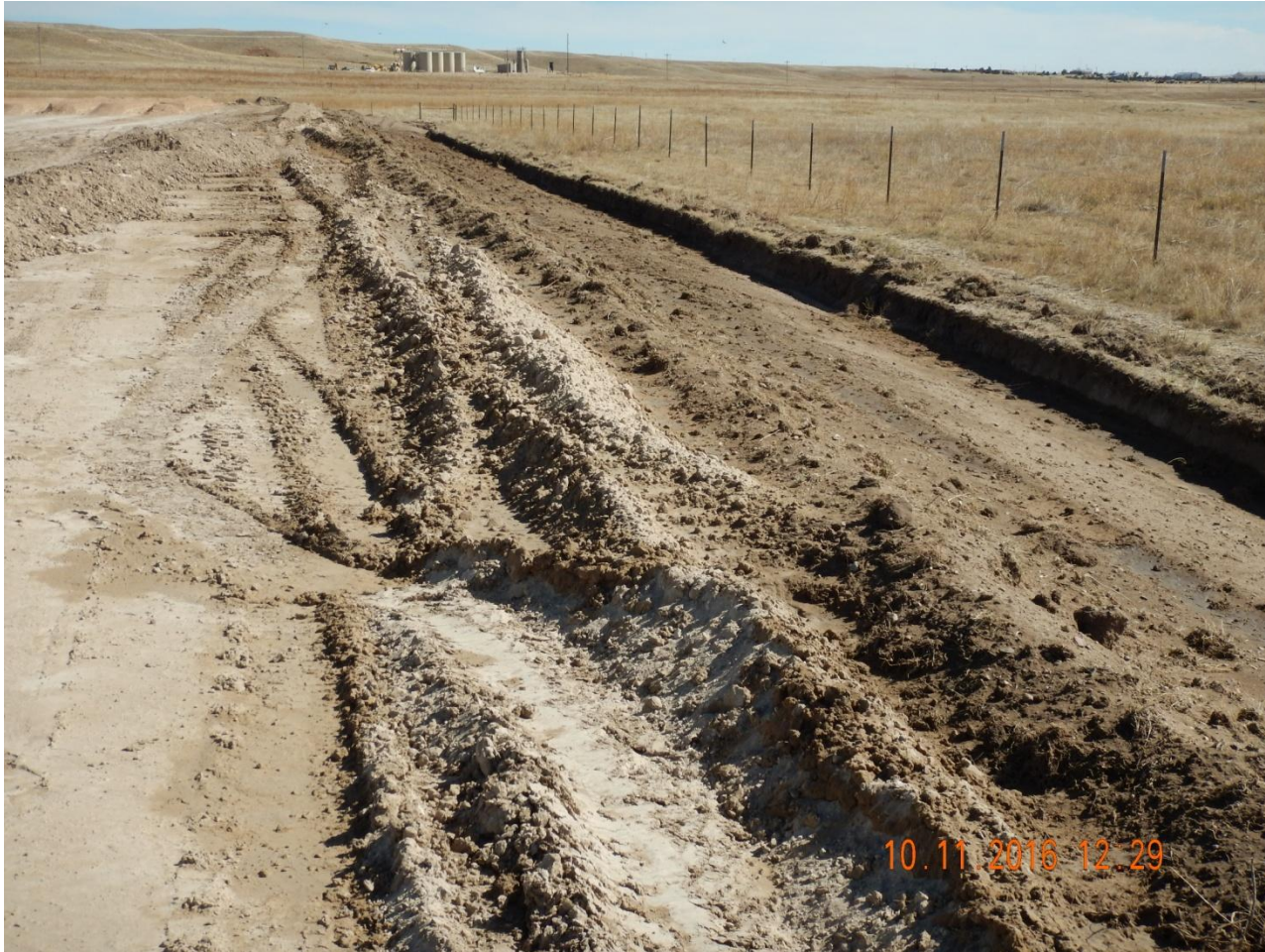
Photo 4. Photo taken from southern location, facing East. Ditch and berm constructed along southern location to control run-off. Contractor mentioned that additional BMPs would be installed along the southern location.
