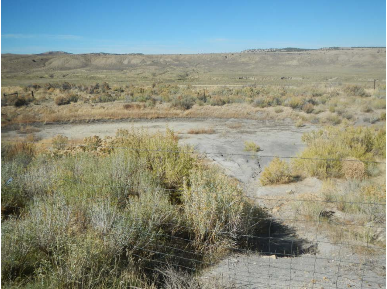
Pit 285519, fenced, no liner, weeds present around perimeter of pit no weeds in bottom. There is a poly line in the bottom of the pit, it is unclear where the flowline is coming from.
