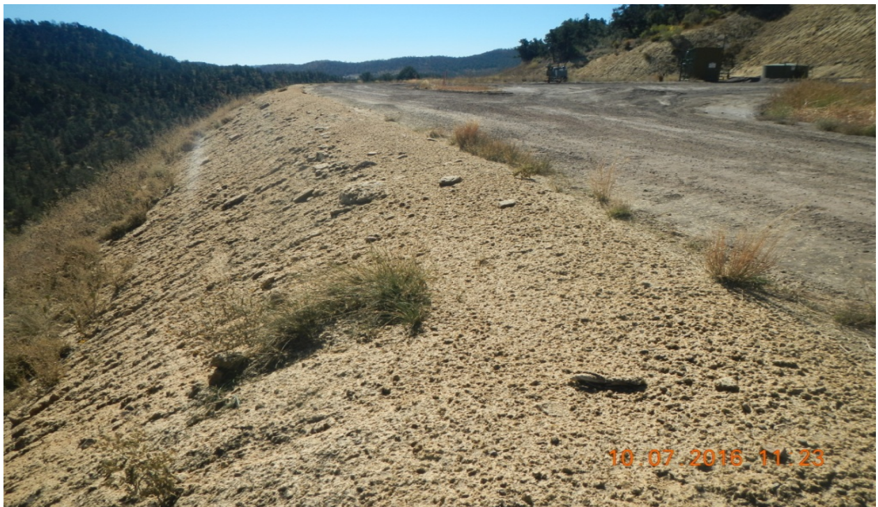
photo 8: Facing southeast at the location. The location has been seeded and hydro-mulched.
