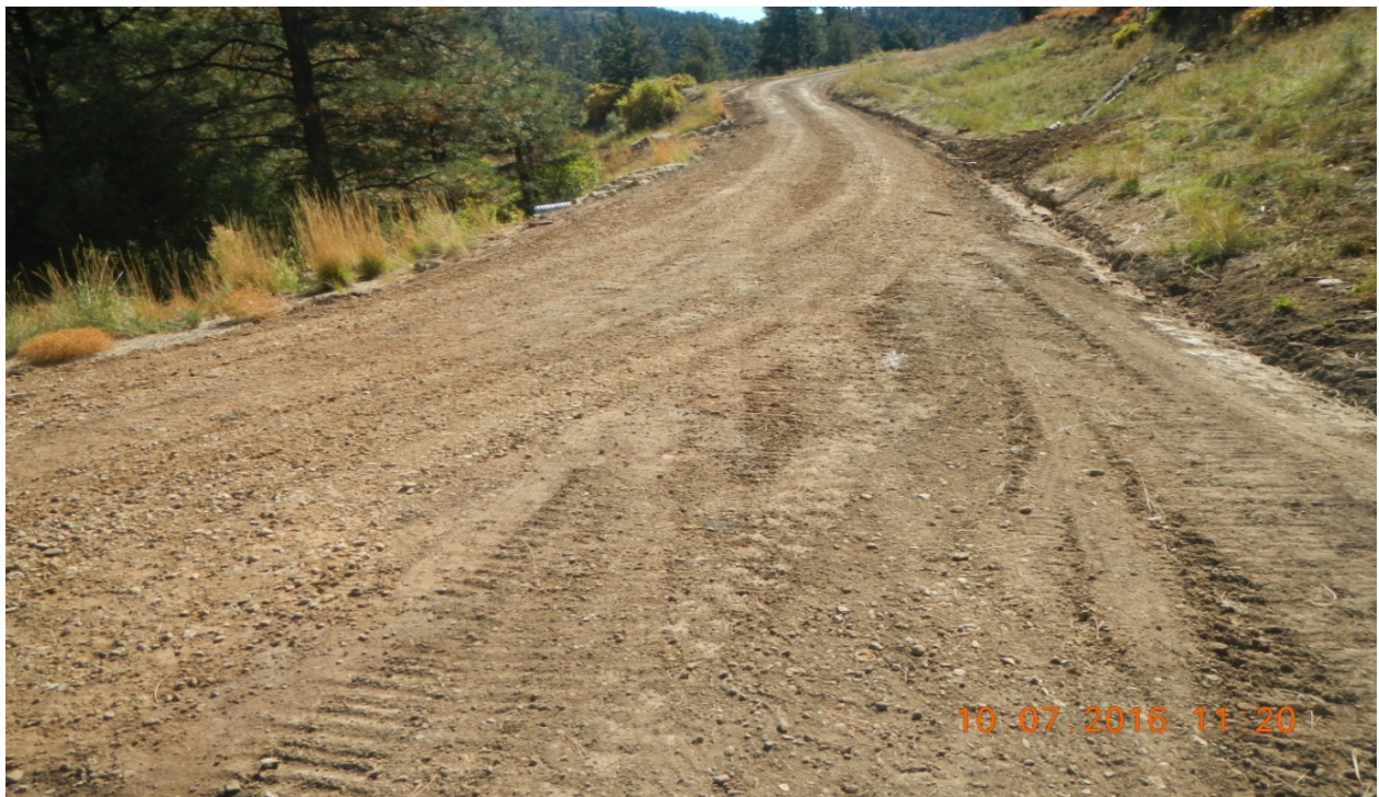
photo 6: Facing southeast along the main access road. Erosion issues have been corrected.
