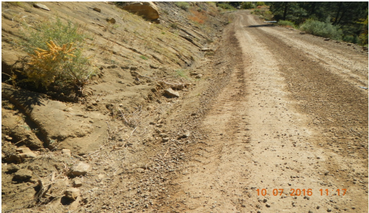
photo 4: Facing southwest along the main access road. Erosion issues have been corrected. Note: Stormwater flow along the access road should be de-energized by installing check dams, ect..
