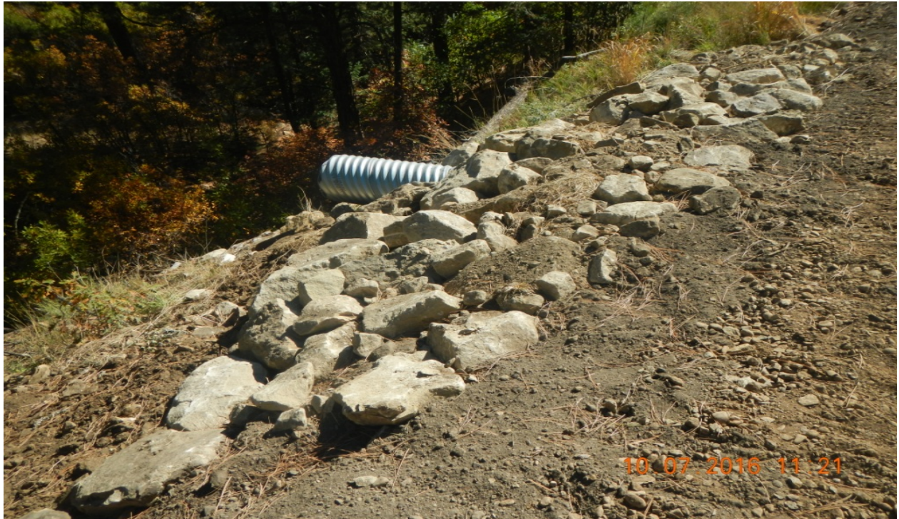
photo 7: A culvert has been installed where water was flowing across the road. Outlet protect has been placed at the culvert.
