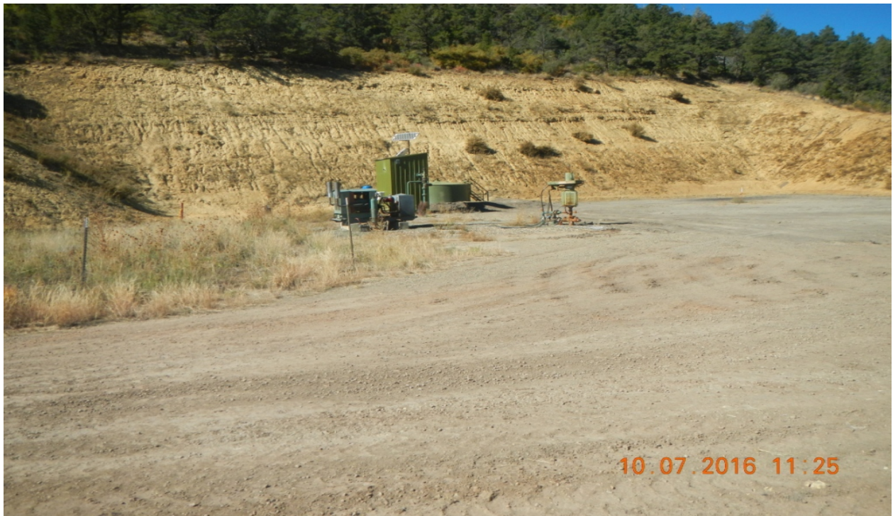
photo 10: Facing west toward the cut slope which has been seeded and hydro-mulched.
