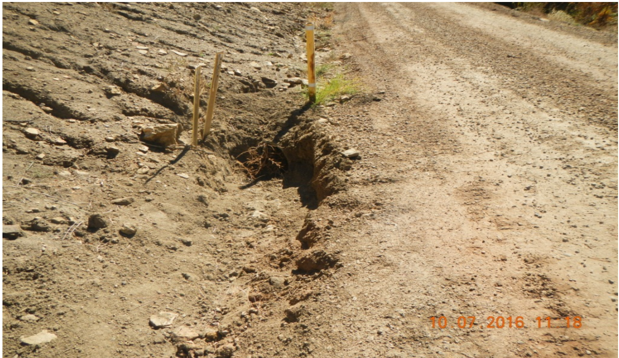
photo 5: The main road switches back to the northeast at this point. Erosion issues have been corrected.
