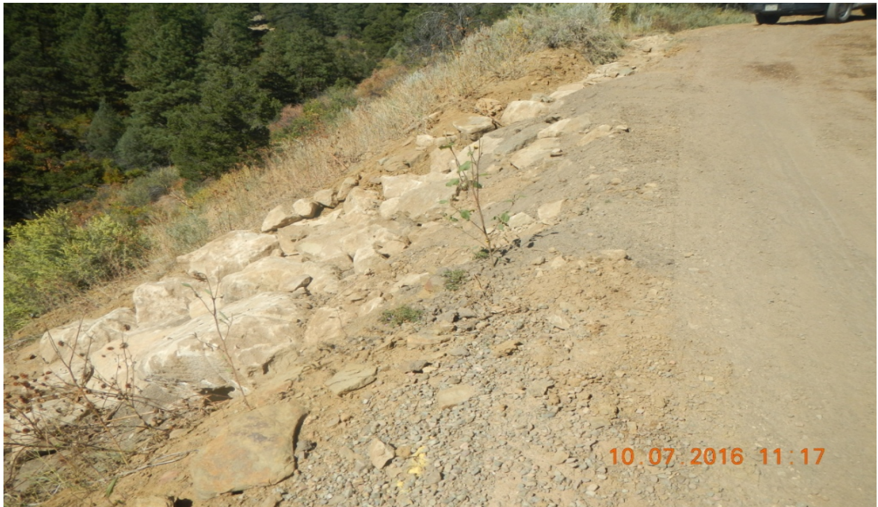
photo 3: Rock rip/rap has been installed along the road.
