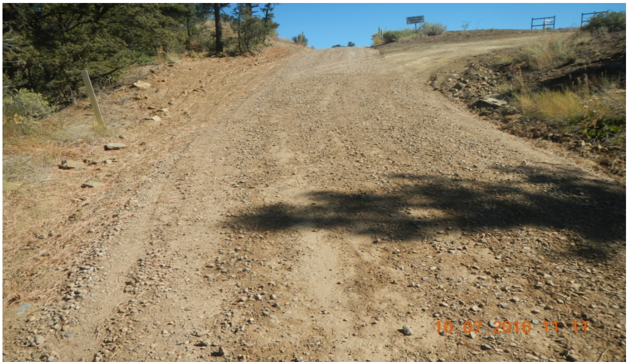
photo 6: Facing northeast along the main access road. Erosion issues have been corrected.
