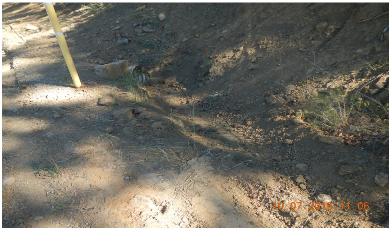
photo 2: The culverts have been cleaned and maintained.
