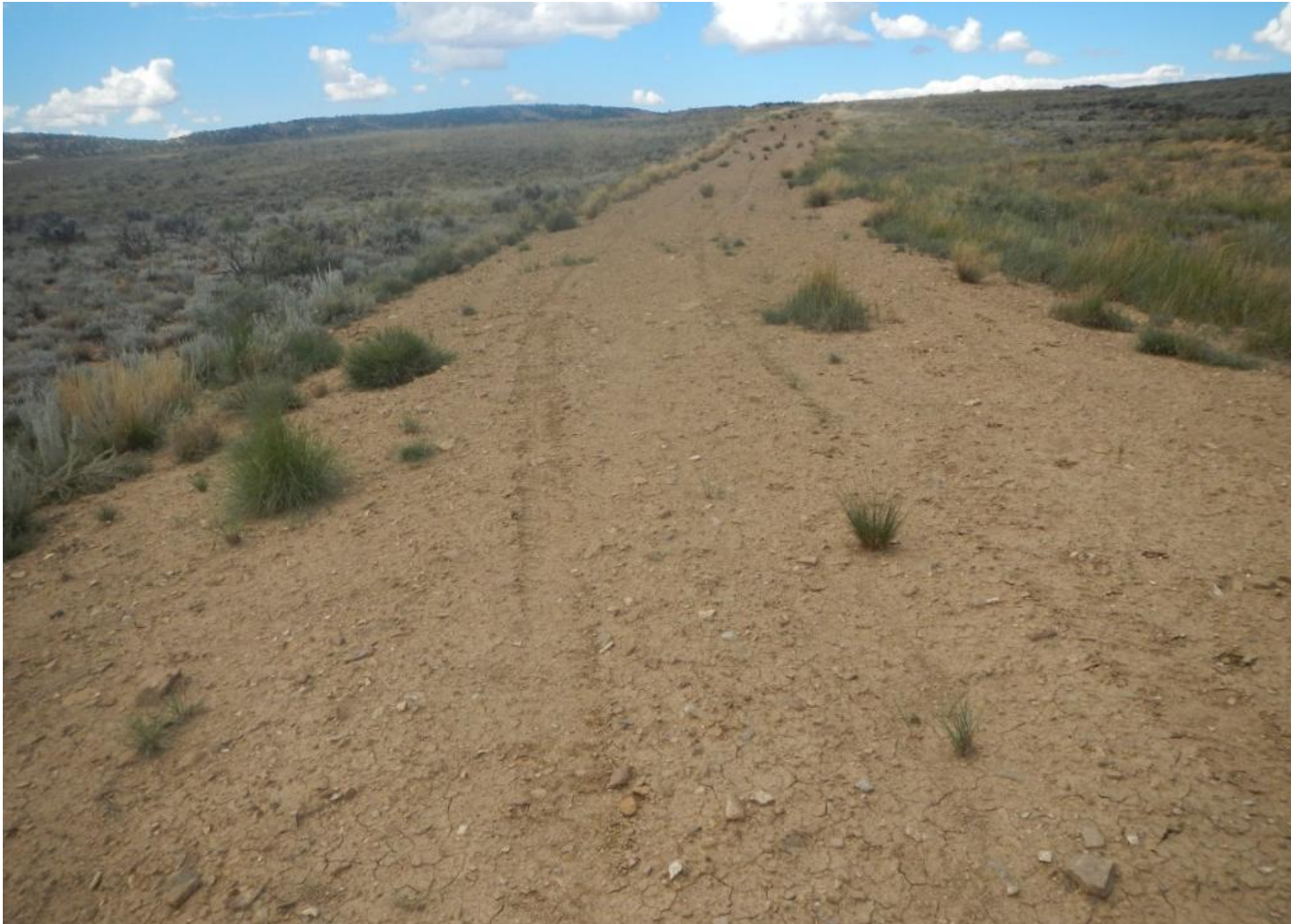
Photo 1. View from the end of the access near the well pad entrance facing westward. Access road has not been reclaimed and needs to be fully reclaimed.
