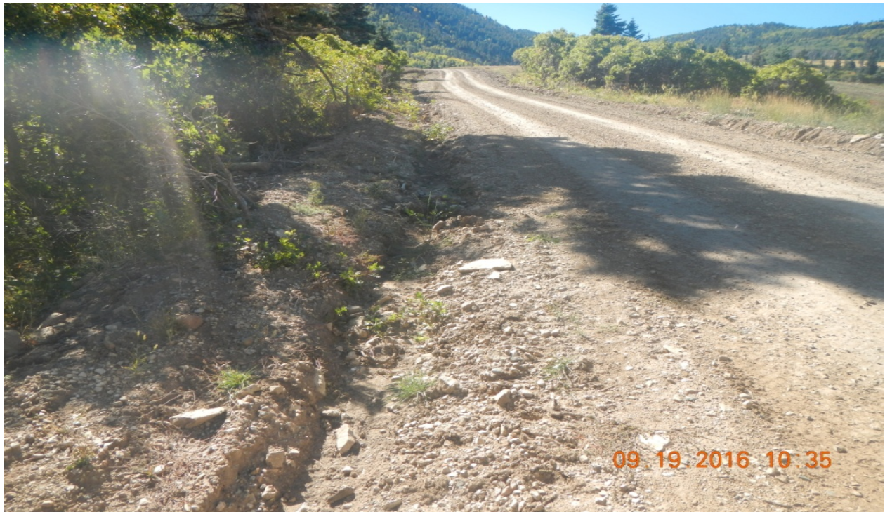
photo 1: Facing south along access road near the location. There are no BMP's to de-energize stormwater that flows down the side of the access road.
