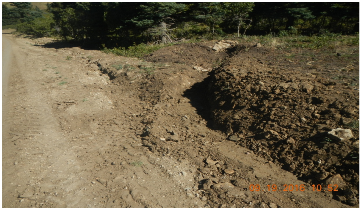
photo 2: Facing along the access road near the location. There is a sediment trap that has been installed.
