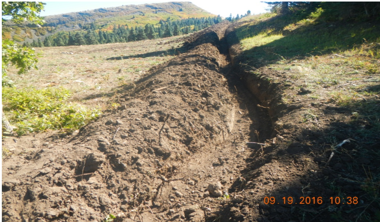
photo 6: A ditch has been installed along the south cut slope side of the location. Additional BMP's should be installed to de-energize stormwater flow within the ditch.
