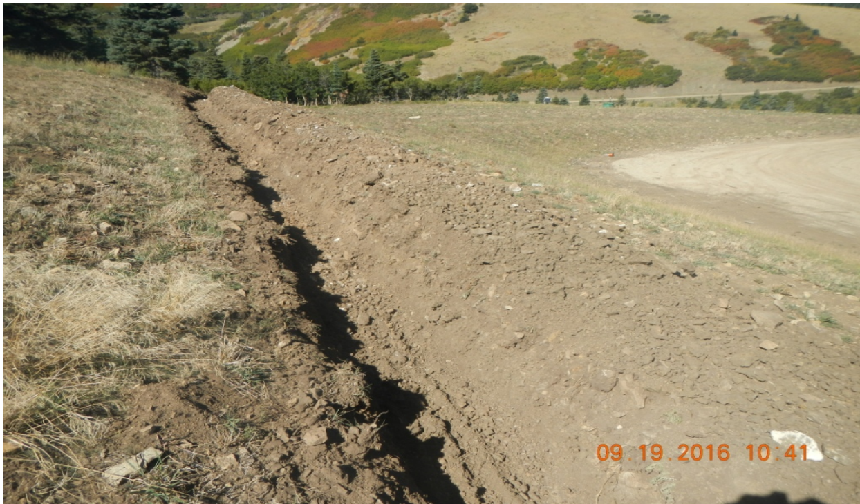
photo 7: Facing northwest along the south side of the location. Additional BMP's should be installed to de-energize stormwater flow within the ditch.
