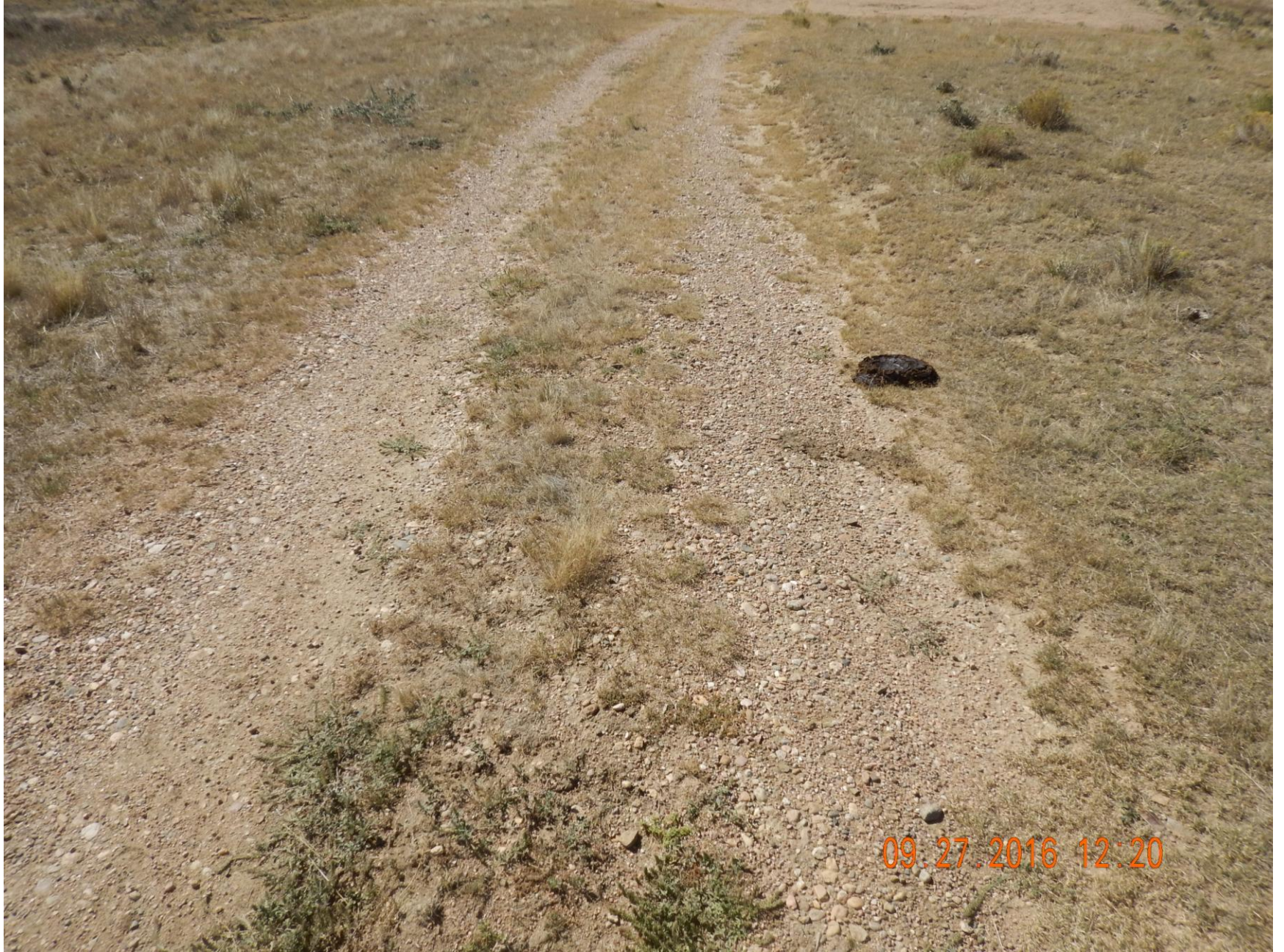
Figure 11: Photo taken from access road immediately north of the location, facing south. Photo shows access road has not been reclaimed, including removal of gravel.
