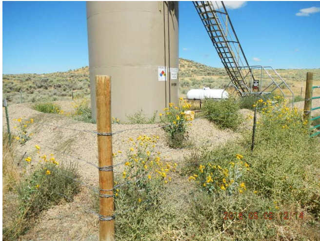
Tank battery bermed.
