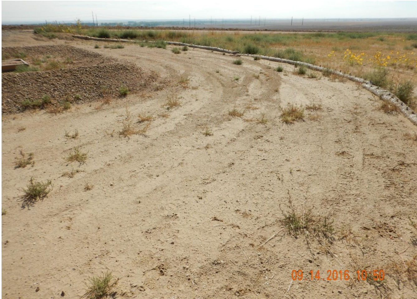
Photo 1. Photo taken from the western location, facing Southeast. Straw wattles installed to control sedimentation from leaving location.
