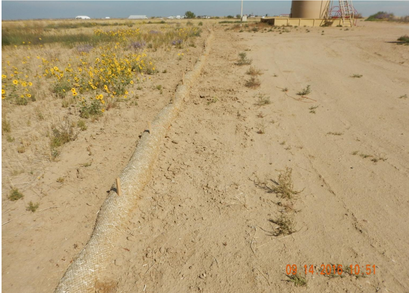
Photo 2. Photo taken from the western location, facing North. Straw wattles installed to control sedimentation from leaving location.
