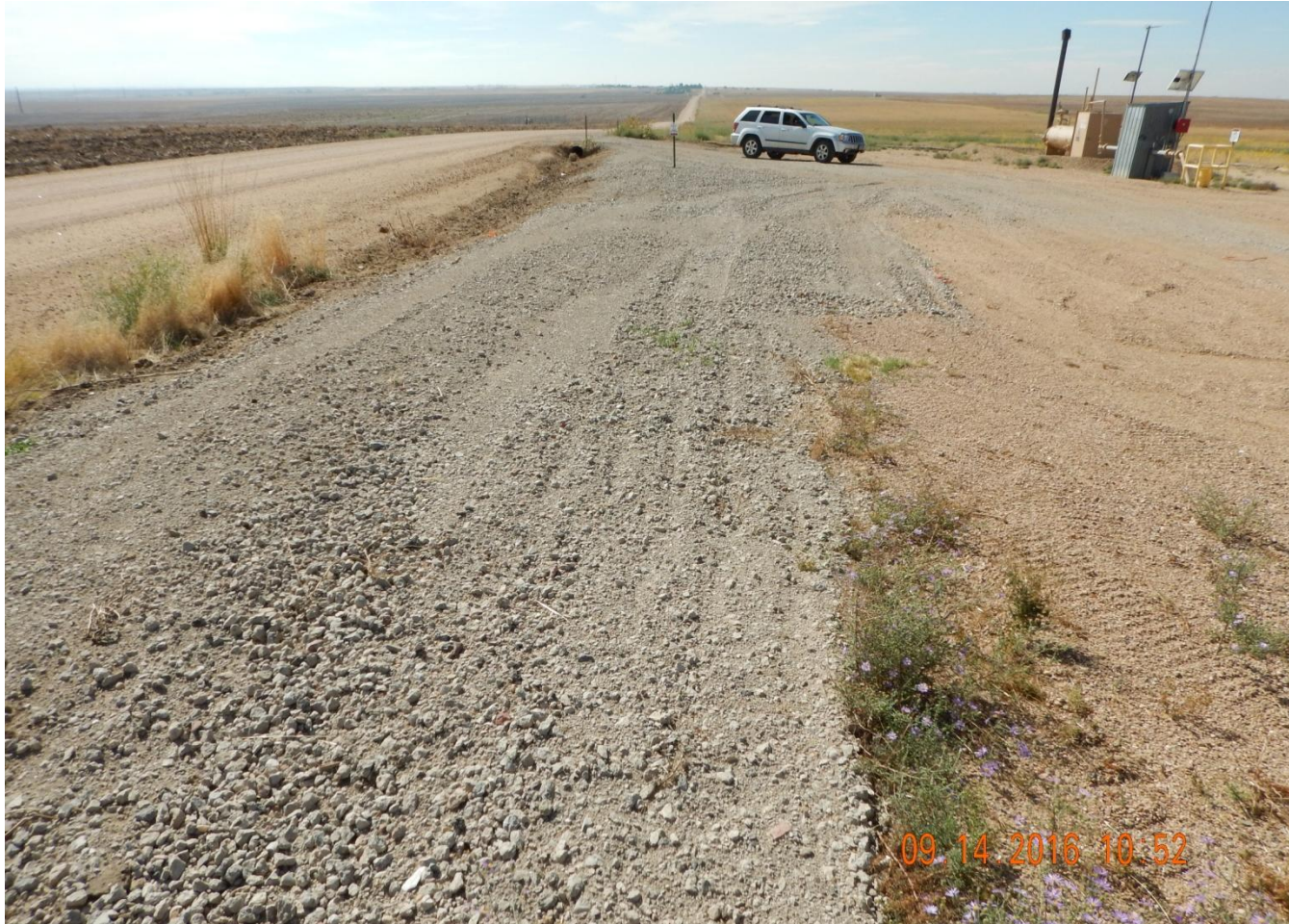
Photo 3. Photo taken from the eastern location, facing South. Gravel installed to stabilize location and prevent erosion.
