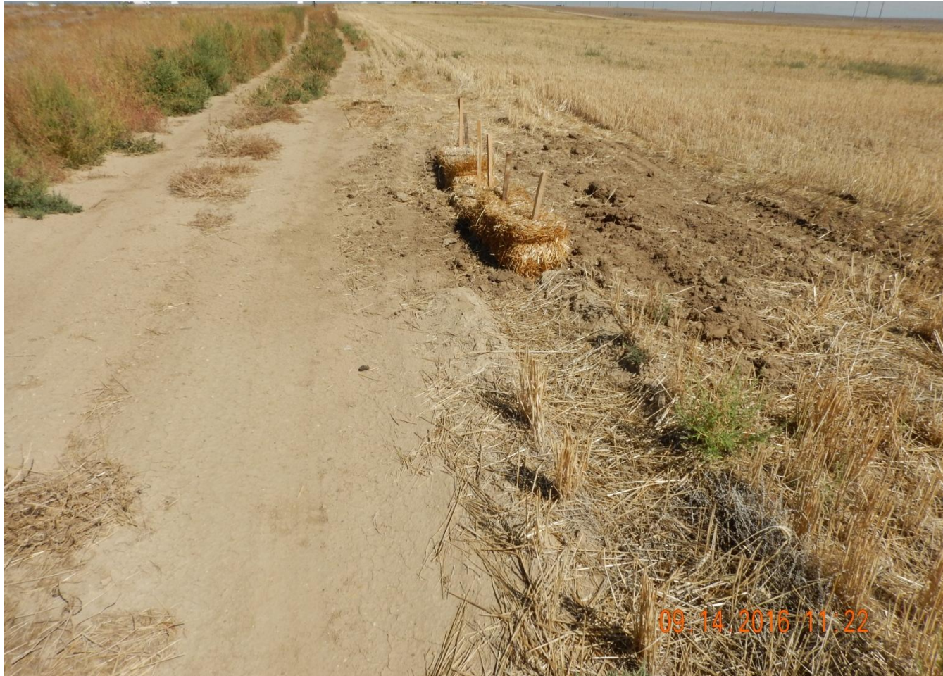
Photo 2. Photo taken from the lease road, facing North. Straw bales installed to control sedimentation from leaving lease road. Stormwater could possibly travel around straw bales because location lacks diversion features.
