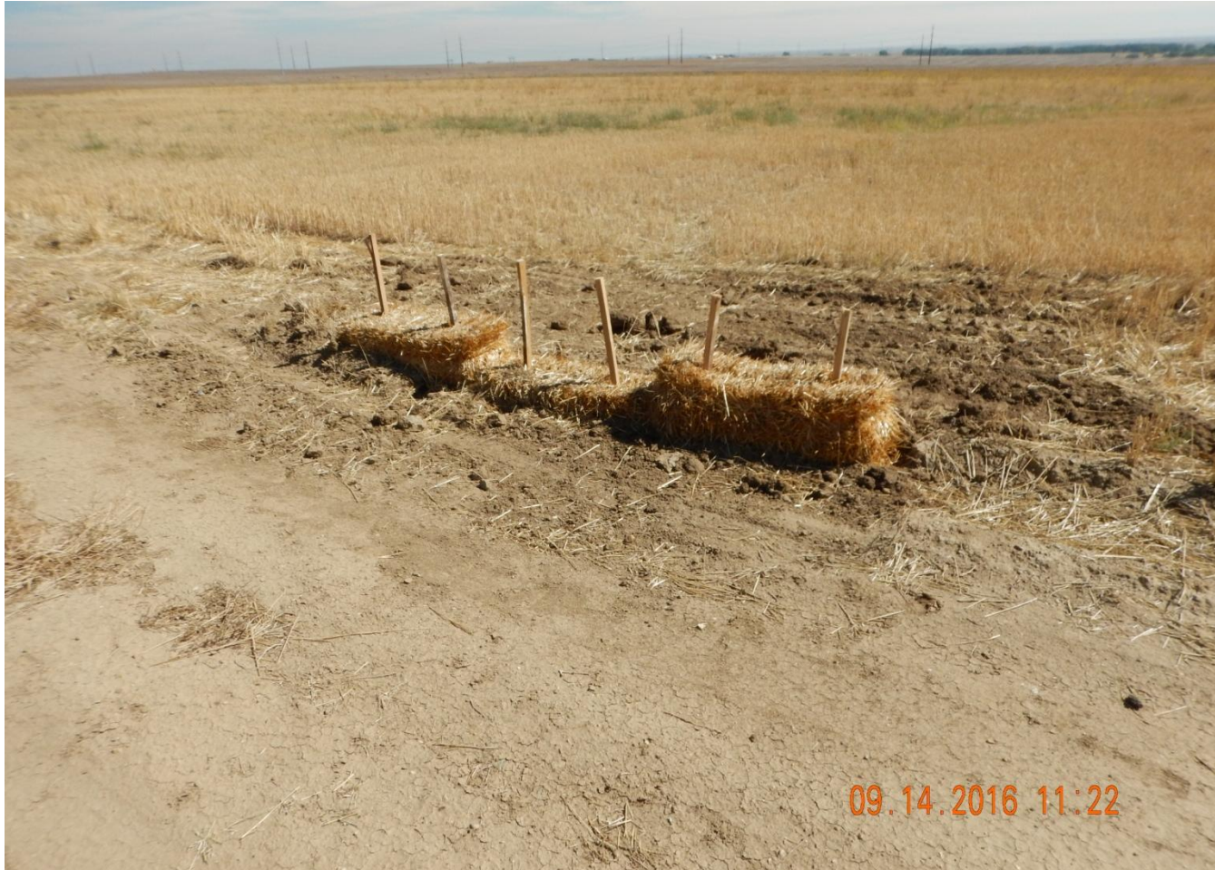
Photo 1. Photo taken from the lease road, facing East. Straw bales installed to control sedimentation from leaving lease road. Stormwater could possibly travel around straw bales because location lacks diversion features.
