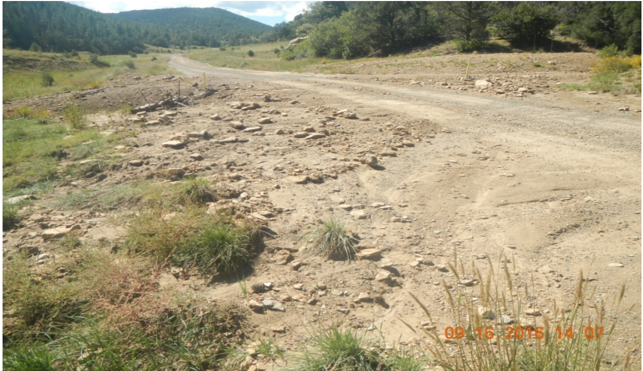
photo 1: Facing west along the main access road. The culverts are filled with sediment and stormwater washed away gravel and deposited sediment on the road.
