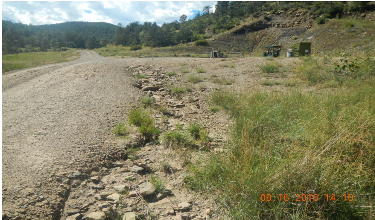
photo 3: Facing west toward the location. There are signs of erosion at this area.
