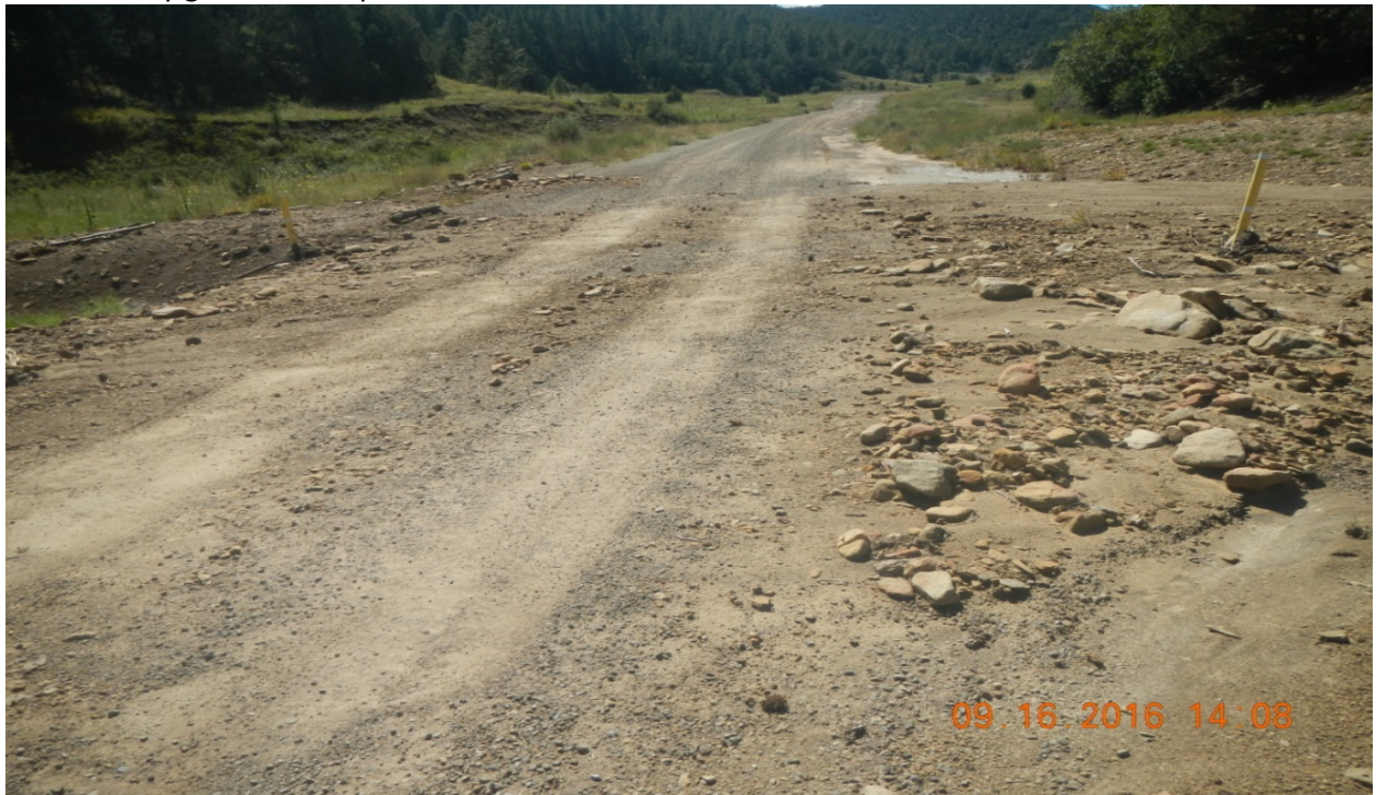
photo 2: Facing west along the main access road. The culverts are filled with sediment and stormwater washed away gravel and deposited sediment on the road.
