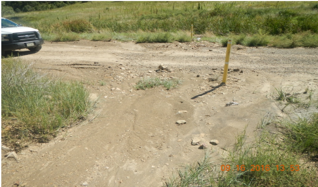
photo 5: The culvert along the main road is filled in with sediment.
