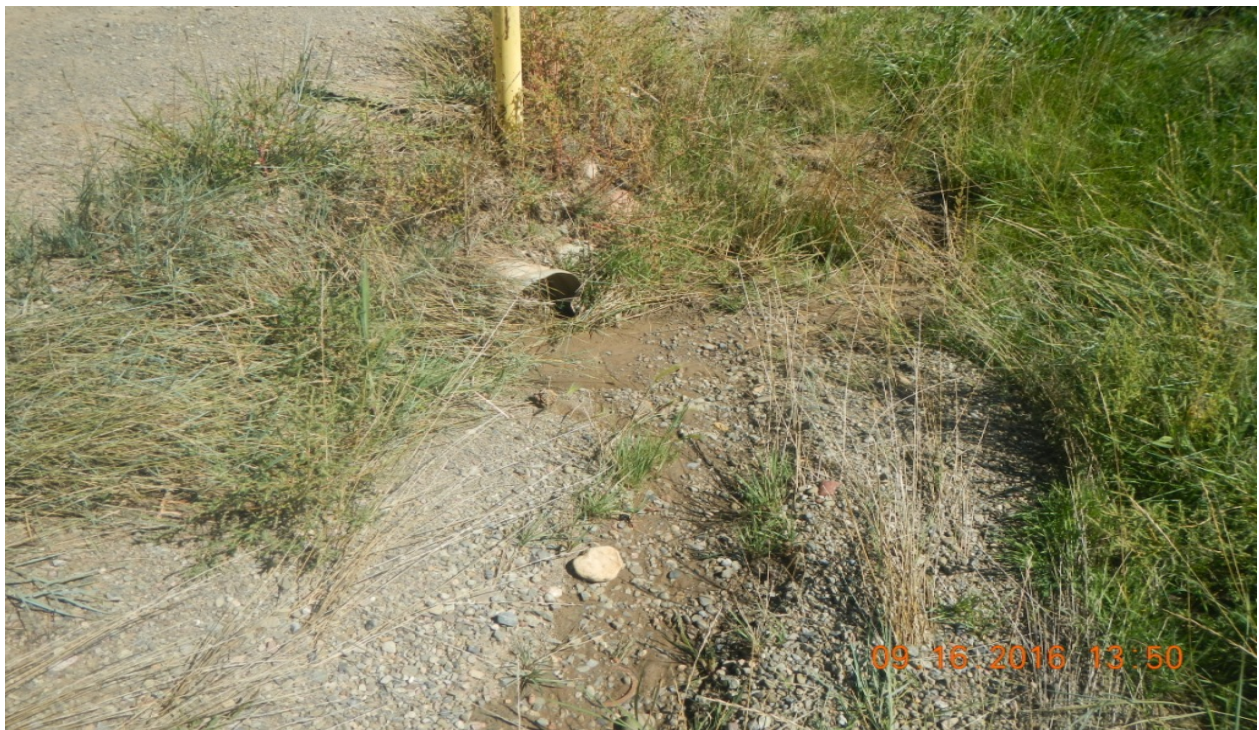
photo 2: The culvert along the access road is filling in with sediment.
