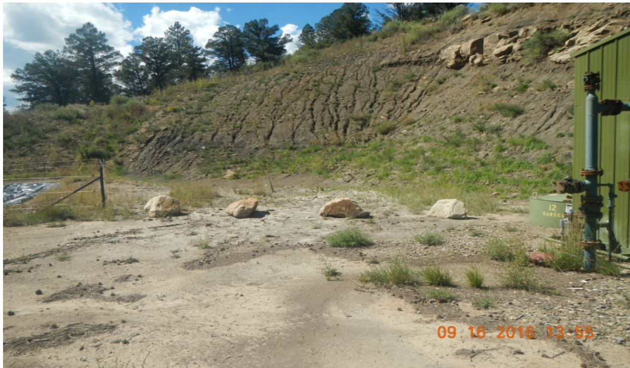
photo 8: Facing toward the northwest side of the location. There are signs of erosion along the cut slope.
