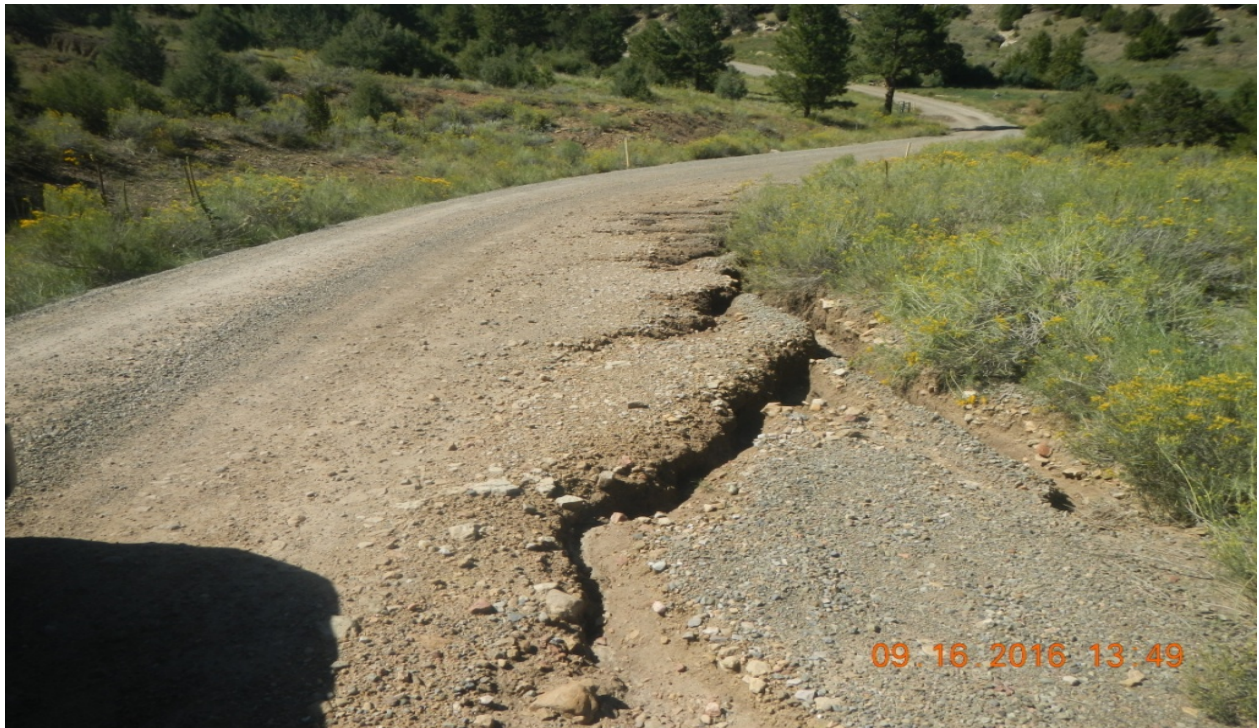
photo 1: Facing west along the main access road. There are signs of erosion occurring on the main road.
