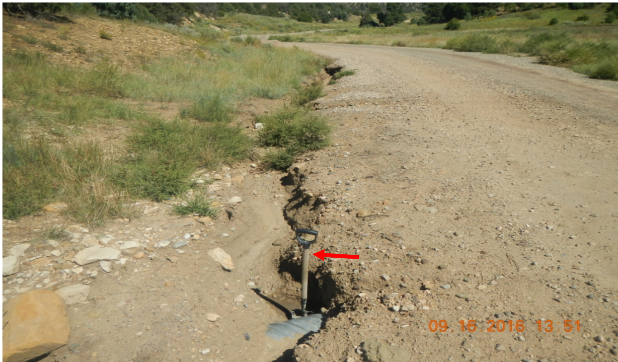
photo 4: There is erosion occurring along the access road. Red arrow points to 3 ft. shovel.
