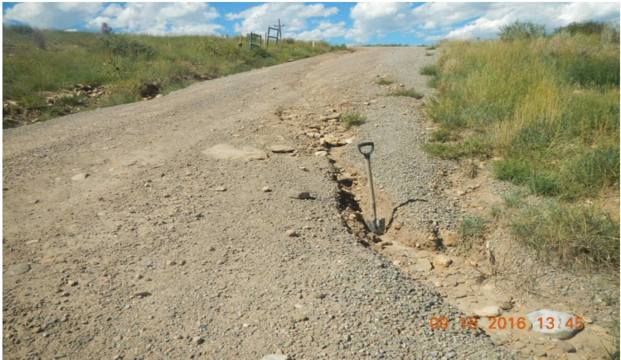
photo 1: There is an erosion channel along the main road near the location.
