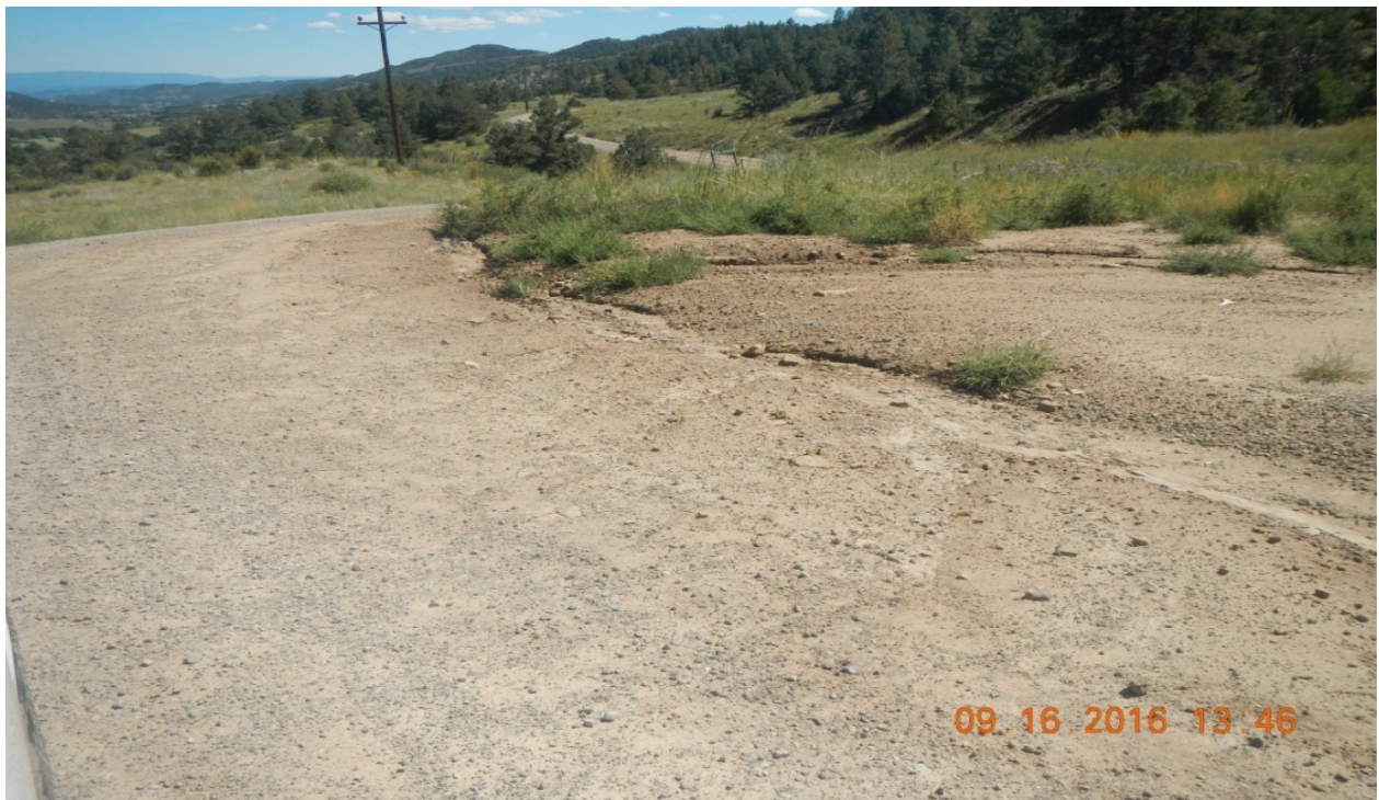
photo 2: Facing back toward the east at the location. There are signs of stormwater flowing toward the main road causing erosion.
