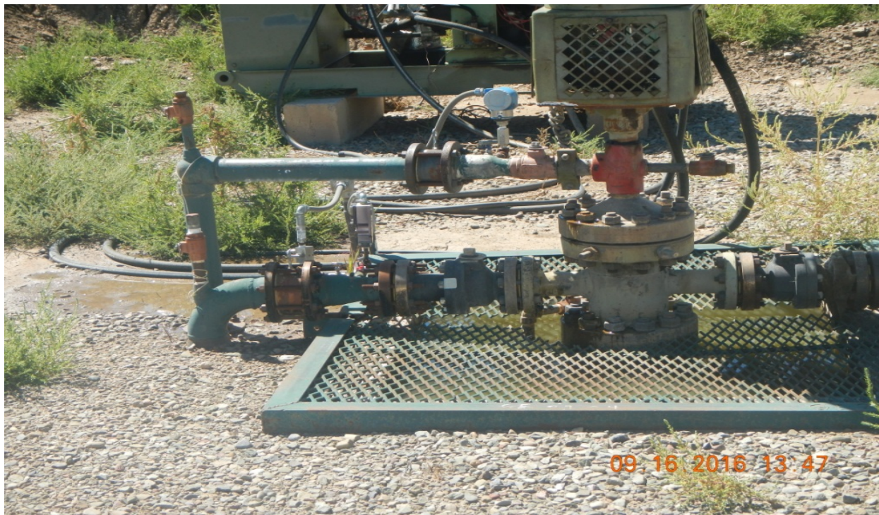
photo 3: There was a dripping water leak noticed at the well head.
