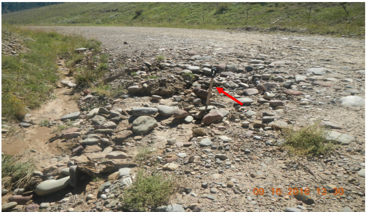
photo 2: There is erosion occurring across the main road and there is no culvert present to divert stormwater. Red arrow points to 3 ft. shovel.
