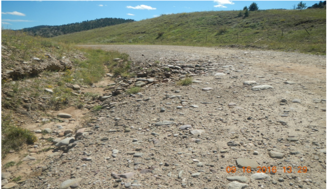
photo 1: Facing southeast along the access road toward the location. There is erosion occurring across the main road and there is no culvert present to divert stormwater.
