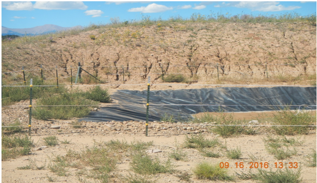
photo 4: Facing west toward the cut where there is signs of erosion.
