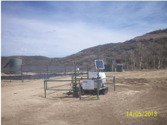
PAD LOCATION LOOKING NORTH
