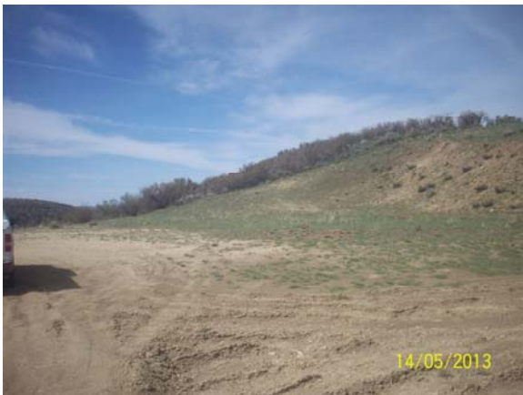
PAD OVERALL LOOKING SOUTHWESTERLY
