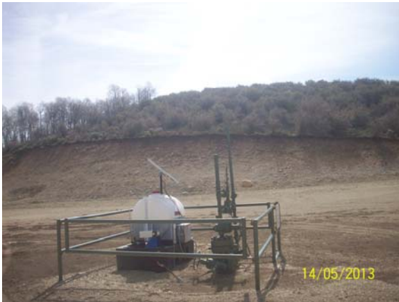
PAD LOCATION LOOKING WEST
