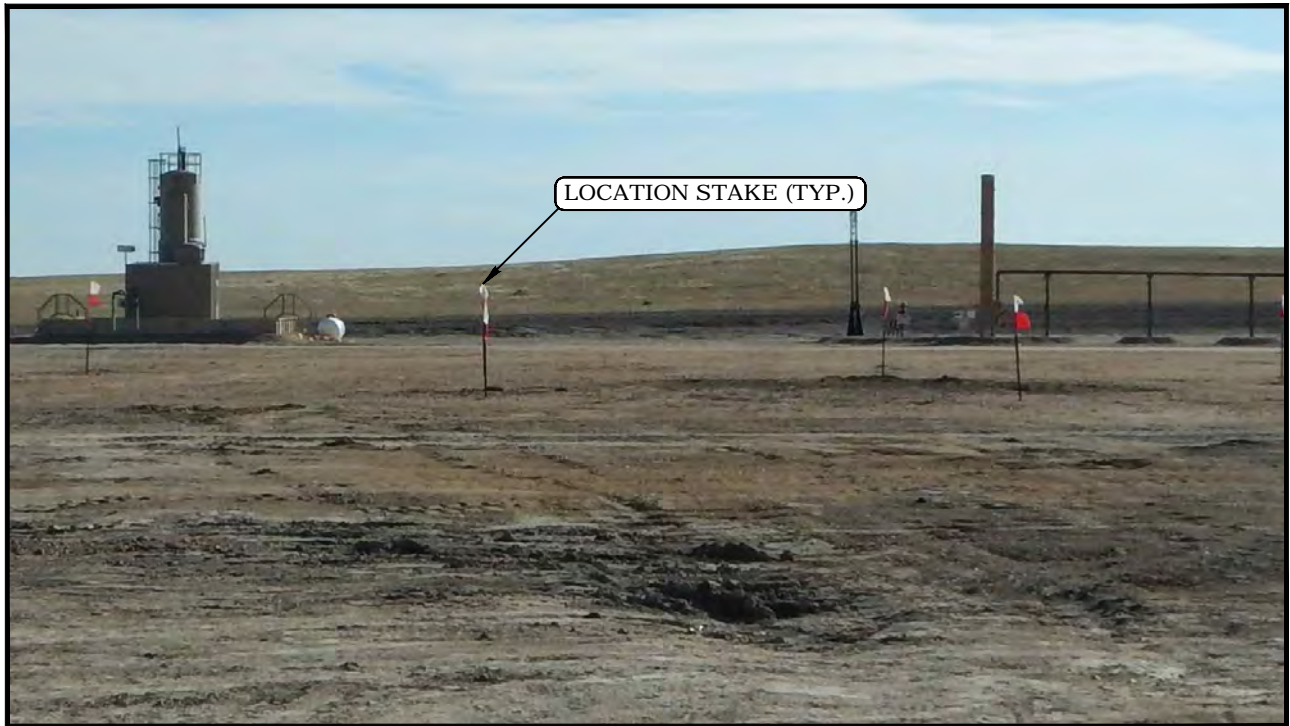
PHOTO: VIEW OF LOCATION STAKES
