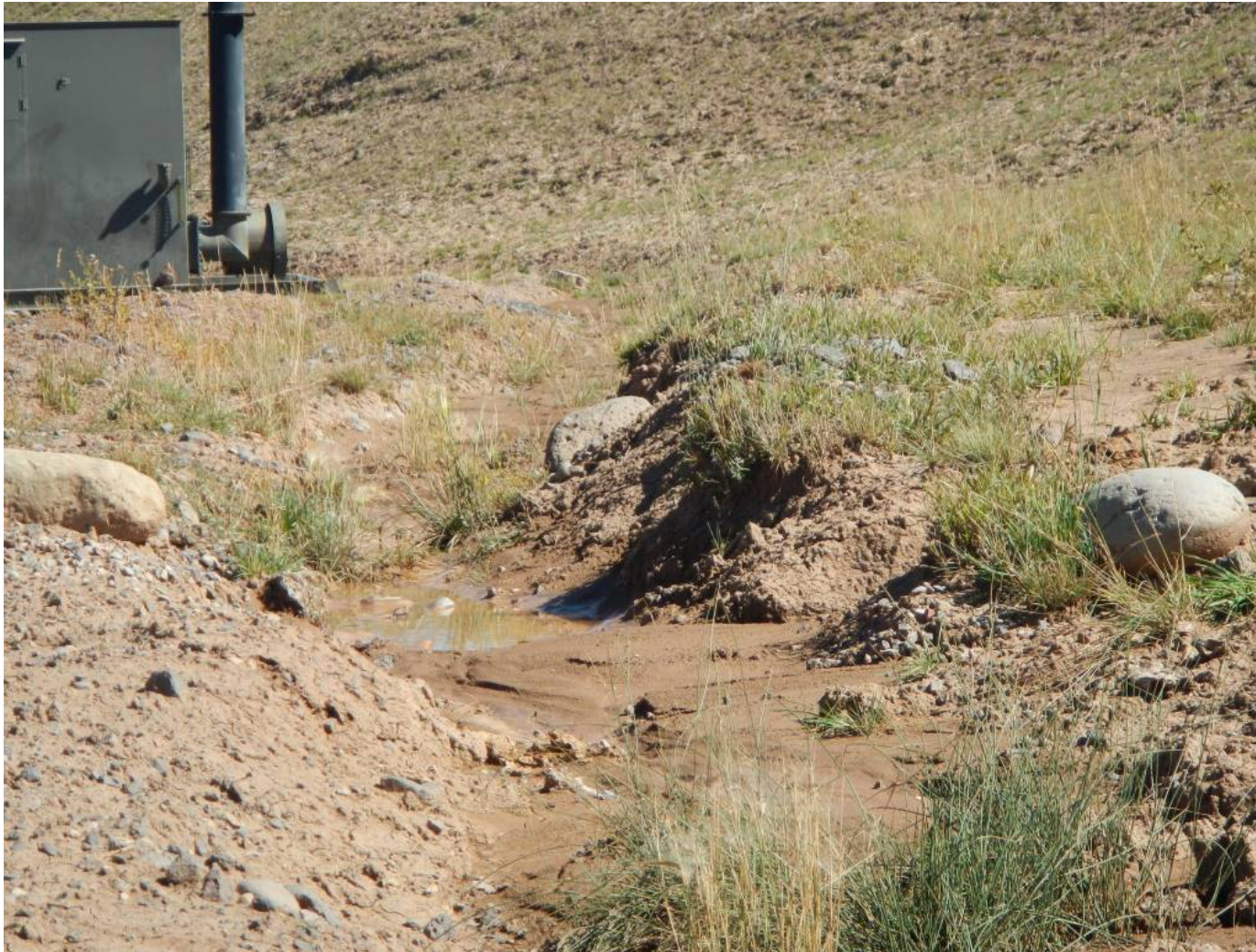
Photo#9: Sediment migrating from Cut Slope to Ditch at Slope Base.
