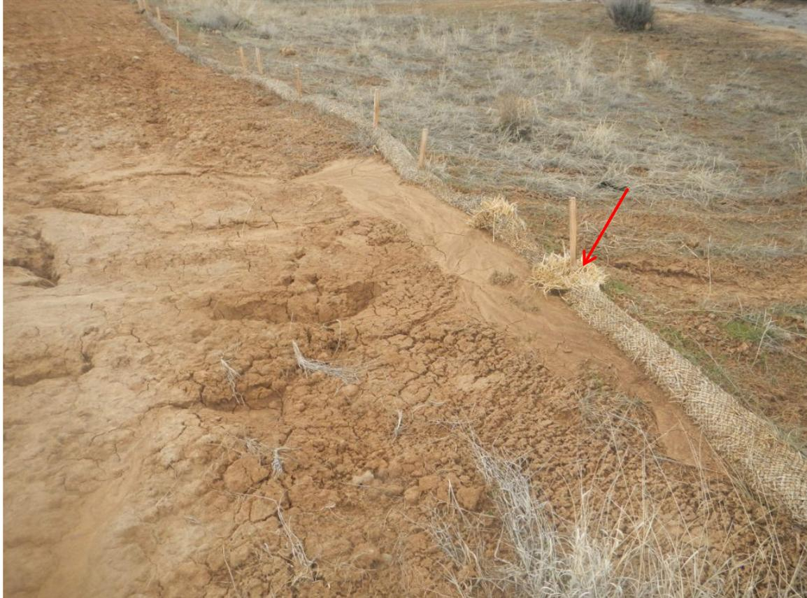
Photo#5: Wattles are being overwhelmed by excessive Runoff from Location; also more evidence of ATV damage to BMPs.
