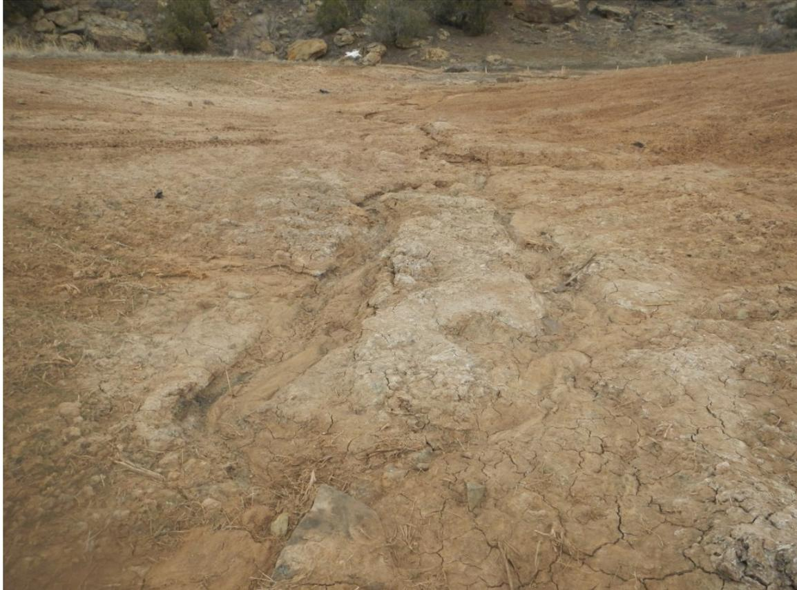
Photo#7: Revegetating areas and drainage swales need stabilizing BMPs installed until vegetation is established.
