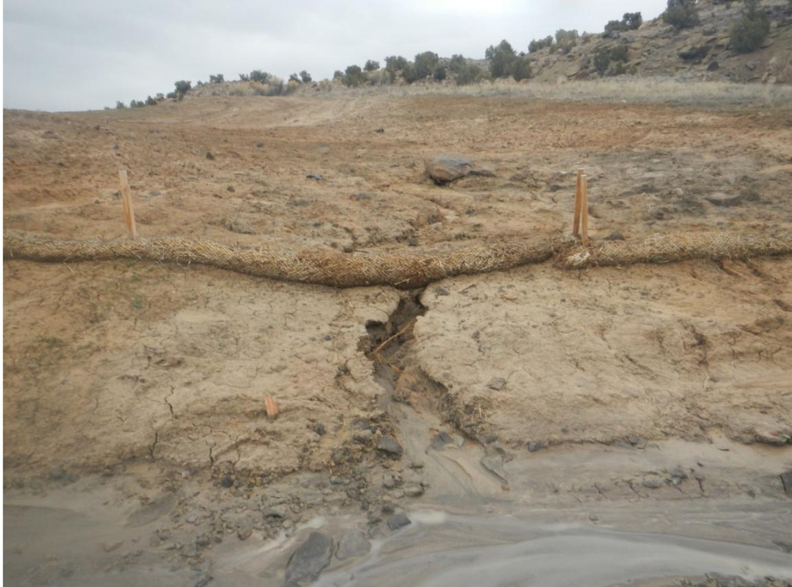
Photo#6: Stormwater undercutting Wattles at South end of Location.
