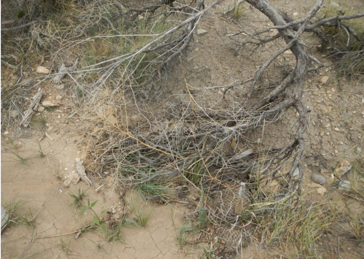
Photo 10. View of straw wattle on the southwestern edge of the project area that is filled with sediment.
