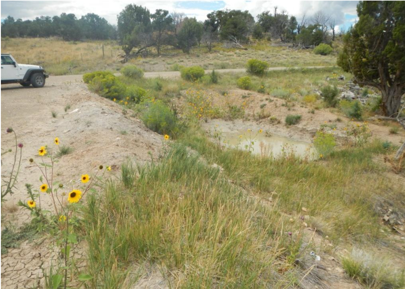
Photo 7. View of silt trap in the western portion of the project area.
