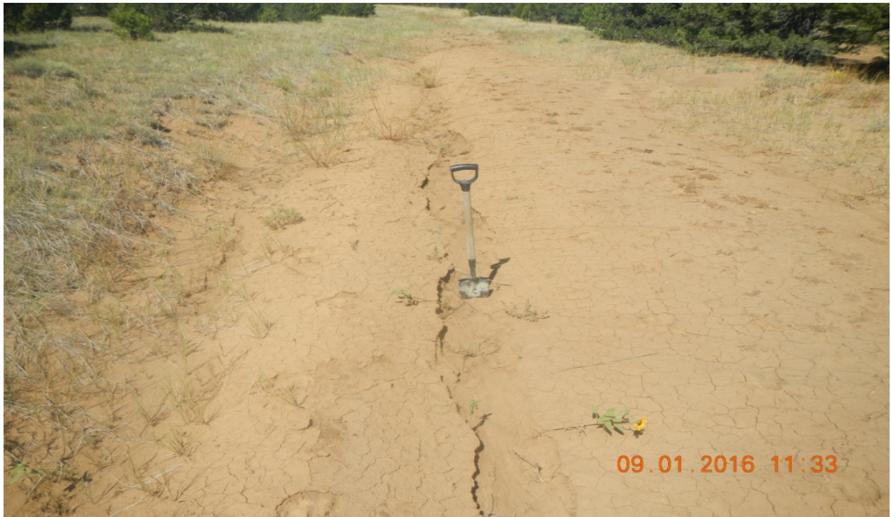
photo 1: Facing northwest along the access road toward the location. There is an erosion channel which is developing along the road near the location.
