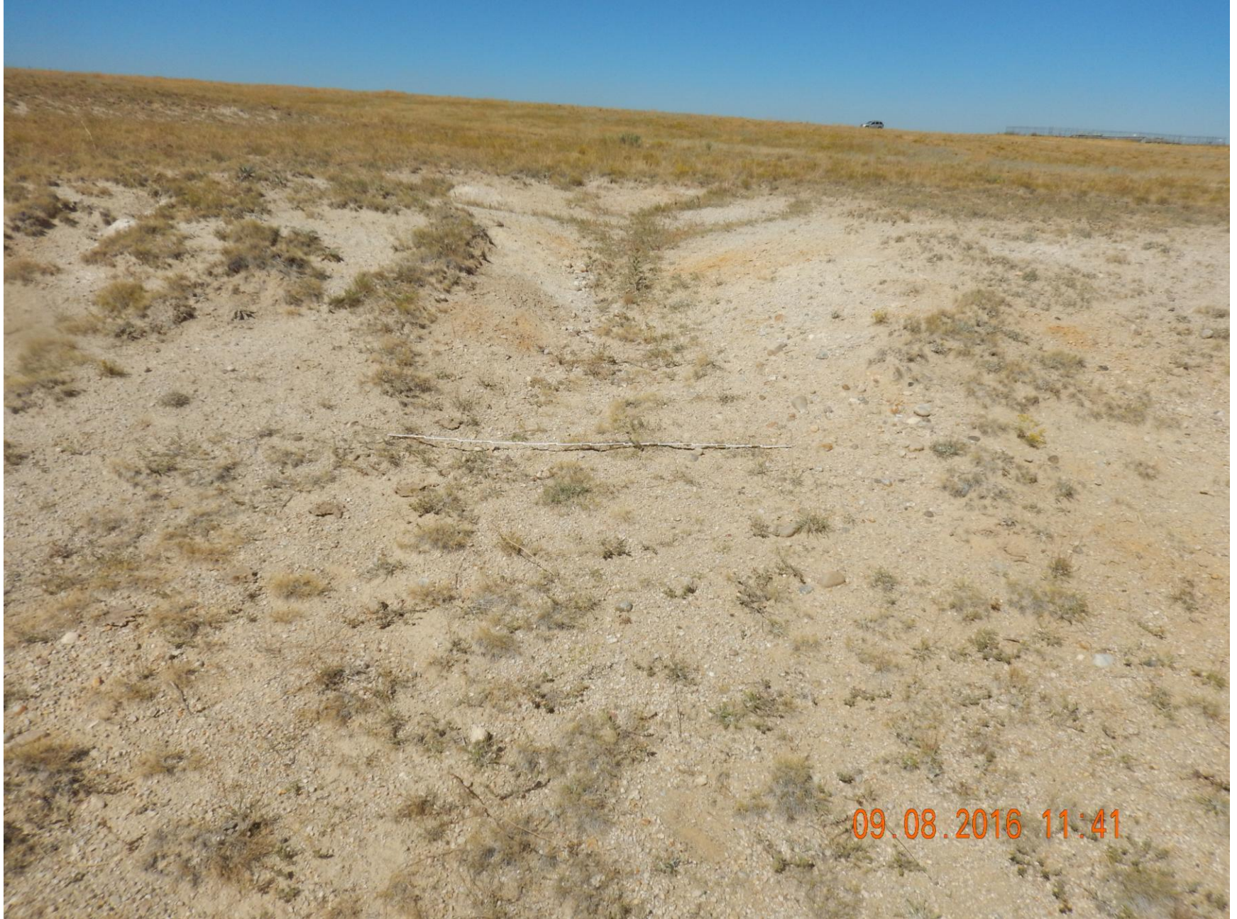
Figure 12: Photo taken from the west end of the location, facing west. Photo shows stormwater erosion occurring on slopes. 6' measuring stick for reference.
