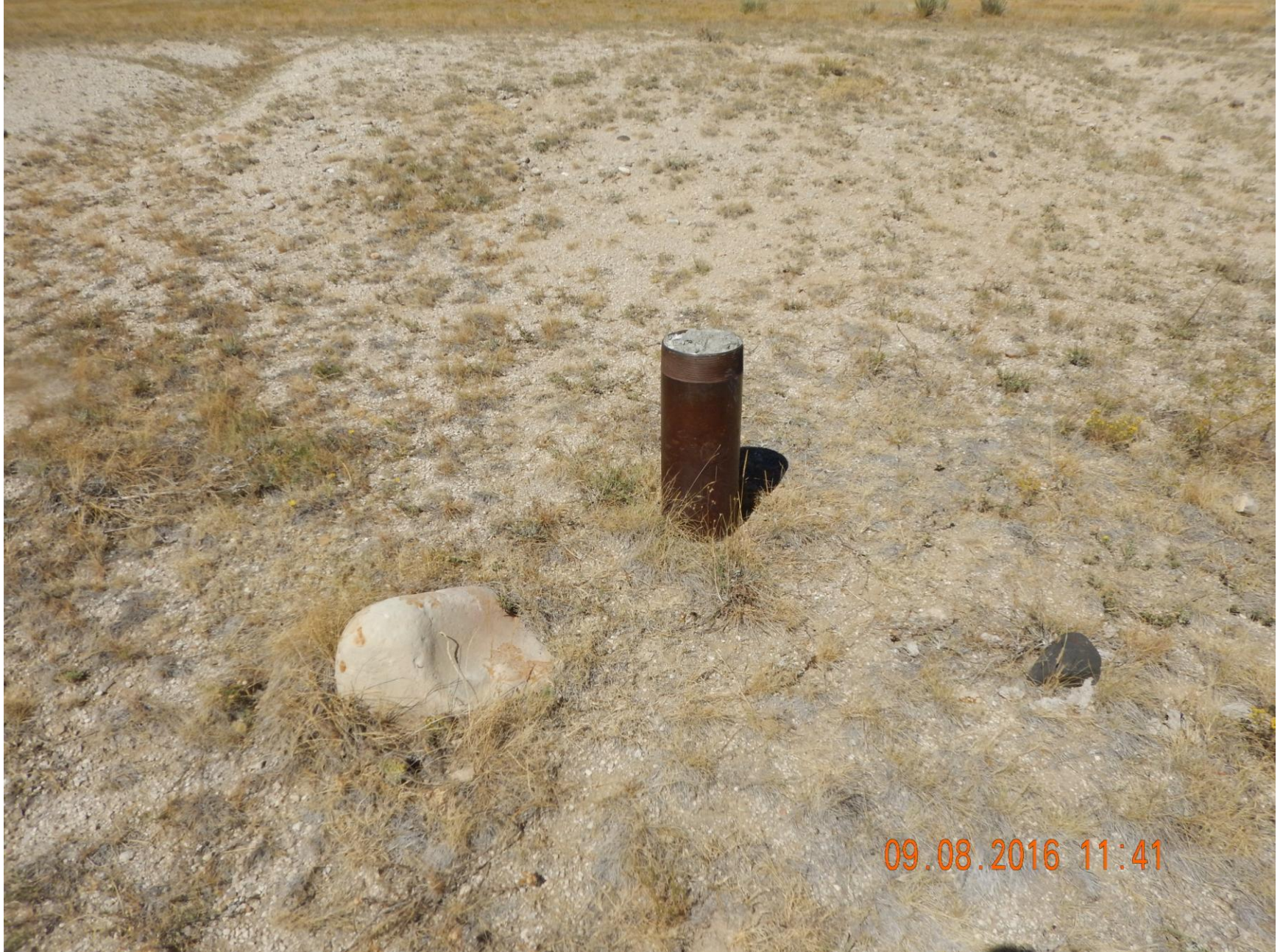
Figure 10: Photo shows casing still remaining on location. Note erosion on slope behind casing.
