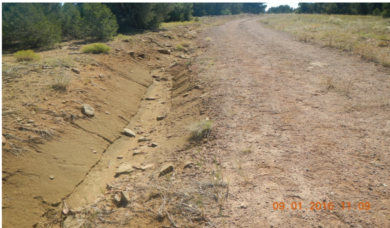
photo 1: Facing southwest along the access road toward the location. There is erosion occurring along the side of the access road.
