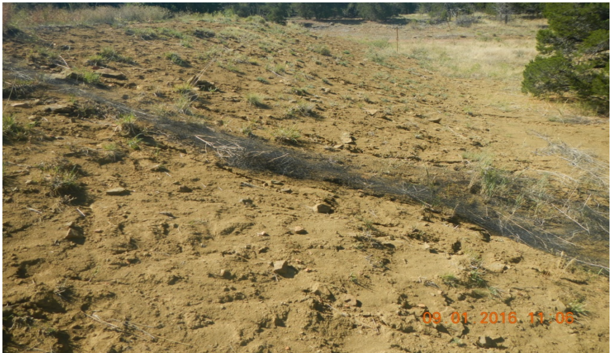
photo 6: There is plastic netting that remains along the fill slope.
