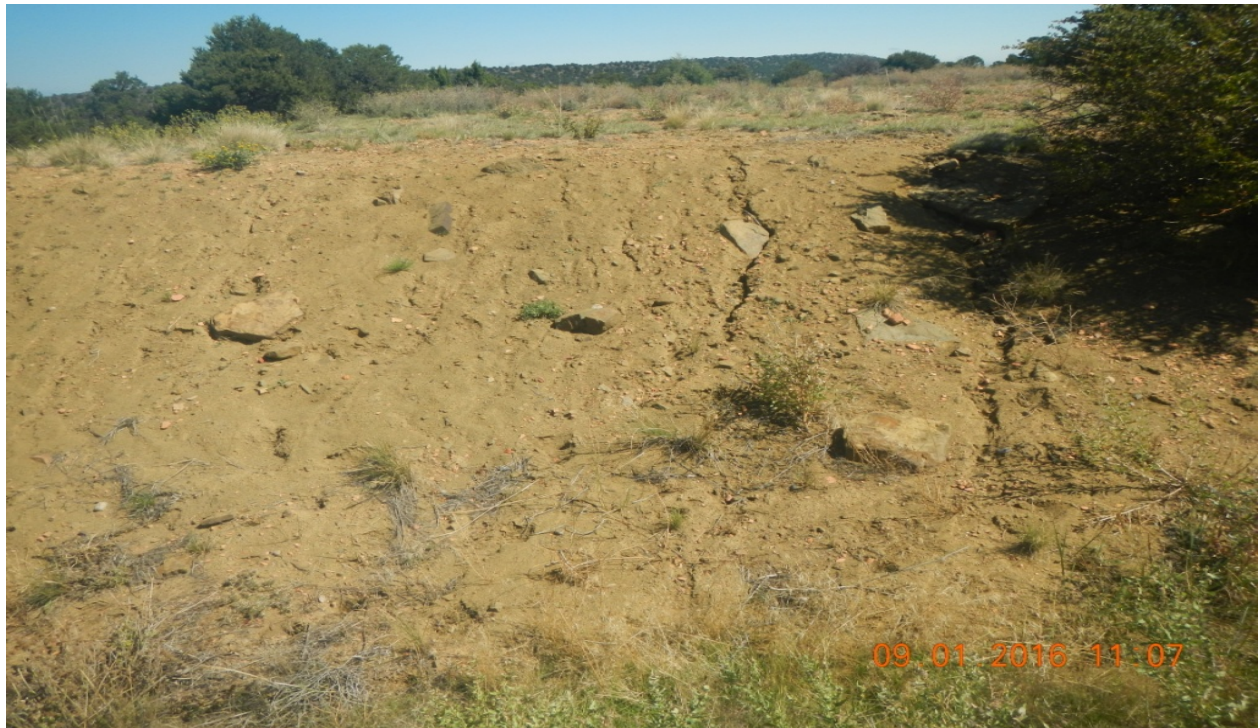
photo 11: There are signs of erosion along west side of the pad.
