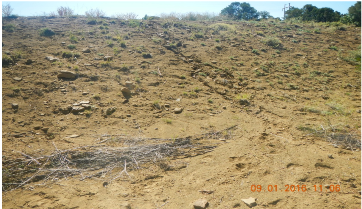
photo 8: The fill slope is not adequately stabilized with vegetation and there are signs of erosion.
