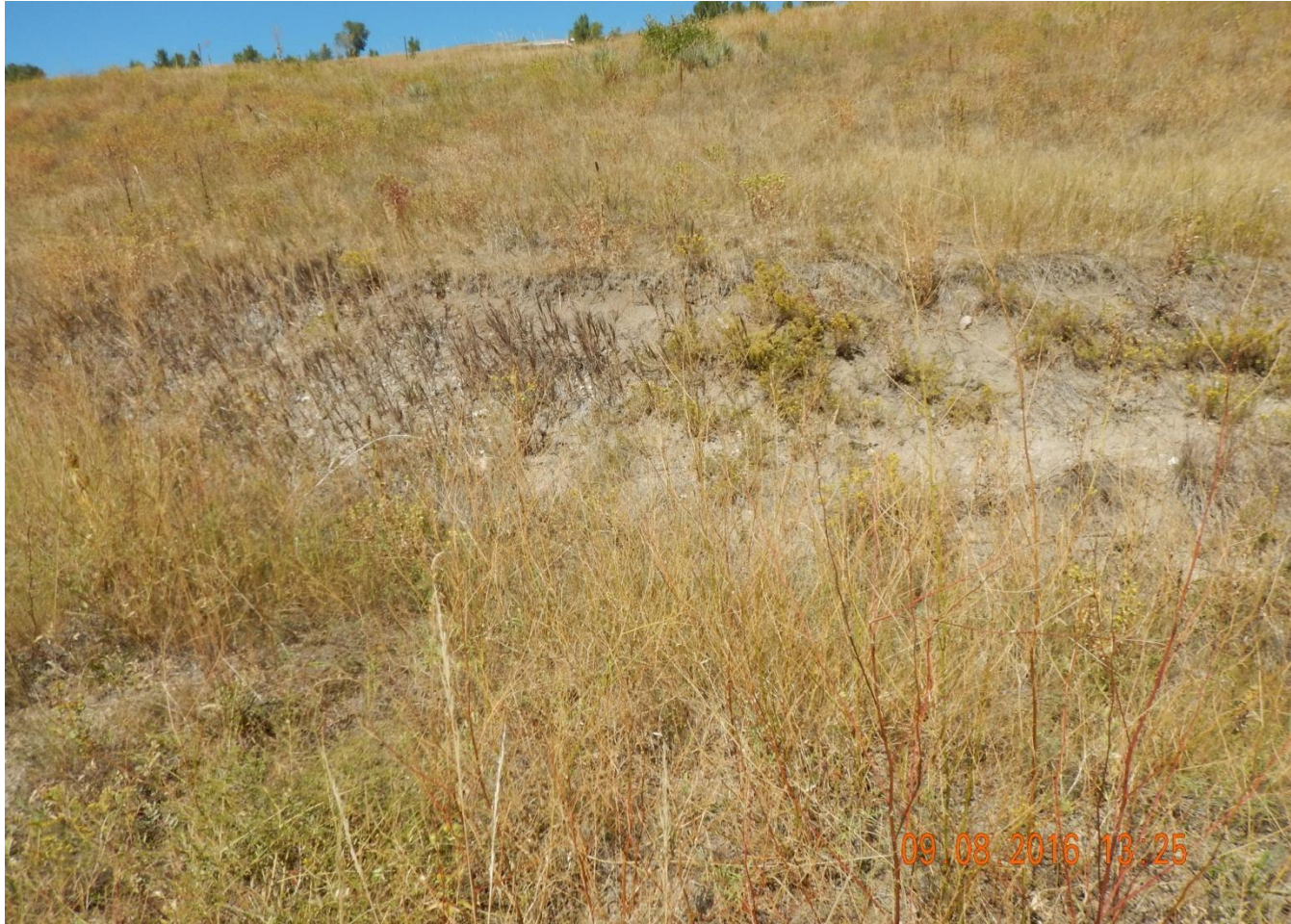
Photo 10. Photo taken along the access road, facing North. Access needs to be re-contoured to the surrounding landscape which will help to prevent erosion which is noticeable along several portions of the access road.
