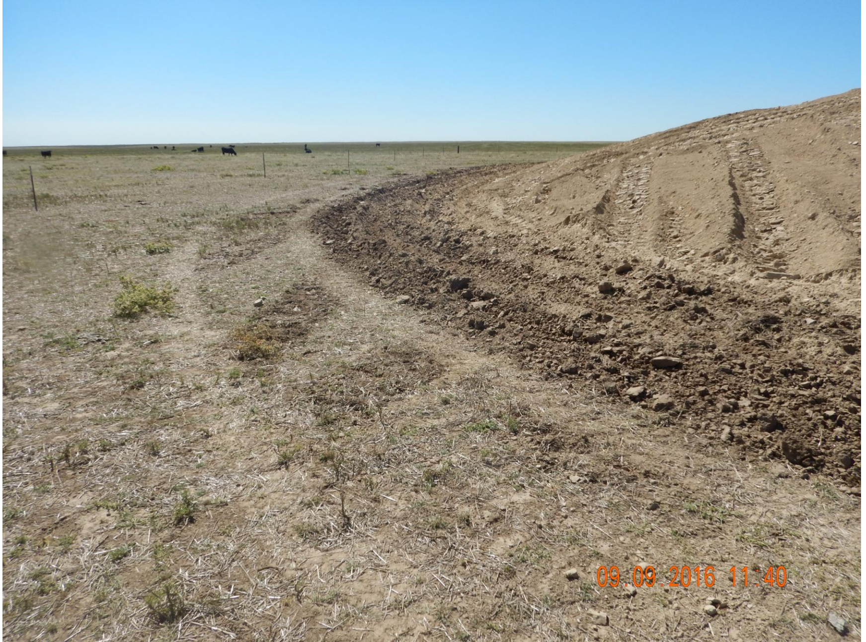
Figure 18: Photo taken from the northeast end of the location, facing south. Photo shows surface roughening used as a stormwater and sediment control BMP on the northeast end of the location. Surface roughening is a BMP that should be used in conjunction with other BMPs. However, with as large as the surface roughening is, and with the topography of this portion of the location being relatively flat, surface roughening alone appears to be sufficient. It is unclear what soil stockpile seen in photo is topsoil, or soil from pits.
