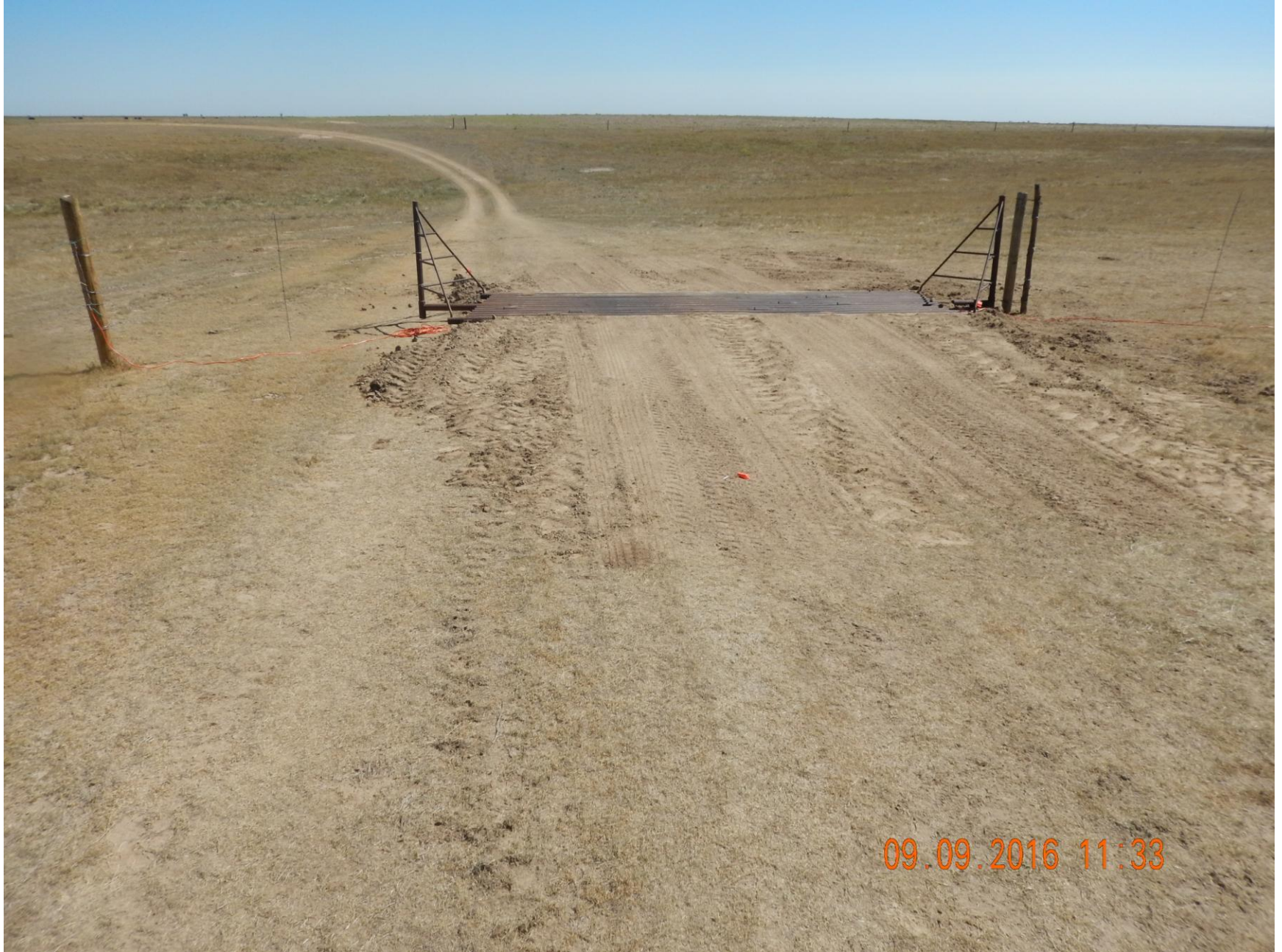
Figure 2: Photo taken from the access road, facing east. Photo shows cattle guard installed on access road.
