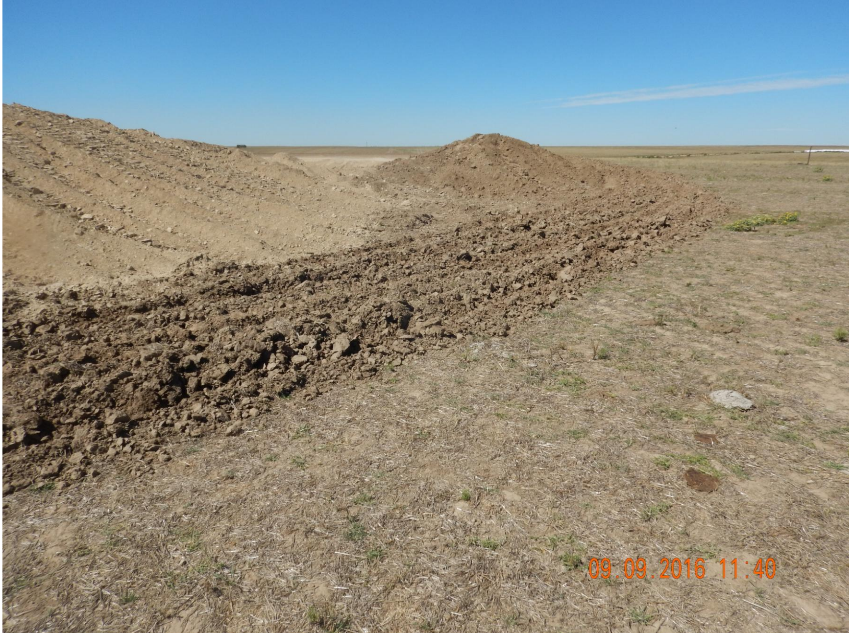
Figure 16: Photo taken from the northeast end of the location, facing west. Photo shows surface roughening used as a stormwater and sediment control BMP on the northeast end of the location. Surface roughening is a BMP that should be used in conjunction with other BMPs. However, with as large as the surface roughening is, and with the topography of this portion of the location being relatively flat, surface roughening alone appears to be sufficient. It is unclear what soil stockpile seen in photo is topsoil, or soil from pits.
