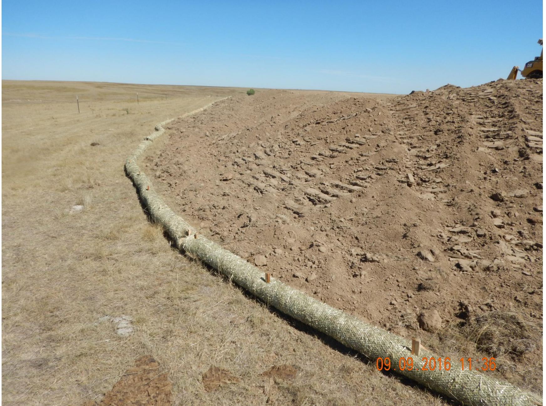
Figure 9: Photo taken from the southwest corner of the location, facing north. Photo shows straw wattles at base of the western end of the location. Wattles improperly installed; need to be entrenched in order to be in proper functioning condition. Unclear if soil seen on perimeter is topsoil.
