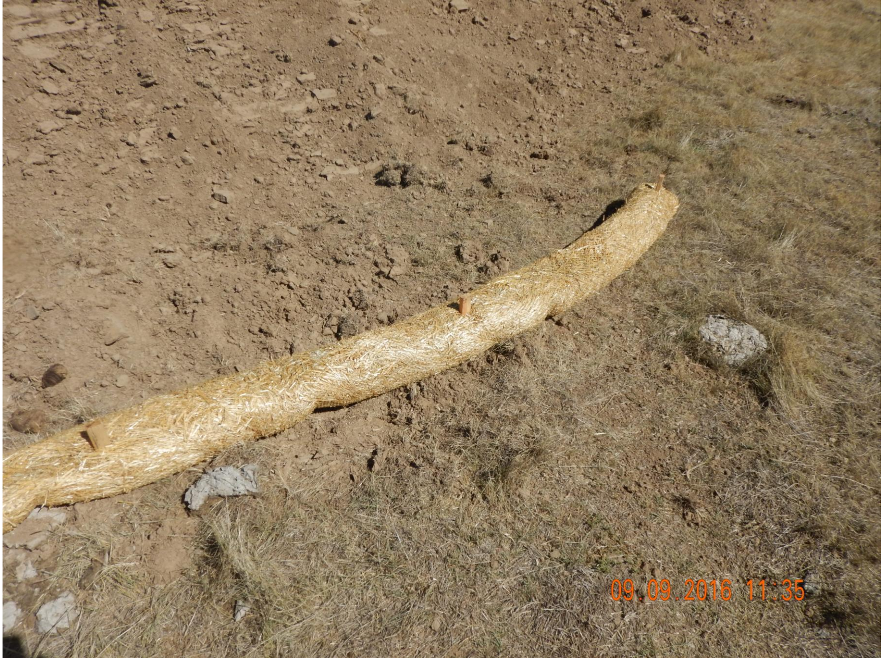
Figure 7: Photo taken from the southwest corner of the location. Photo shows straw wattle used as a stormwater and sediment control BMP improperly installed. Wattles need to be entrenched in order to be in proper functioning condition.
