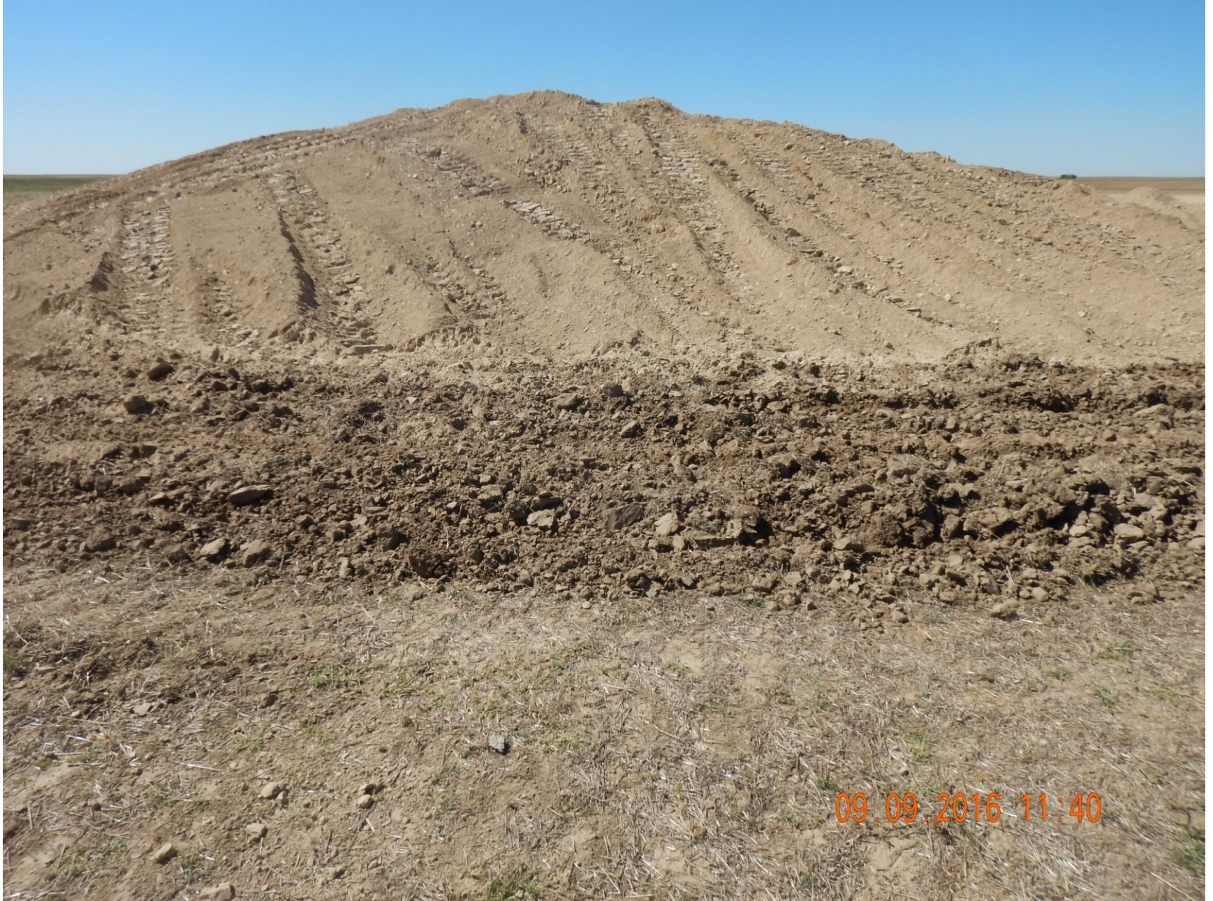
Figure 17: Photo taken from the northeast end of the location, facing southwest. Photo shows surface roughening used as a stormwater and sediment control BMP on the northeast end of the location. Surface roughening is a BMP that should be used in conjunction with other BMPs. However, with as large as the surface roughening is, and with the topography of this portion of the location being relatively flat, surface roughening alone appears to be sufficient. It is unclear what soil stockpile seen in photo is topsoil, or soil from pits.
