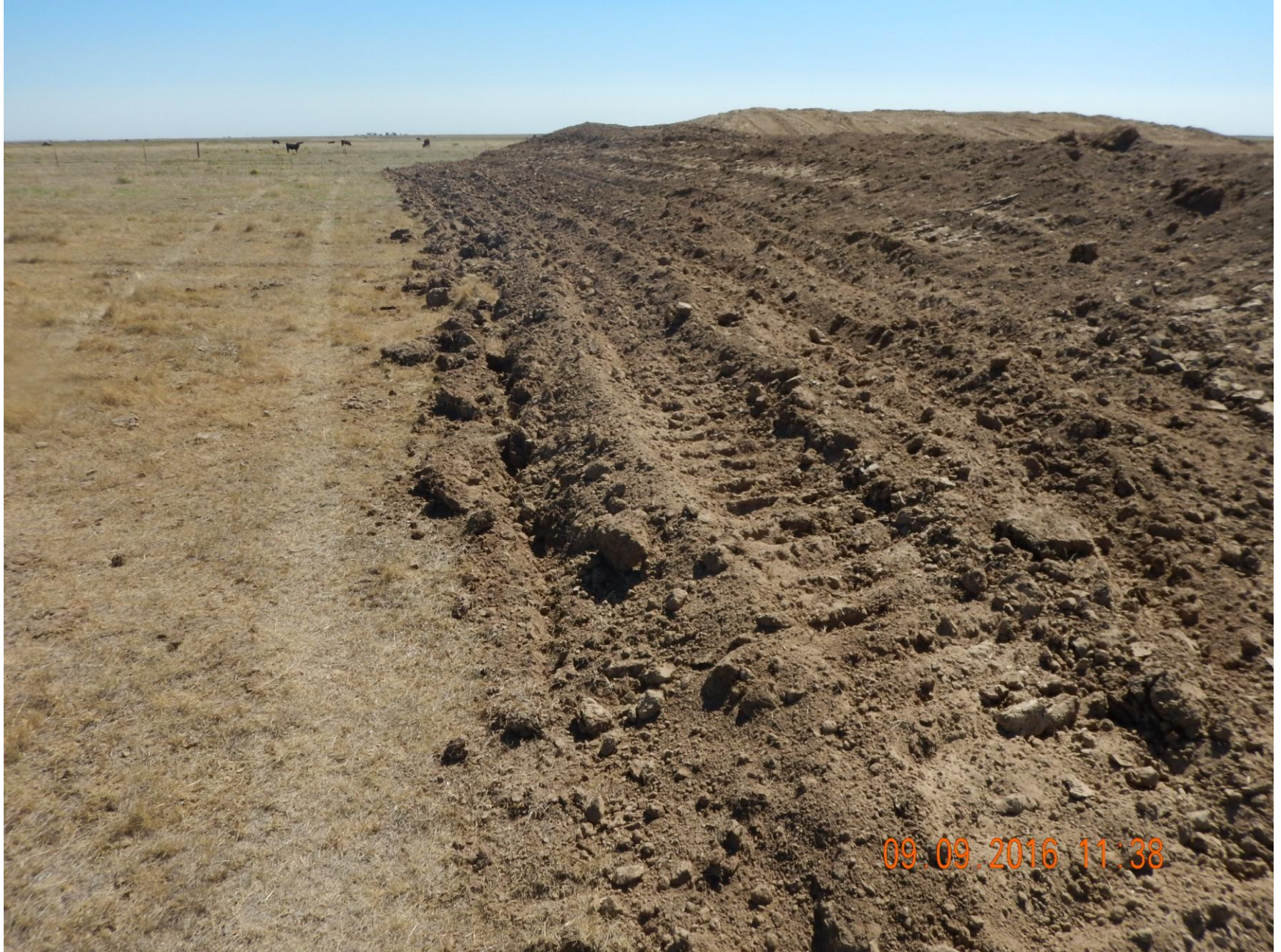
Figure 14: Photo taken from the north end of the location, facing east. Photo shows surface roughening used as a stormwater and sediment control BMP on the northeast end of the location. Surface roughening is a BMP that should be used in conjunction with other BMPs. However, with as large as the surface roughening is, and with the topography of this portion of the location being relatively flat, surface roughening alone appears to be sufficient.
