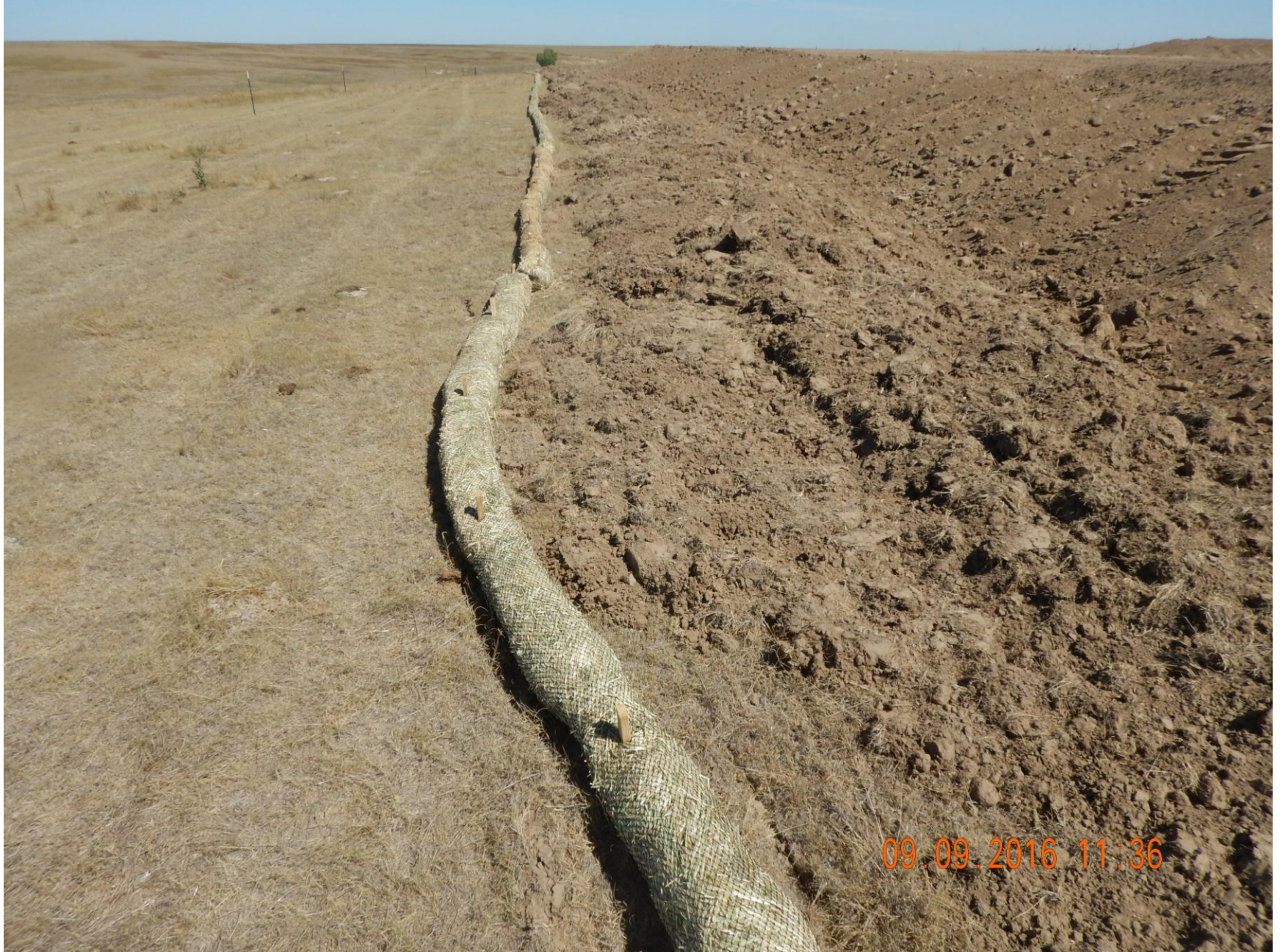
Figure 10: Photo taken from the west end of the location, facing west. Wattles improperly installed; need to be entrenched in order to be in proper functioning condition. It is unclear if soil seen on perimeter is topsoil.
