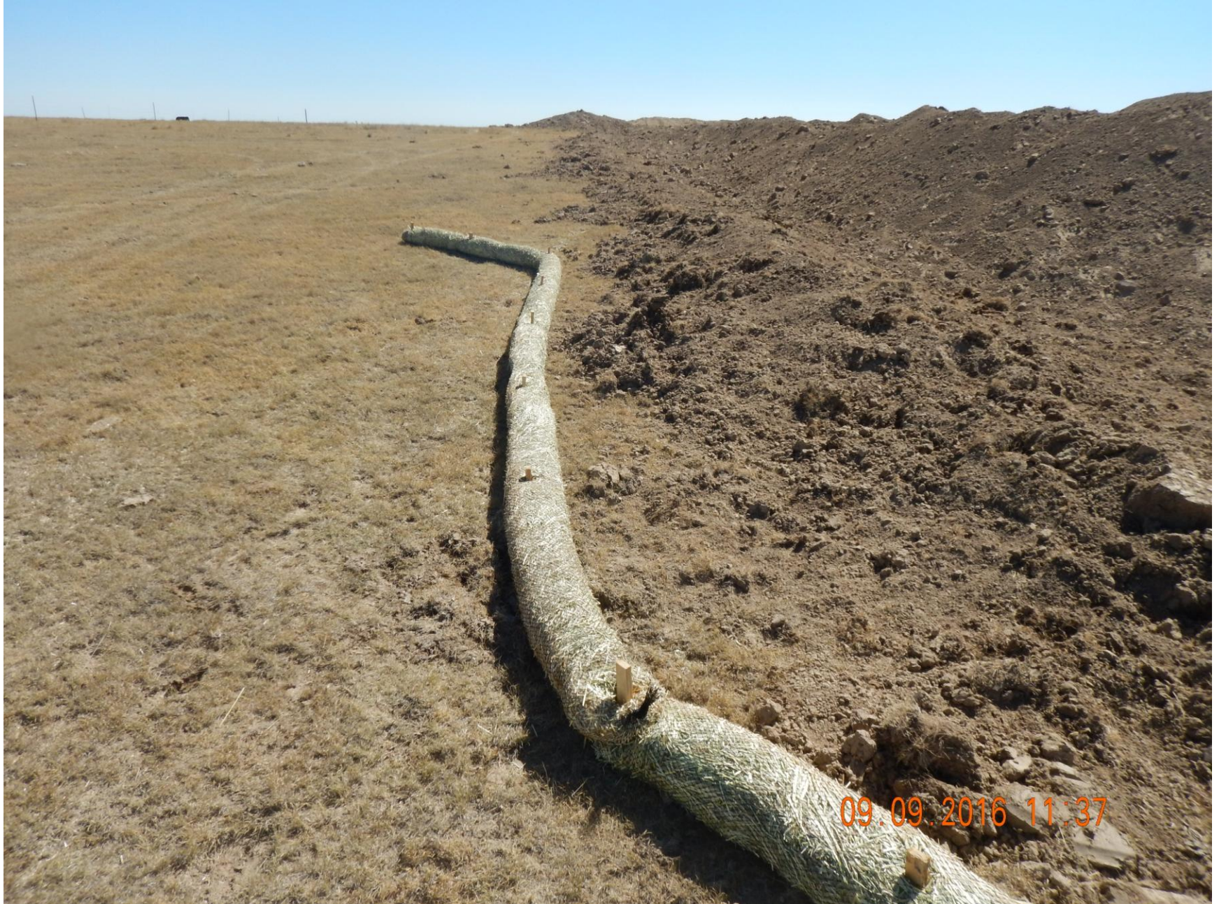
Figure 12: Photo taken from the northwest corner of the location, facing east. Photo shows straw wattles at base of the western end of the location. Wattles improperly installed; need to be entrenched in order to be in proper functioning condition. Unclear if soil seen on perimeter is topsoil.
