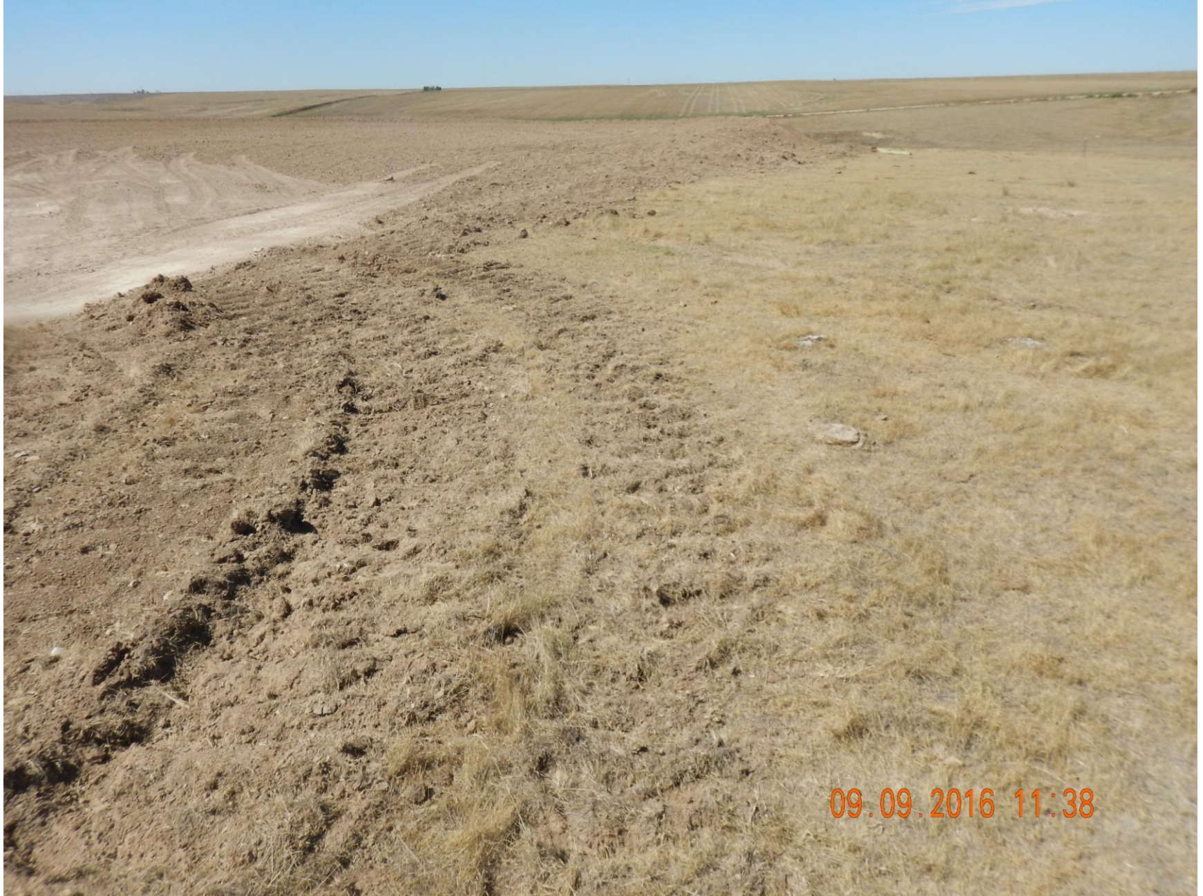
Figure 15: Photo taken from the north end of the location, facing west. Photo shows straw wattle “j-hook” as only stormwater and sediment control BMP in place on the northwest end of the location. Note: “J-hook” seen here does not appear to be large enough to capture stormwater from the north end of the location. Advise increasing size of “j-hook”
