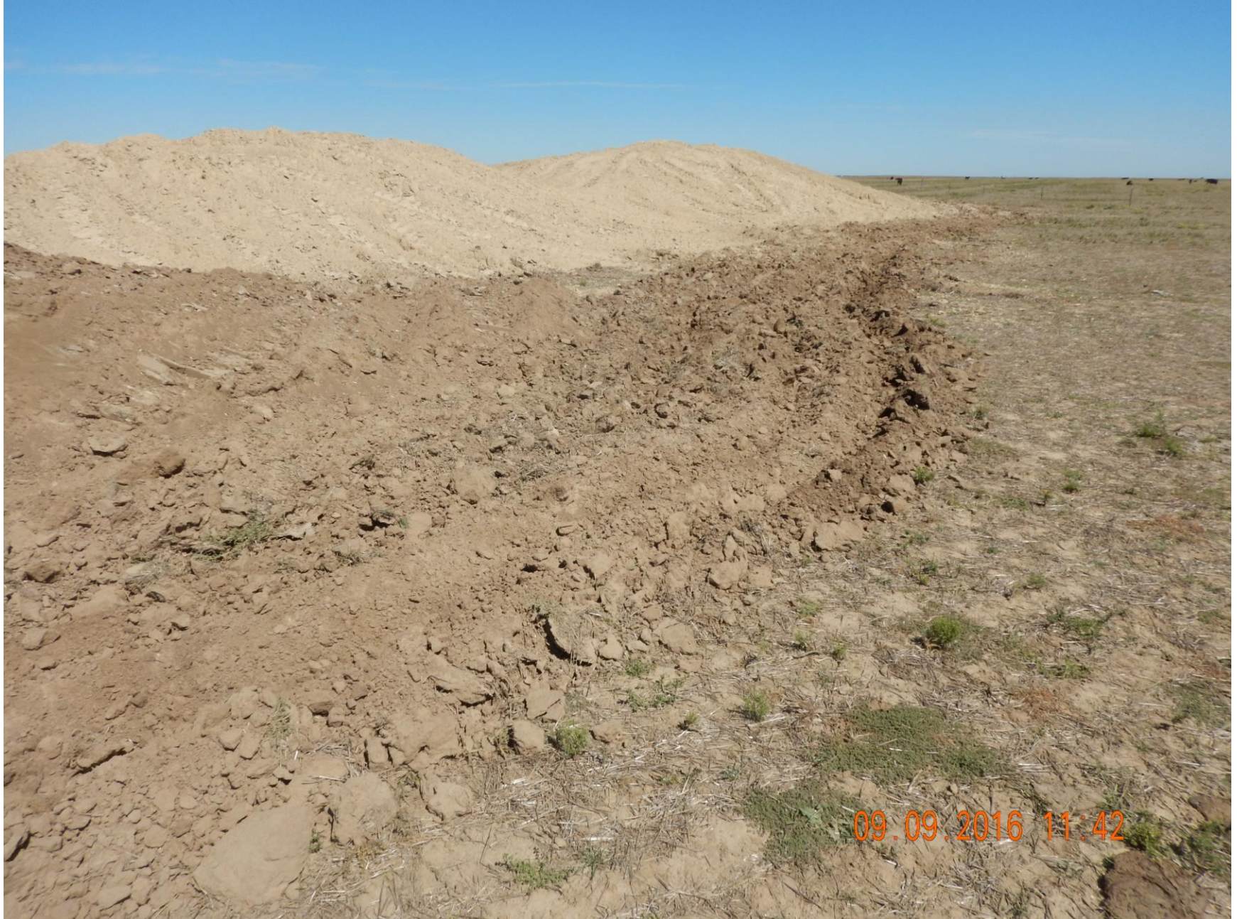
Figure 19: Photo taken from the southeast end of the location, facing north. Photo shows surface roughening used as a stormwater and sediment control BMP on the northeast end of the location. Surface roughening is a BMP that should be used in conjunction with other BMPs. However, with as large as the surface roughening is, and with the topography of this portion of the location being relatively flat, surface roughening alone appears to be sufficient. It is unclear what soil stockpile seen in photo is topsoil, or soil from pits.
