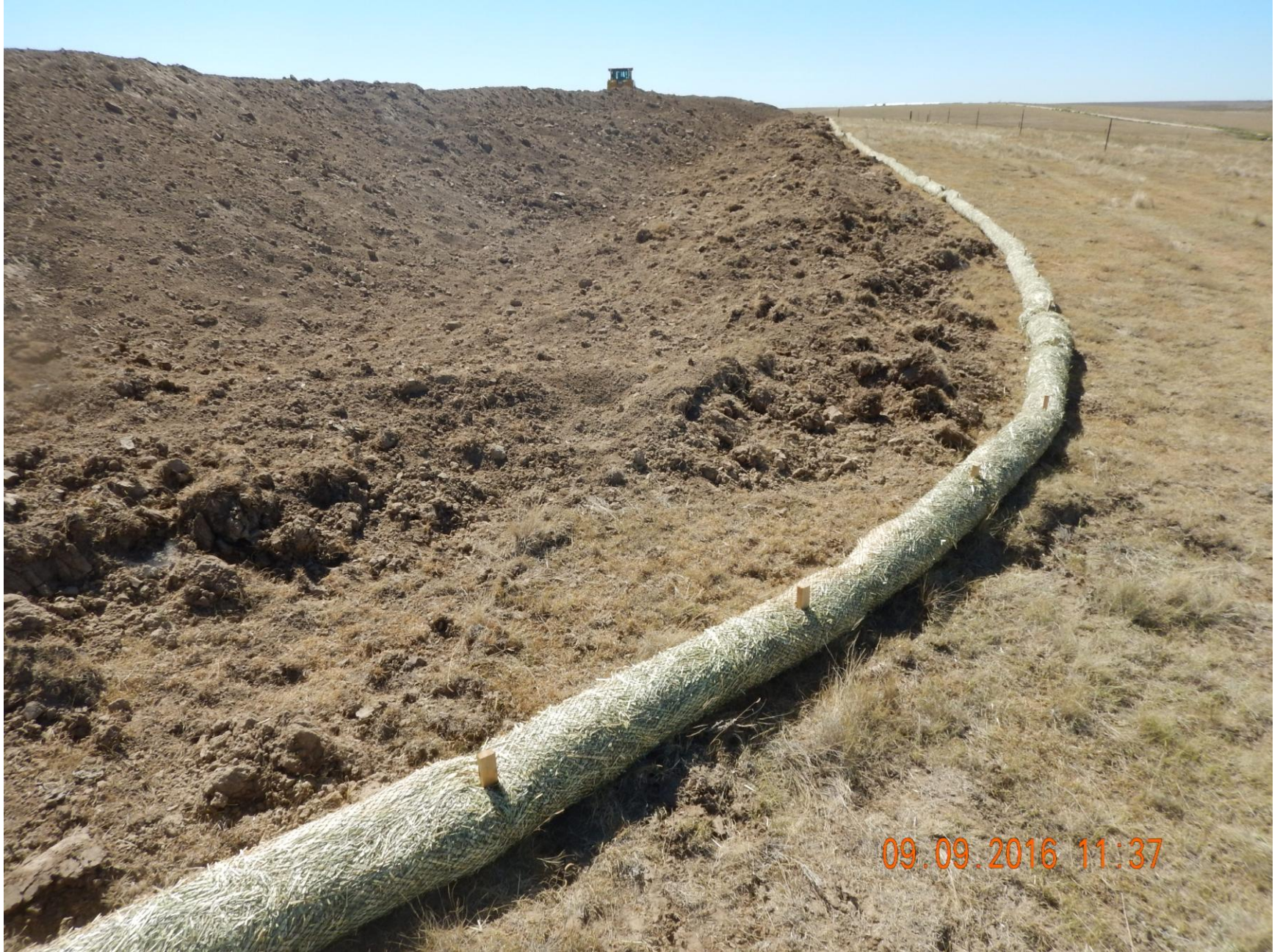
Figure 11: Photo taken from the northwest corner of the location, facing north. Photo shows straw wattles at base of the western end of the location. Wattles improperly installed; need to be entrenched in order to be in proper functioning condition. Unclear if soil seen on perimeter is topsoil.
