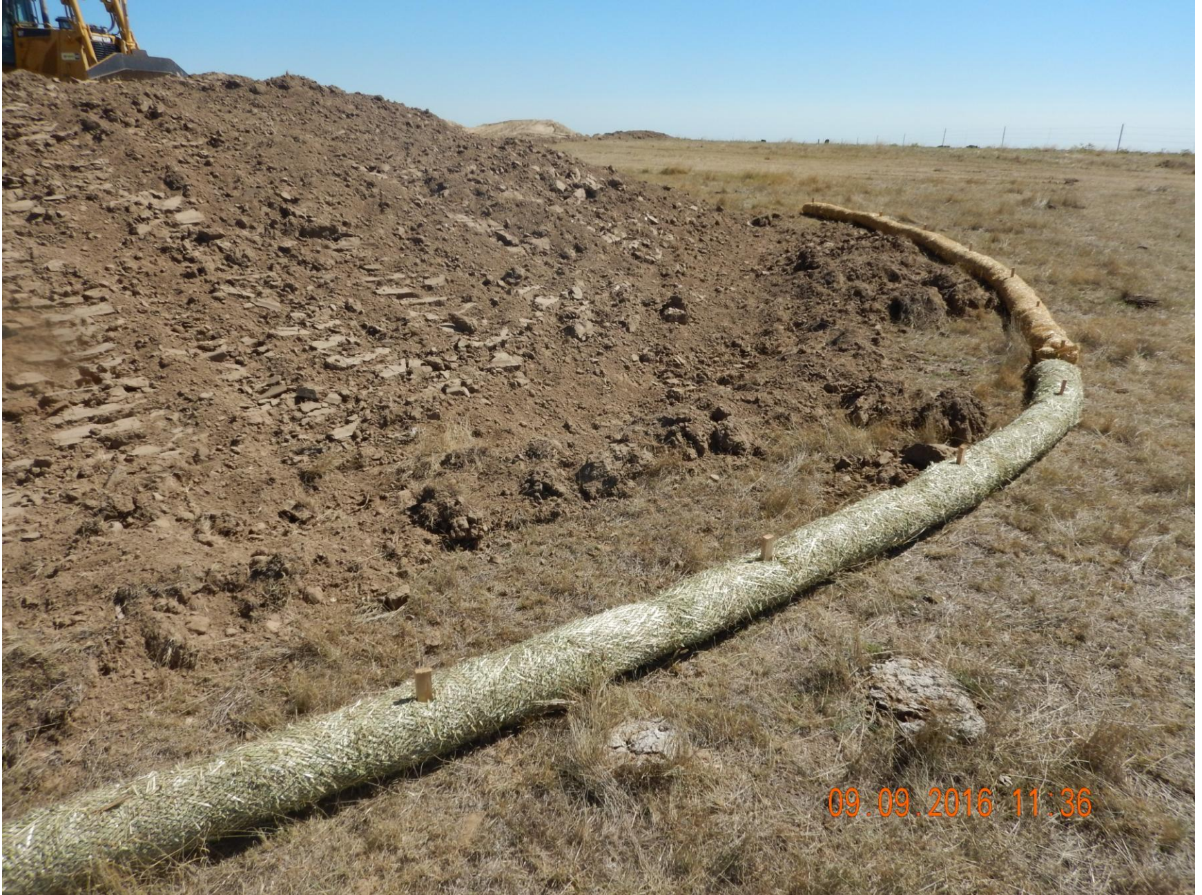
Figure 8: Photo taken from the southwest corner of the location, facing east. Photo shows straw wattles at base of the western end of the location. Wattles improperly installed; need to be entrenched in order to be in proper functioning condition.
