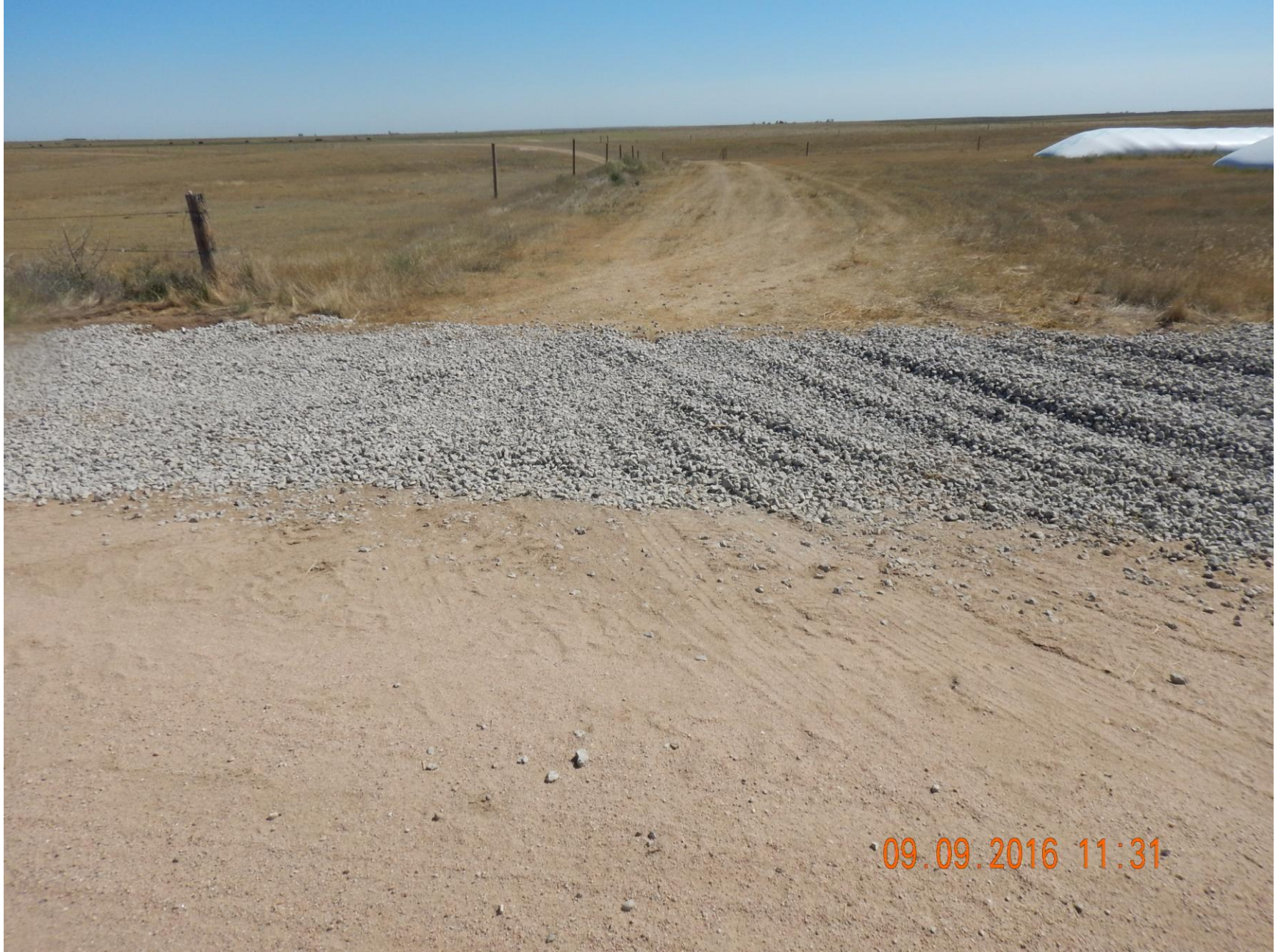
Figure 1: Photo taken from CR 46, facing east. Photo shows vehicle tracking BMP installed at access road entrance.
