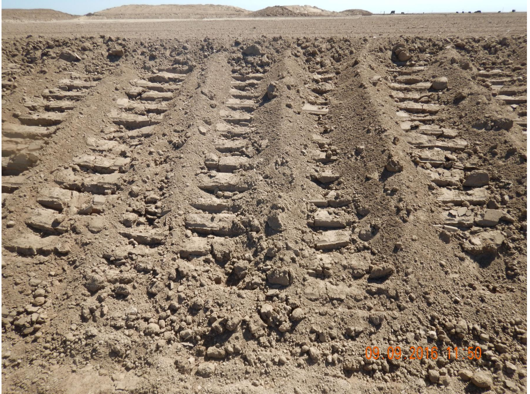
Figure 31: Photo taken from the west end of the location, facing east. Photo shows slopes have been improperly tracked and remain largely unstabilized.
