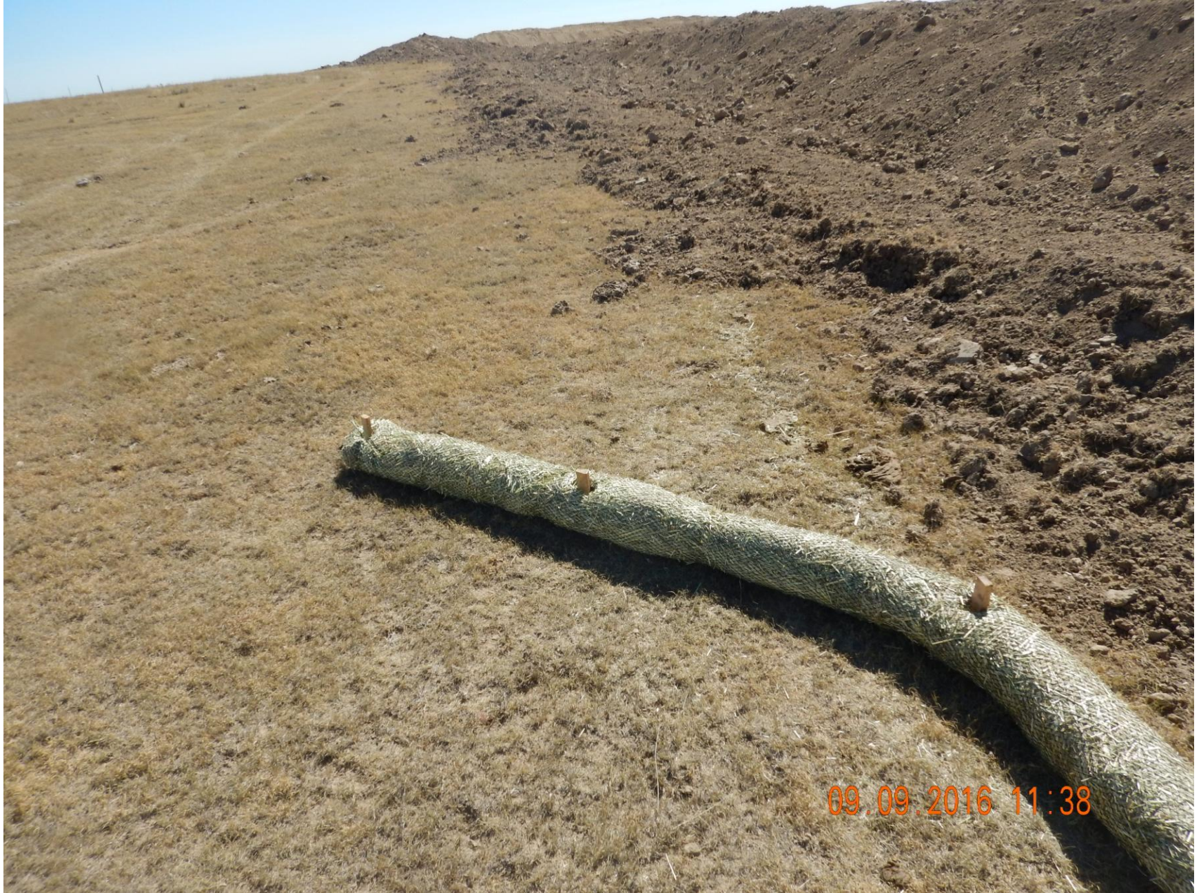
Figure 13: Photo taken from the northwest corner of the location, facing east. Photo shows wattles improperly installed; need to be entrenched in order to be in proper functioning condition. Note: “J-hook” seen here does not appear to be large enough to capture stormwater from the north end of the location. Advise increasing size of “j-hook”
