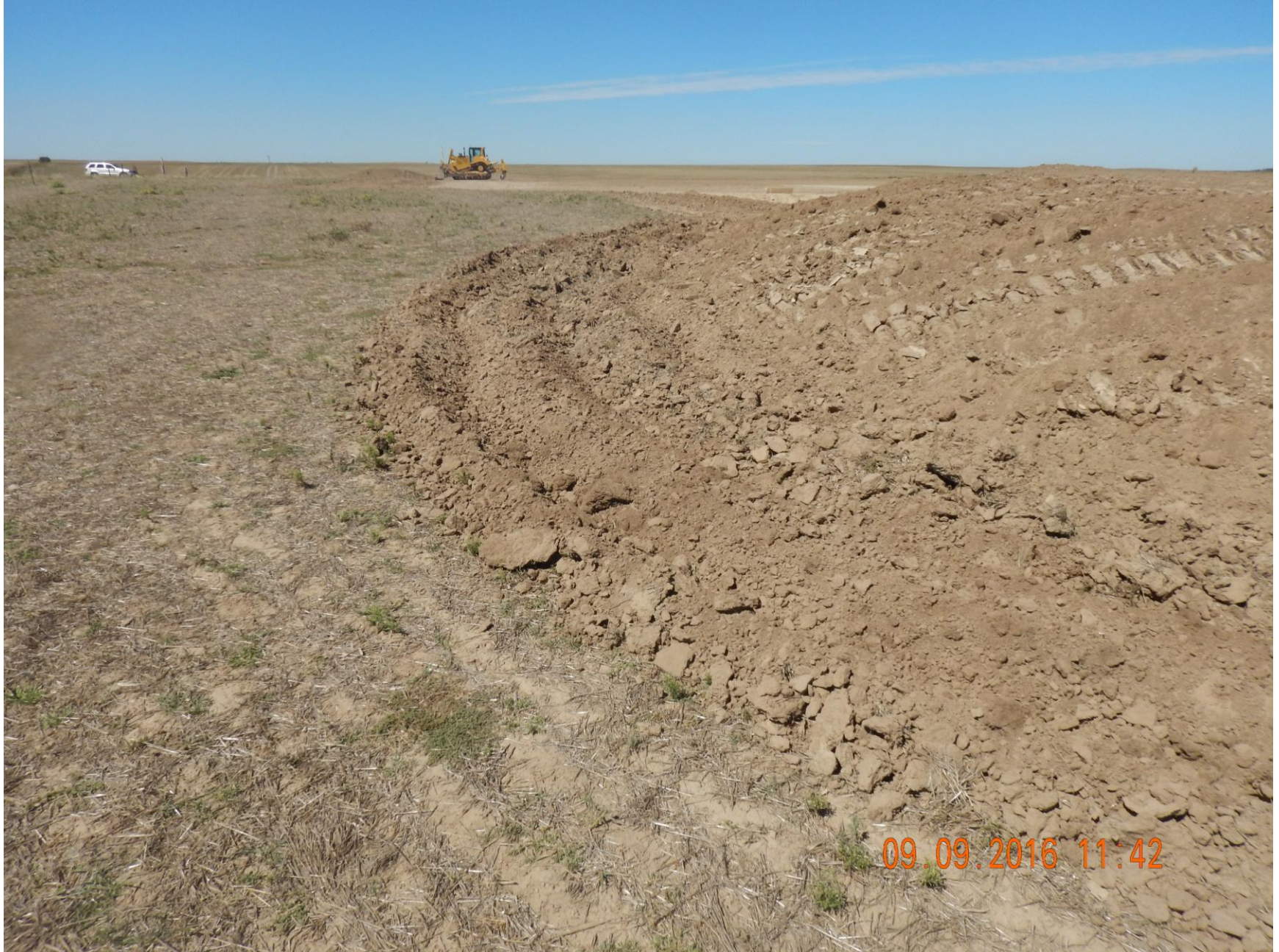
Figure 20: Photo taken from the southeast end of the location, facing west. Photo shows surface roughening used as a stormwater and sediment control BMP on the northeast end of the location. Surface roughening is a BMP that should be used in conjunction with other BMPs. However, with as large as the surface roughening is, and with the topography of this portion of the location being relatively flat, surface roughening alone appears to be sufficient. It is unclear what soil stockpile seen in photo is topsoil, or soil from pits.
