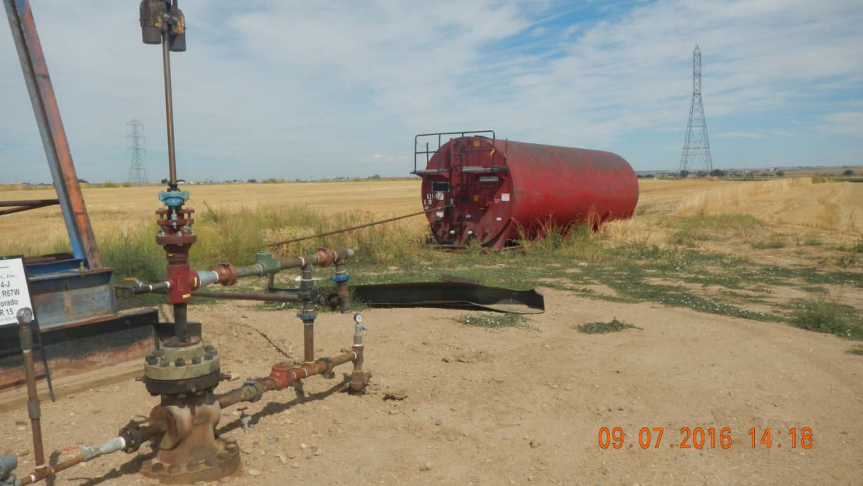
API # 123-12831, WEEDS AND TANK WITH NO BERM.
