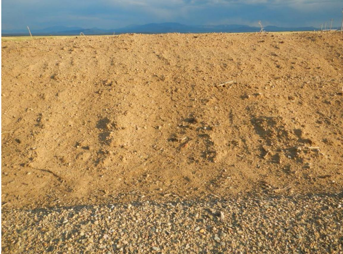
Photo#4: West slope of East N>S Berm is Bare of Vegetation.
