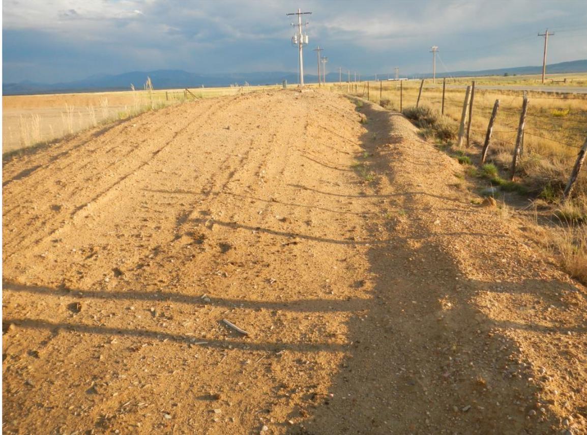
Photo#6: West Slope of West N>S Berm is bare of Vegetation.
