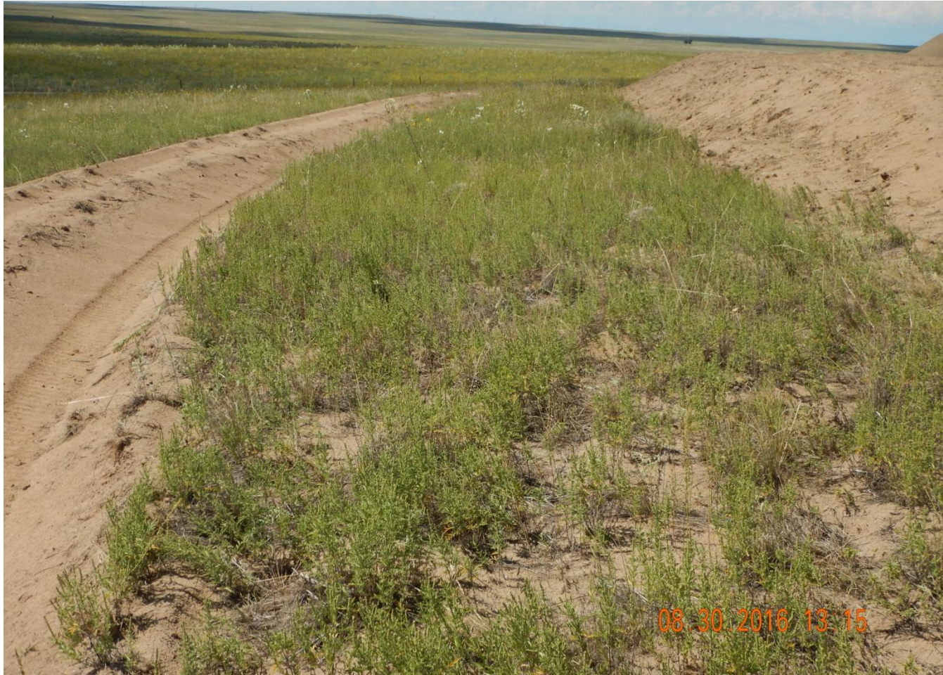
Photo 5. Photo taken from southeast location, facing West. BMP installed to the left and topsoil stockpile salvage pile to the right.
