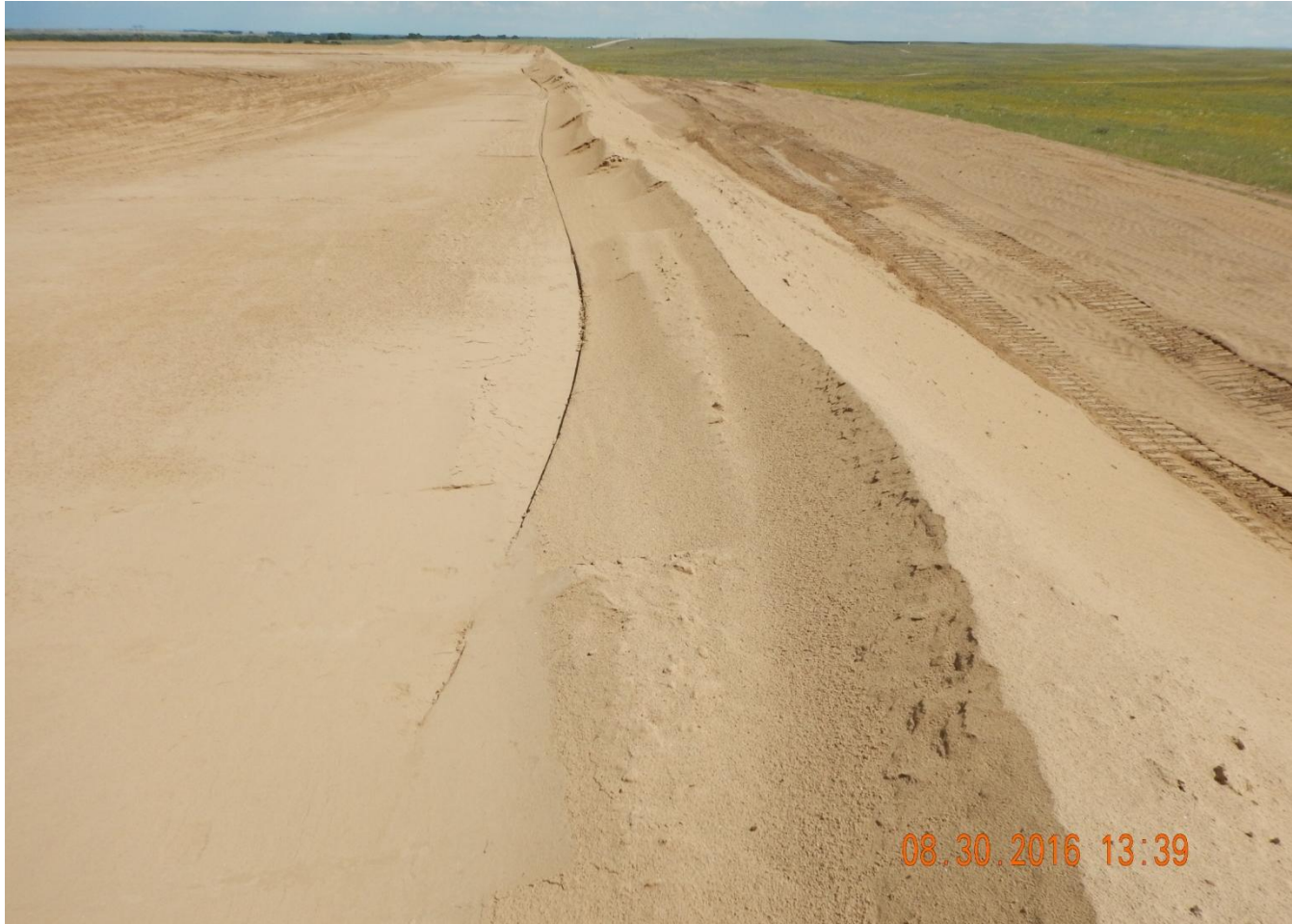
Photo 10. Photo taken from southern well pad location, facing East. BMP installed along outer perimeter of well pad.
