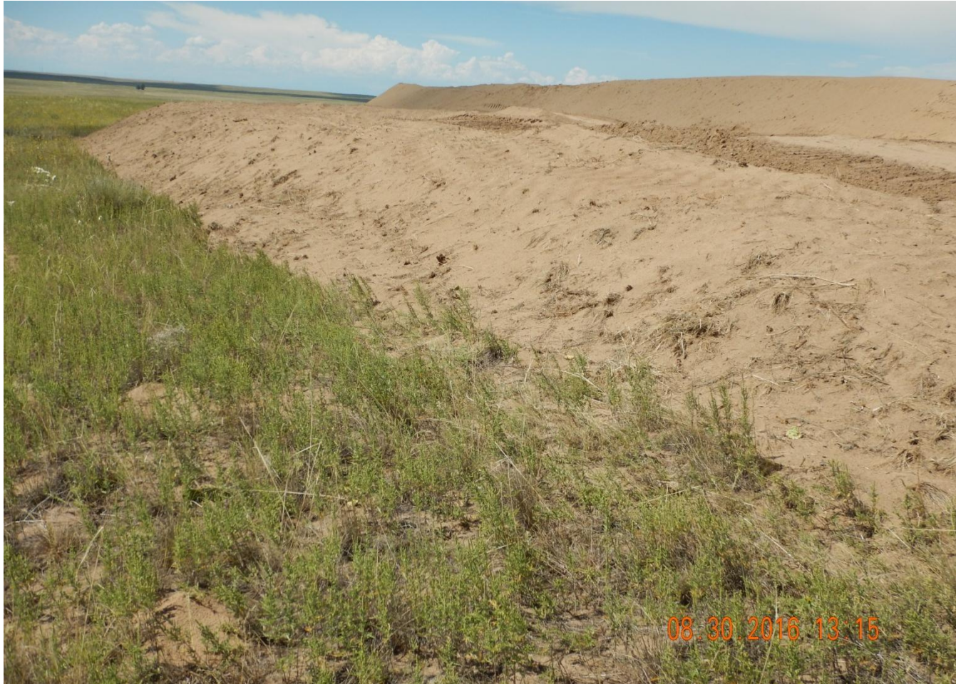
Photo 6. Photo taken from southern location, facing North towards topsoil stockpile. Need to stabilize topsoil stockpile and all fill slopes.
