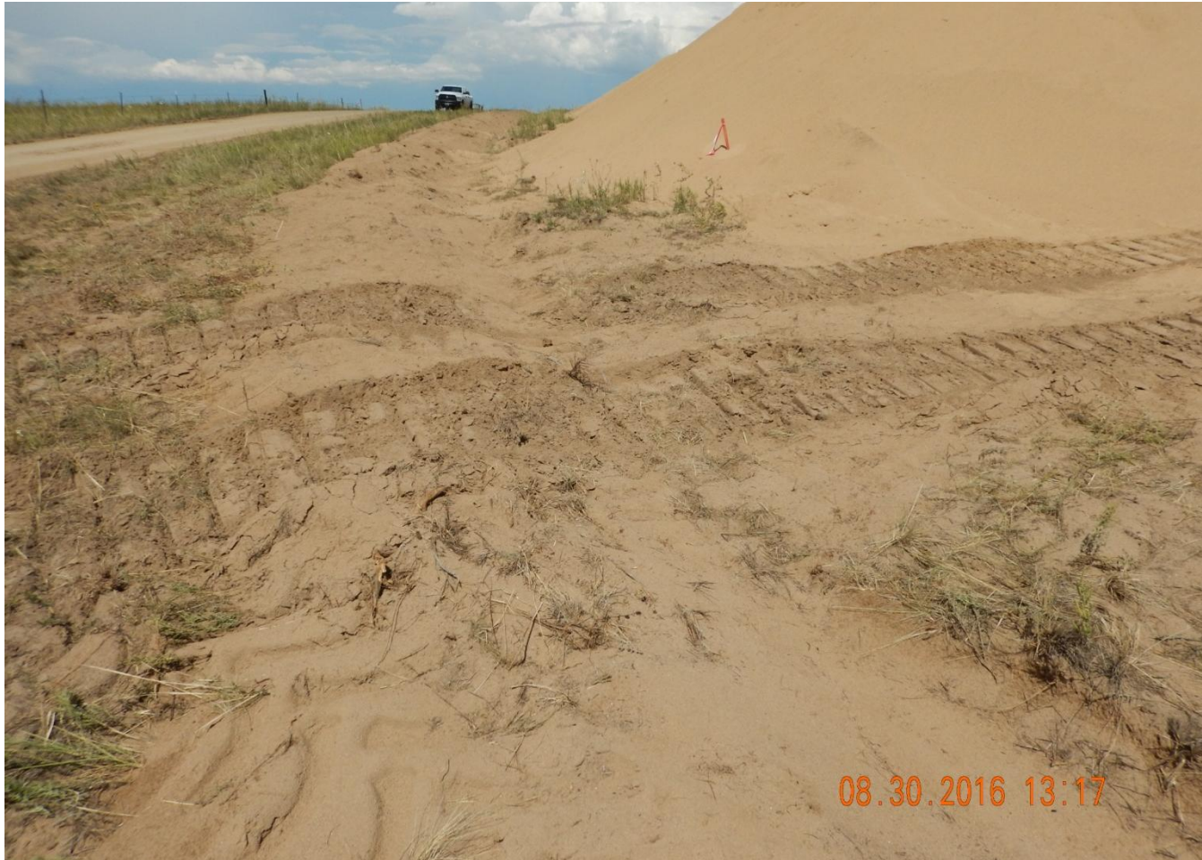
Photo 7. Photo taken from southwest location, facing North. Need to maintain BMPs at all times and keep vehicle traffic off BMPs. Need to stabilize all fill slopes.
