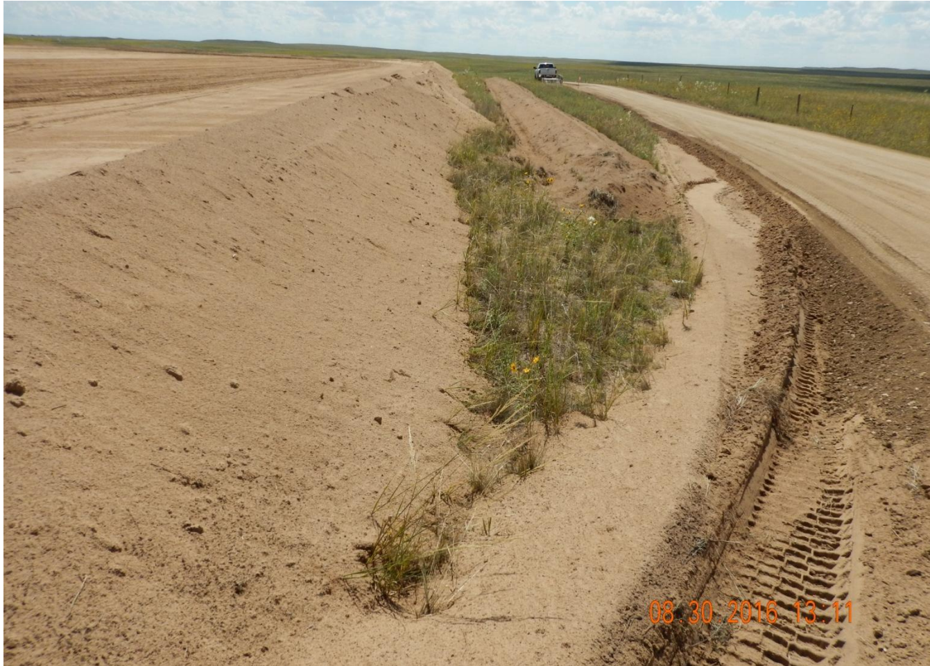
Photo 1. Photo taken from northwestern location, facing South. Need to stabilize all fill slopes.
