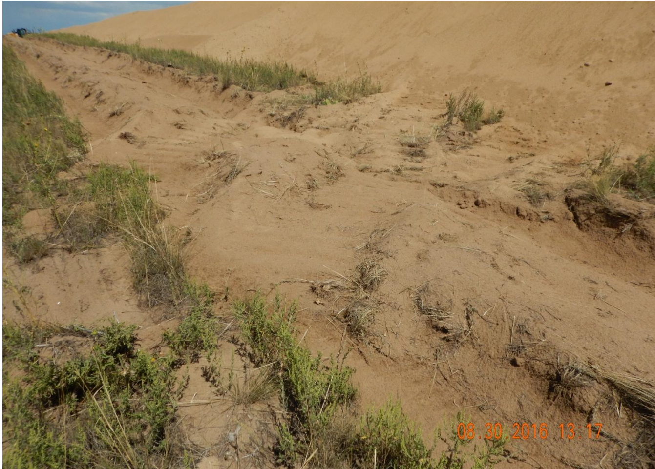
Photo 8. Photo taken from southwest location, facing East. Need to maintain BMPs at all times and keep vehicle traffic off BMPs. Need to stabilize all fill slopes.
