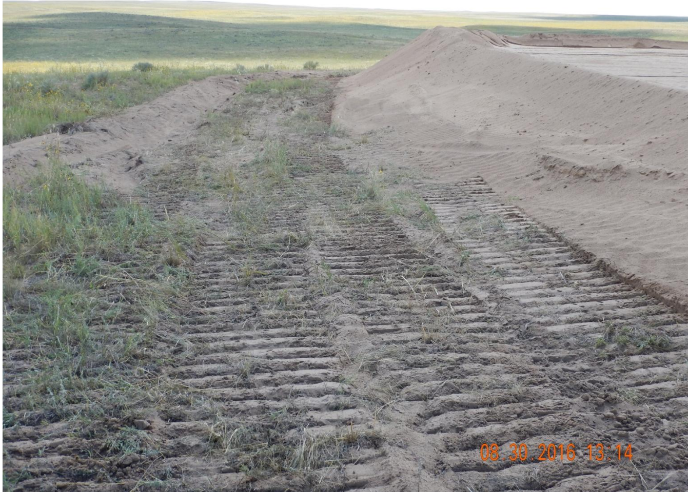
Photo 3. Photo taken from southeastern location, facing South. Need to stabilize all fill slopes.
