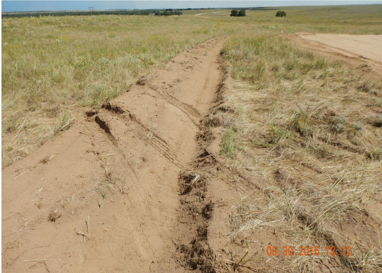
Photo 2. Photo taken from northern location, facing East. Need to maintain BMPs at all times and keep vehicle traffic off BMPs.
