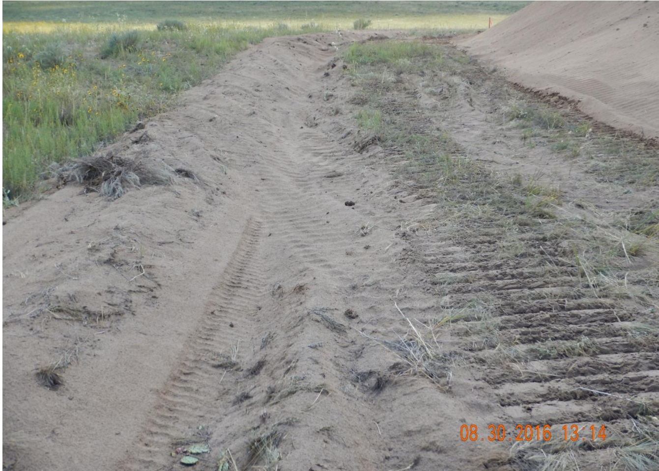
Photo 4. Photo taken from southeastern location, facing South. Need to maintain BMPs at all times and keep vehicle traffic off BMPs.
